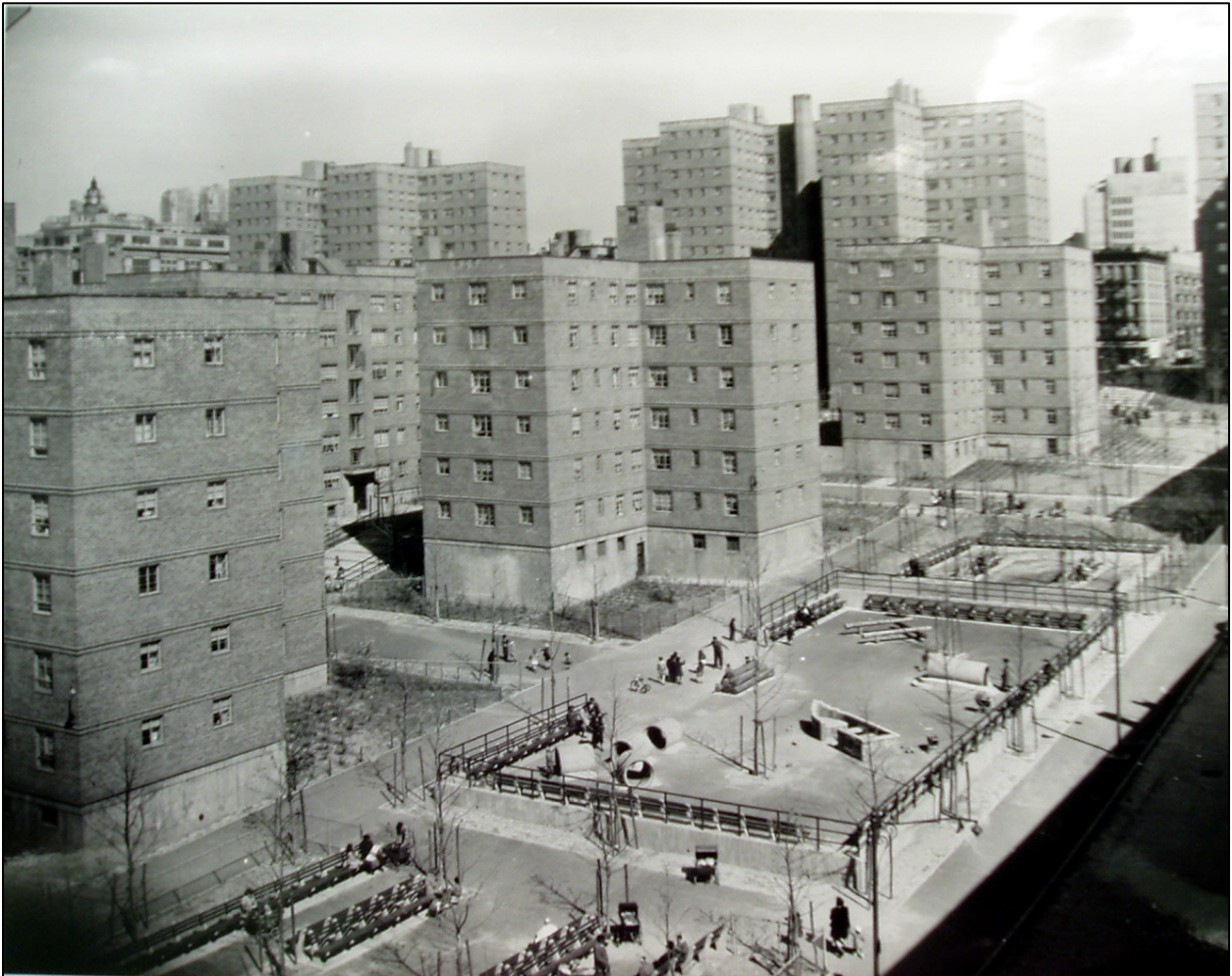
Amsterdam Houses (ca. 1947) looking east from West 61 st St. and West End Ave. New York Historical Society
