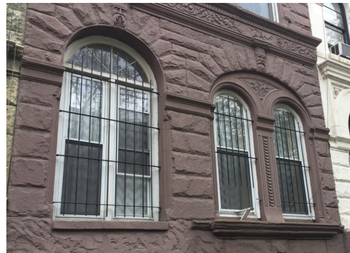
2 nd floor Windows
