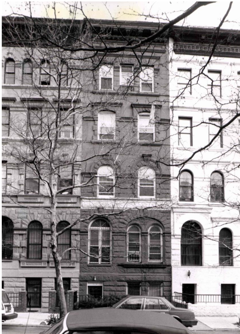
Designation Photo taken at the time the violation was issued
