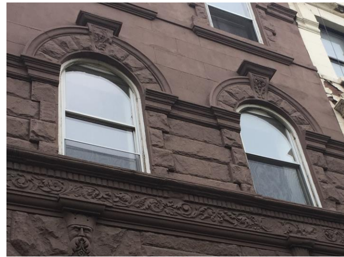
3 rd floor Windows
