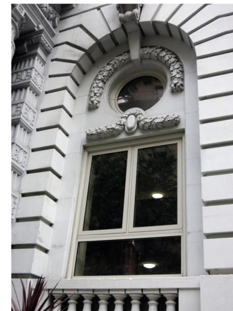
INSTALLED WINDOW TYPE B2 WITH GLASS PANEL
