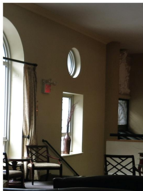
INSTALLED WINDOW TYPE B FROM INTERIOR
