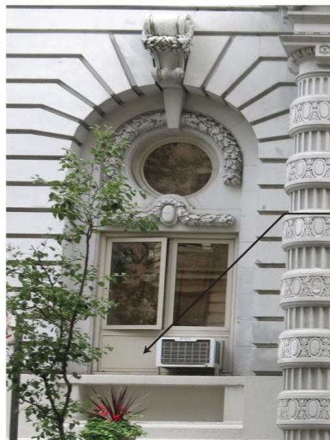
INSTALLED WINDOW TYPE B1 WITH AIR CONDITIONER UNIT
