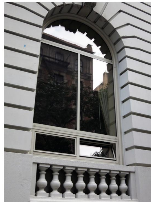
INSTALLED WINDOW TYPE A EXTERIOR
