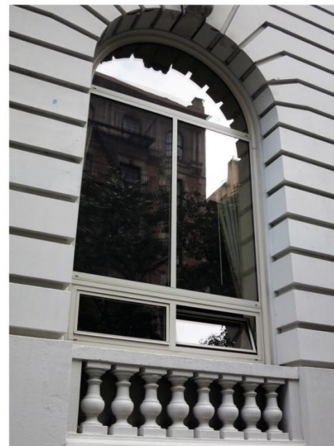
INSTALLED WINDOW TYPE A EXTERIOR
