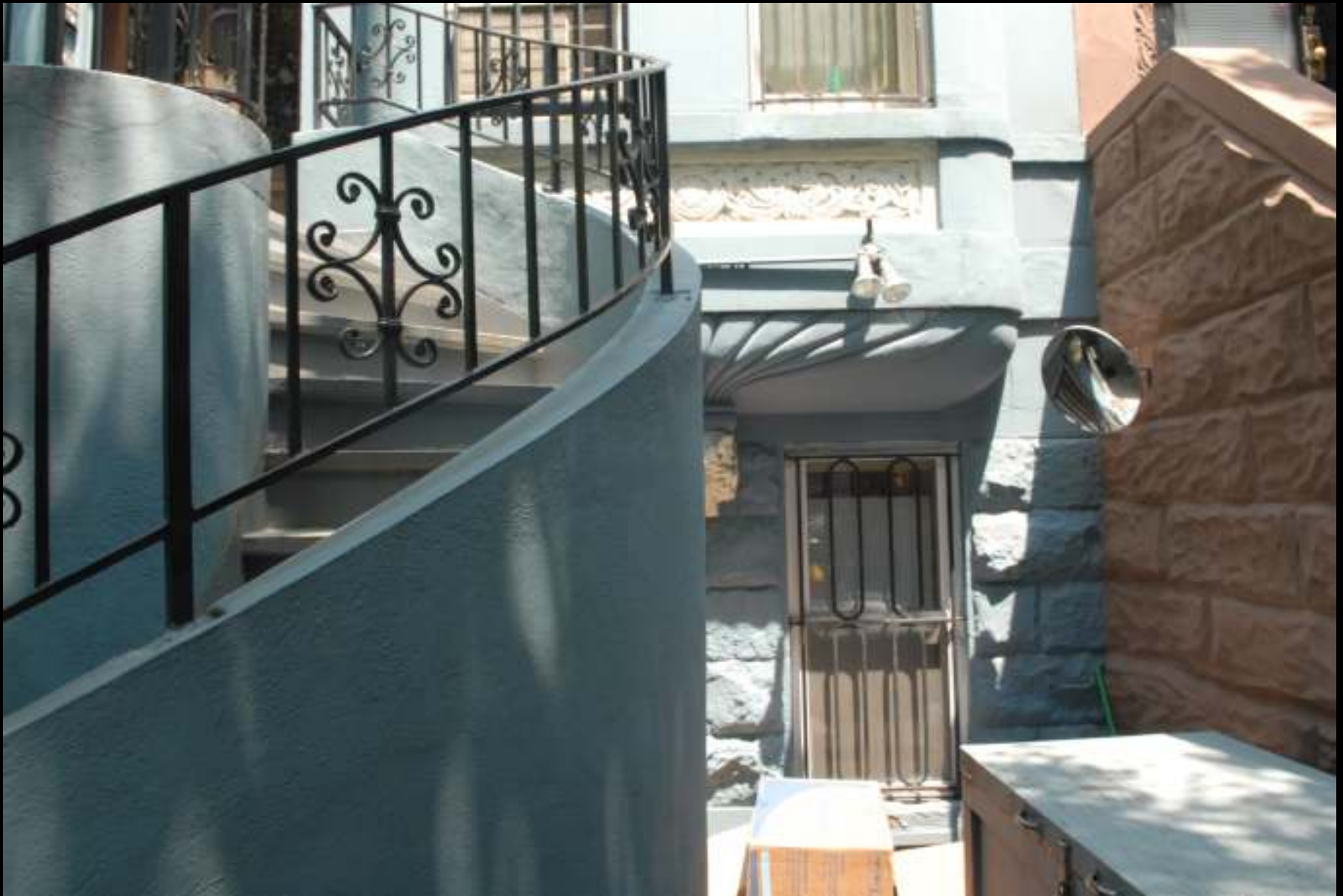
Area Way Garbage Area tucked beside altered stoop
