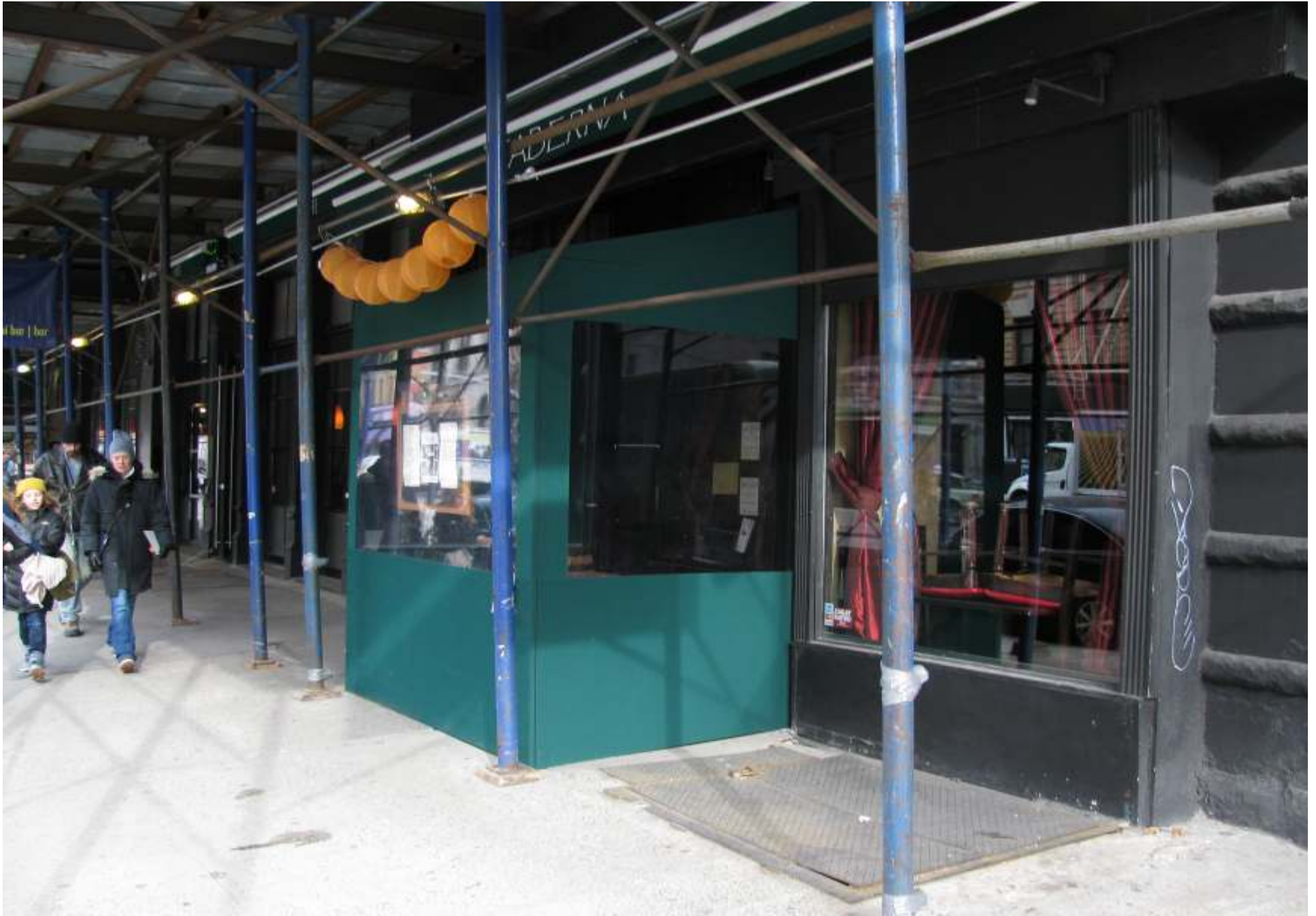
Restaurants right neighbor under a Scaffold
