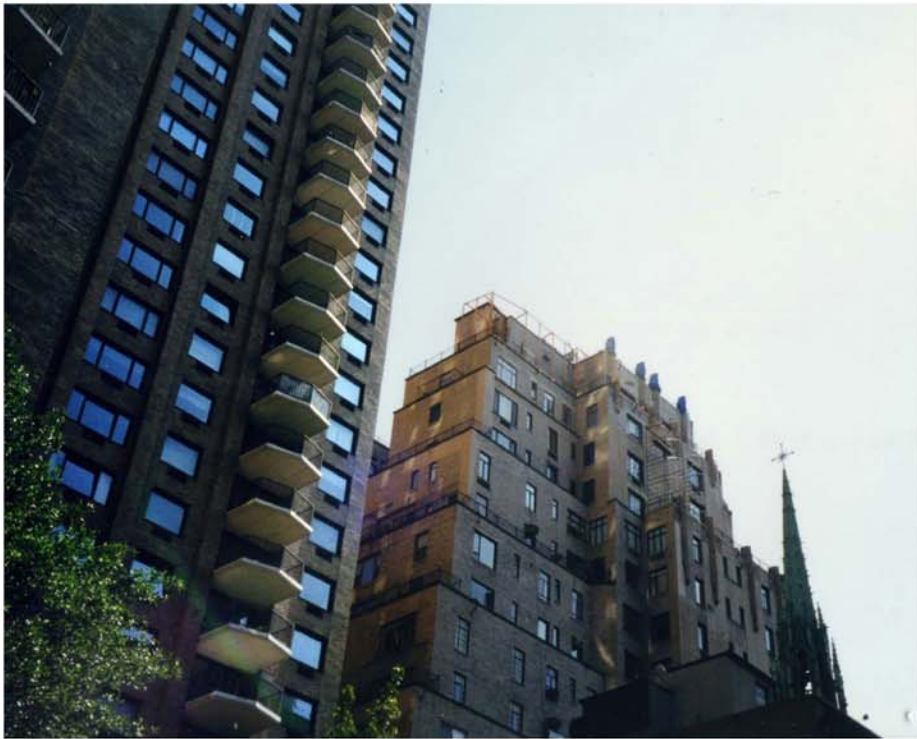
1 VIEW A FROM 65TH STREET EXISTING CONDITION WITH MOCK UP
