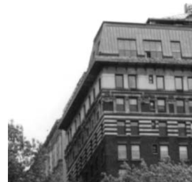
CONSTRUCTION OF THE TWO-STORY PENTHOUSE IS
