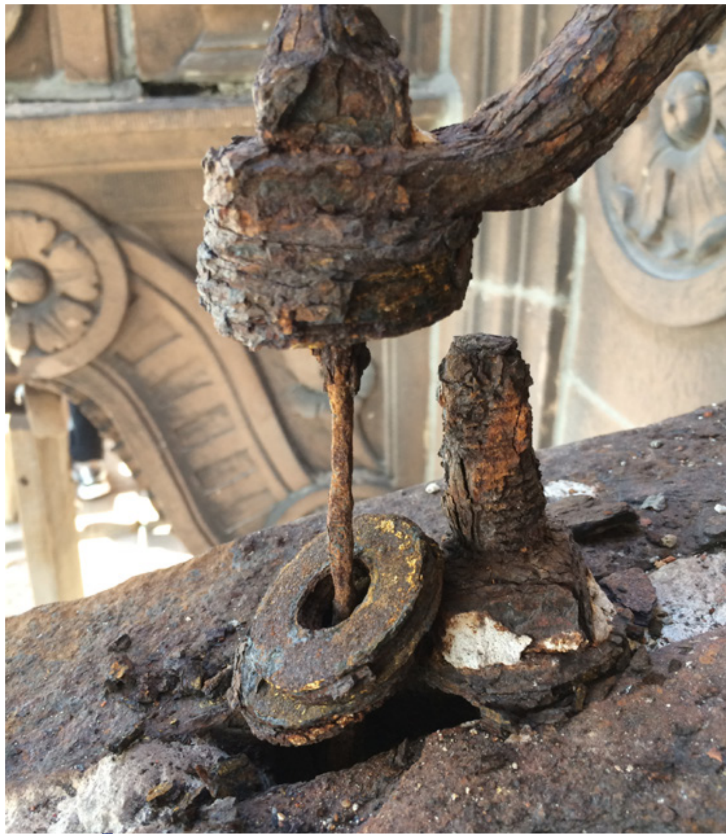
TYPICAL CORROSION AT STEEL ARMATURE
