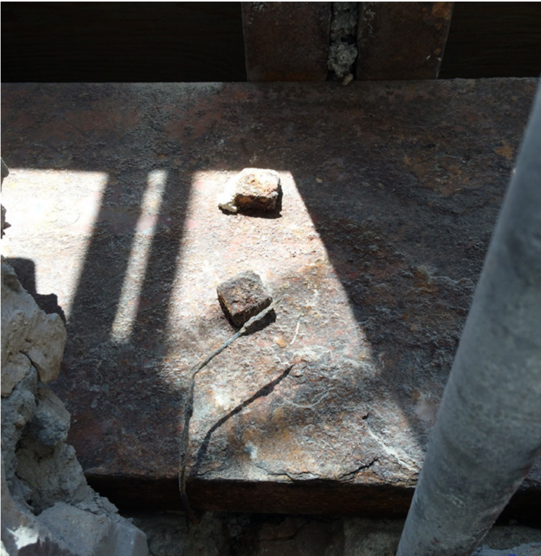
DETAIL OF STEEL CHANNEL SHOWING EVIDENCE OF SPALLING
