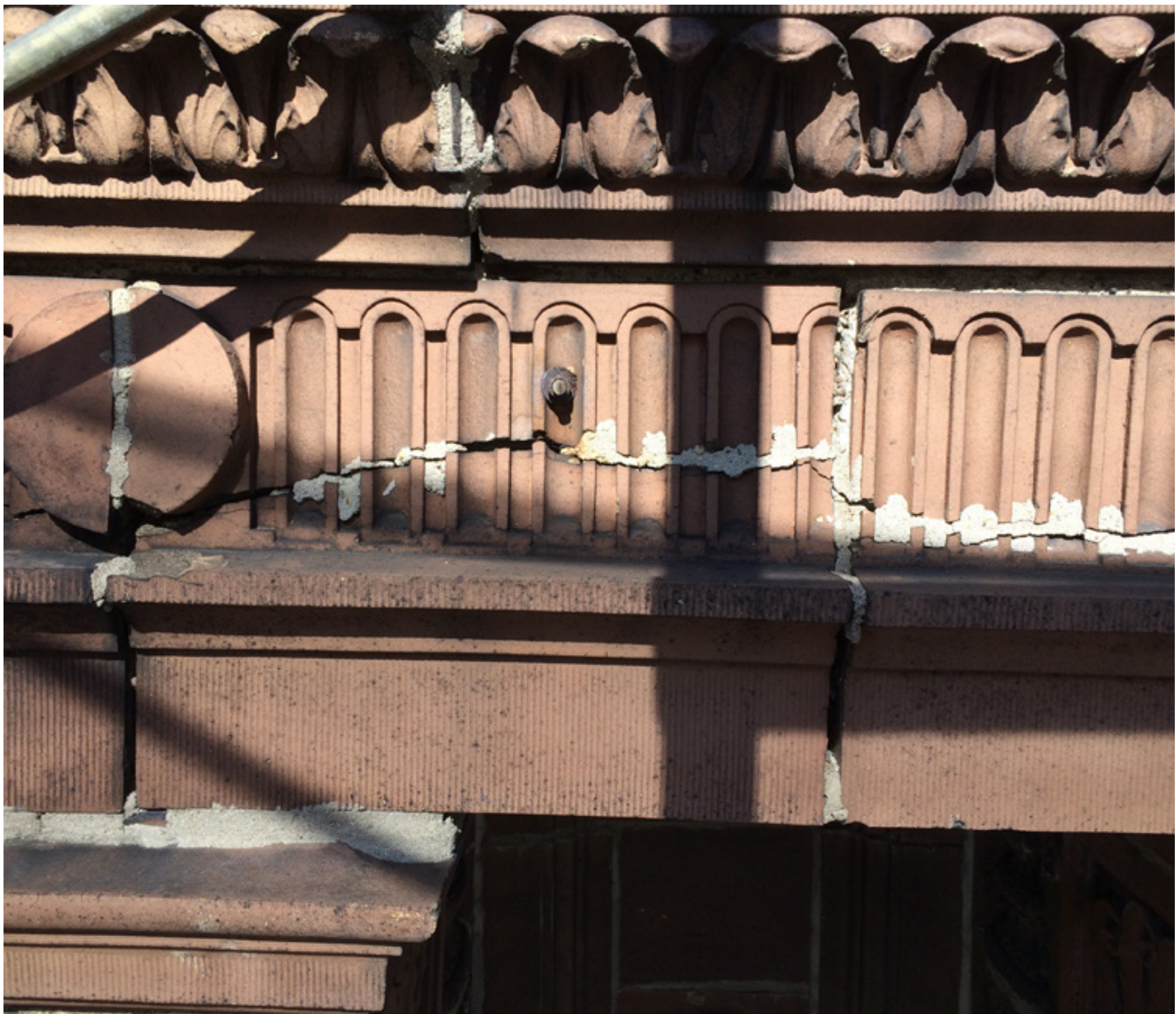
DAMAGED TERRA COTTA AT UPPER BAND COURSE
