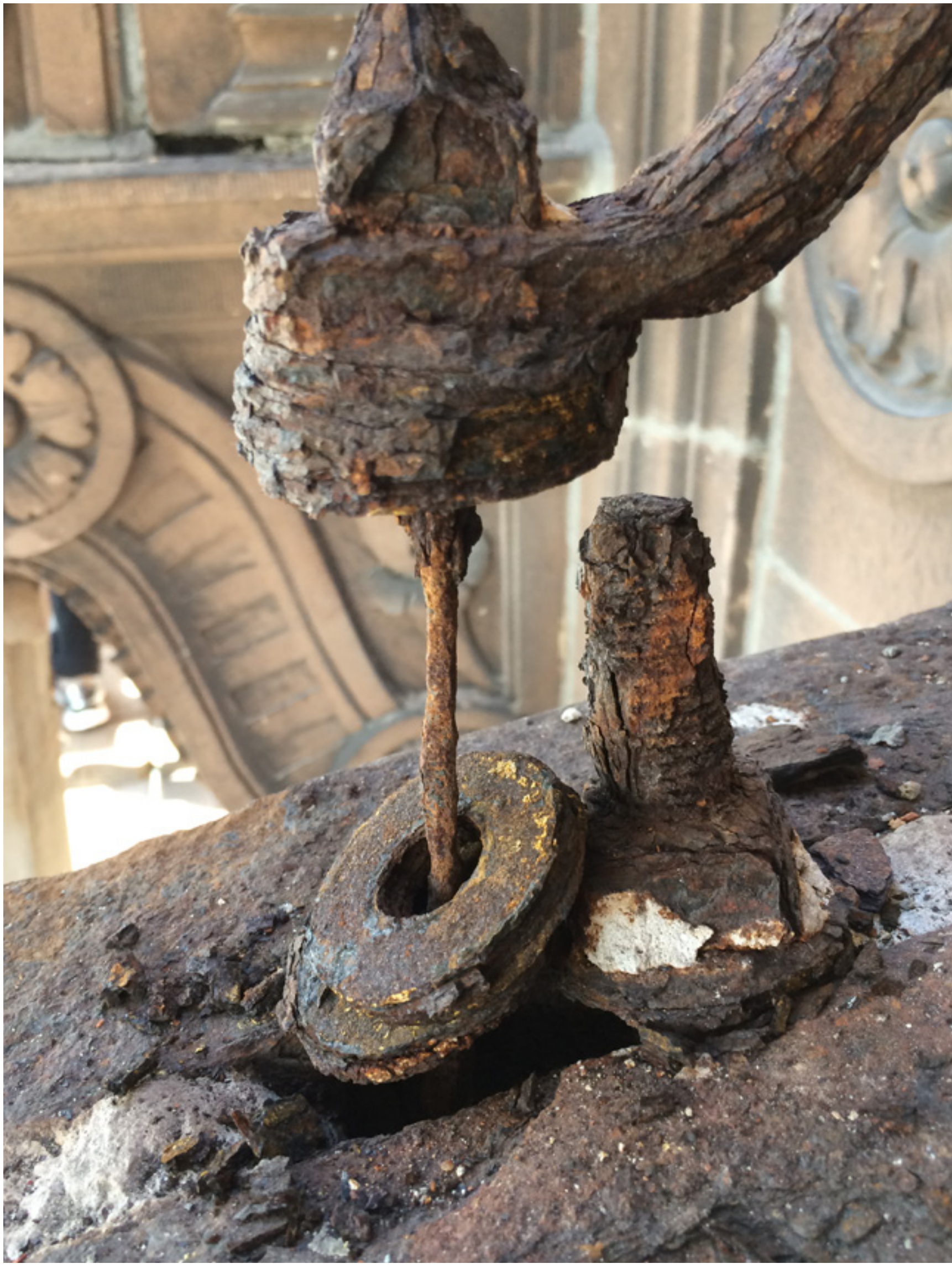
TYPICAL CORROSION AT STEEL ARMATURE
