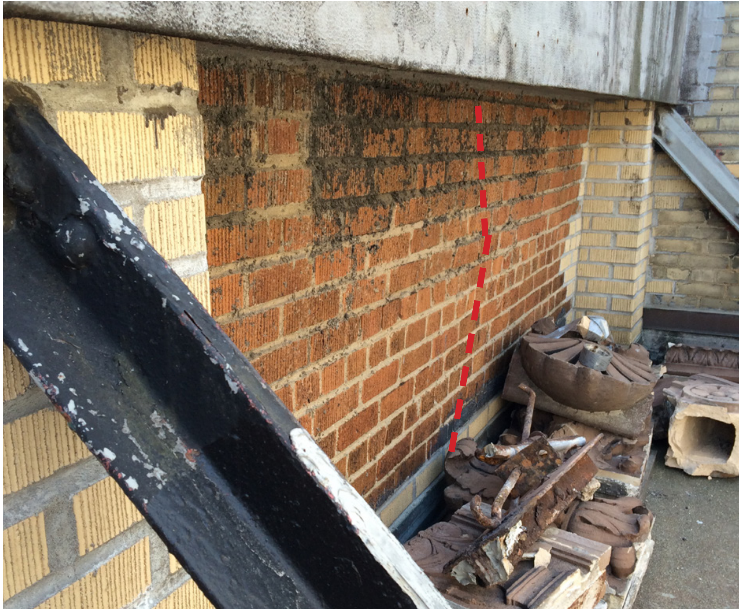
VIEW OF INBOARD SIDE OF CORNICE, SHOWING BULGE AT PARAPET WALL
