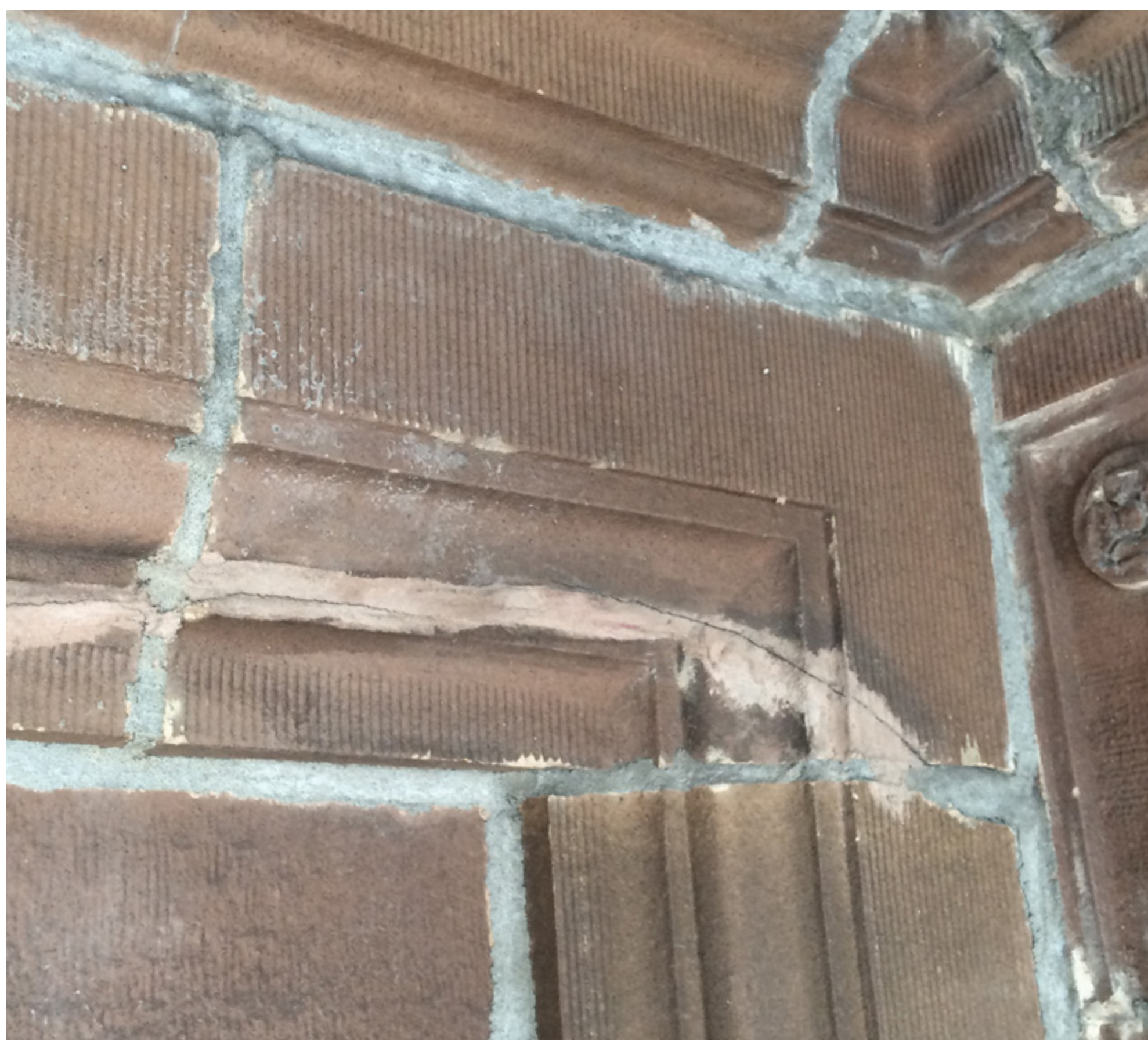
TYPICAL CRACKING NEAR LOCATION OF STEEL STRUCTURE
