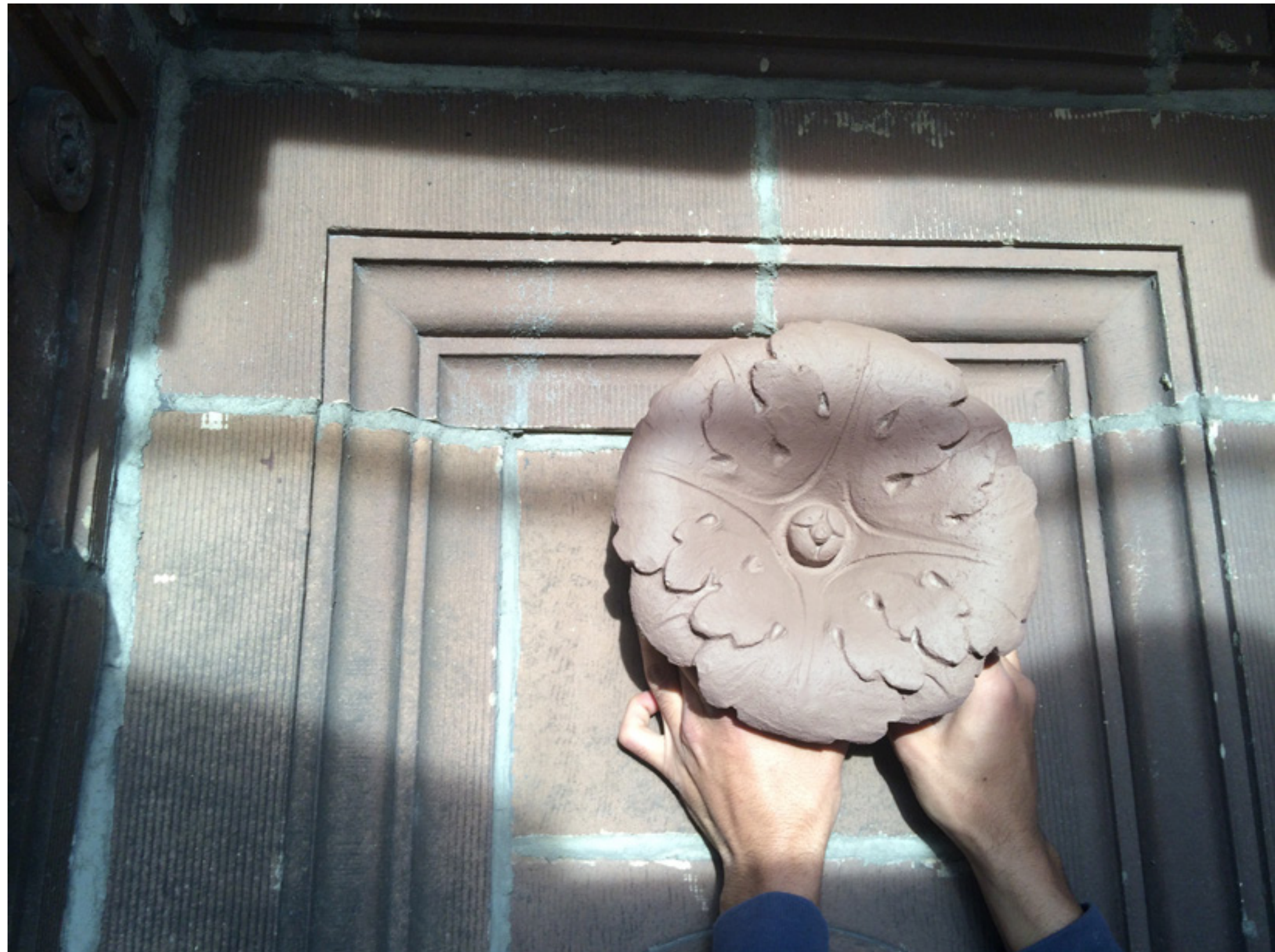
FIBERGLASS REPLACEMENT SAMPLE AND ORIGINAL TERRA COTTA (ON SITE)
