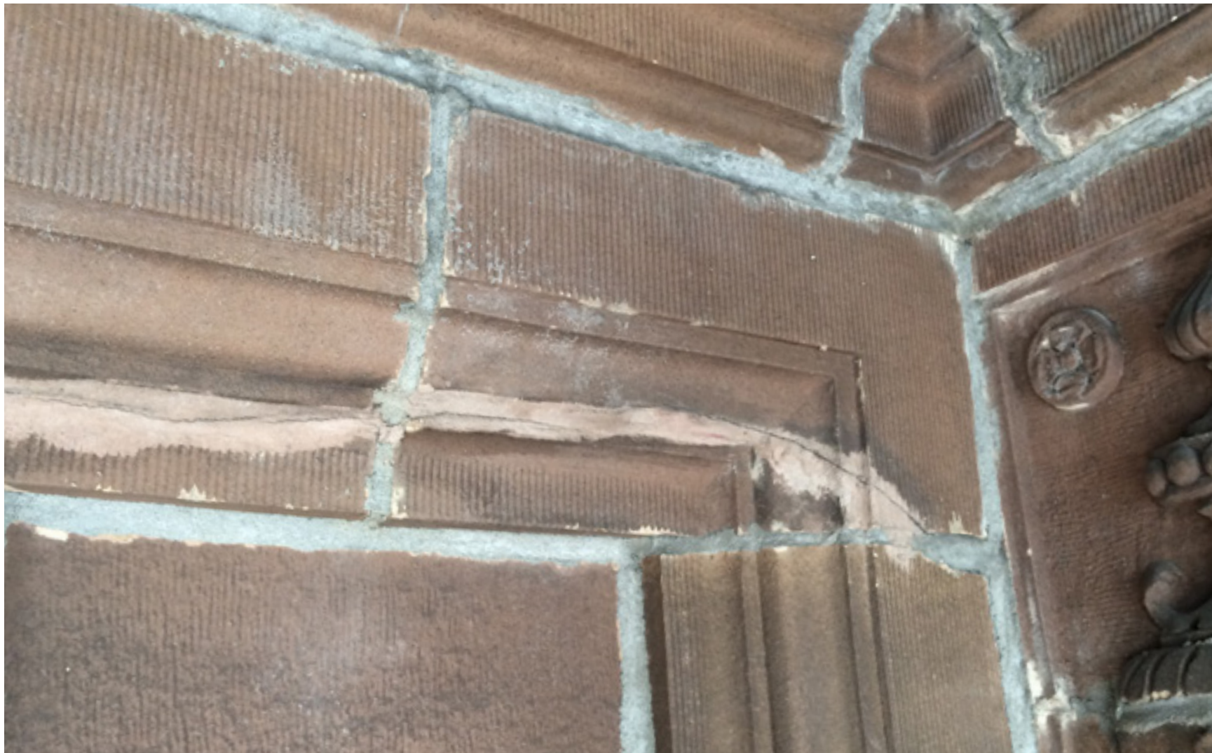
TYPICAL CORROSION AT STEEL ARMATURE
