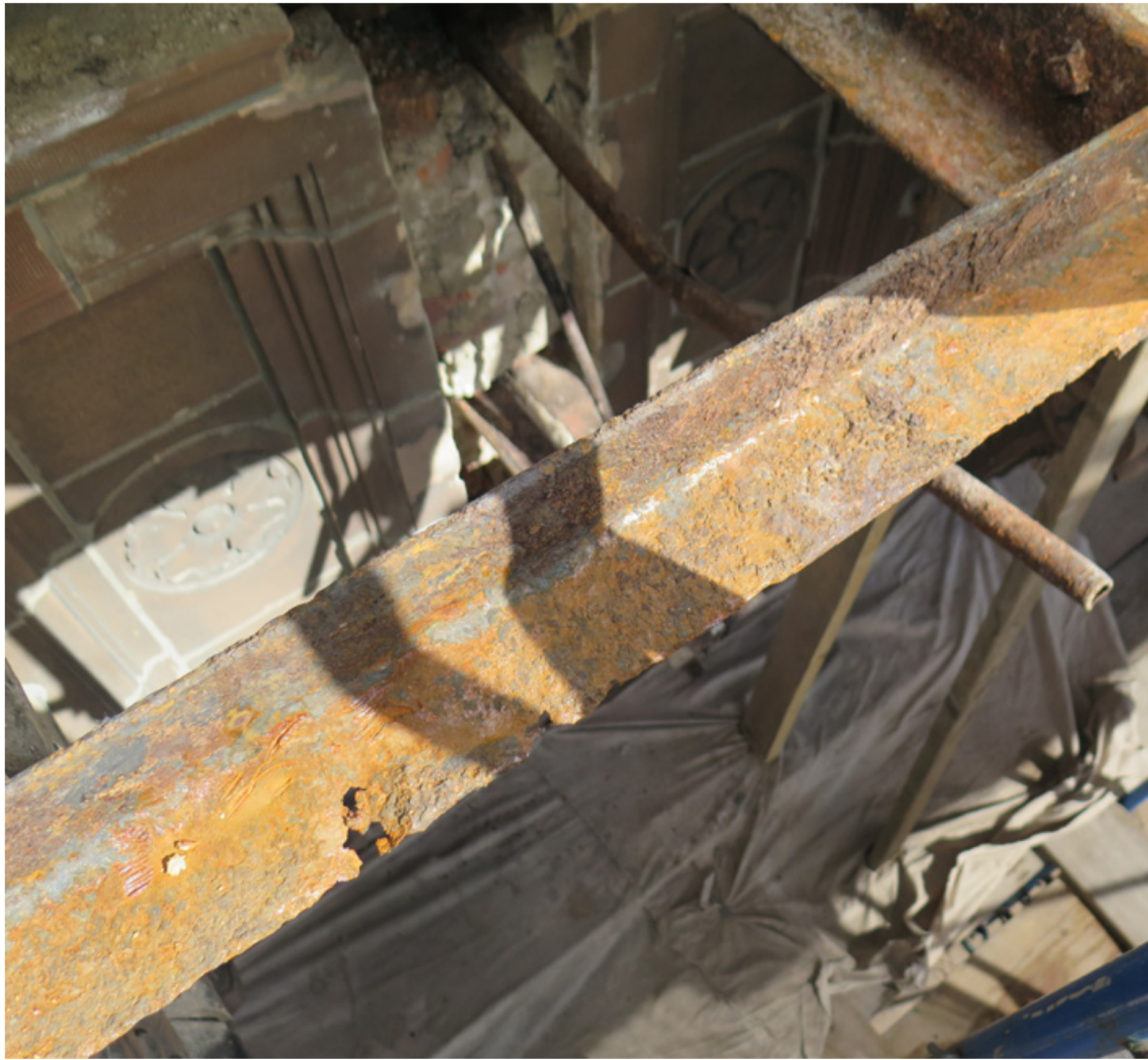
TYPICAL CORROSION AT STEEL ARMATURE
