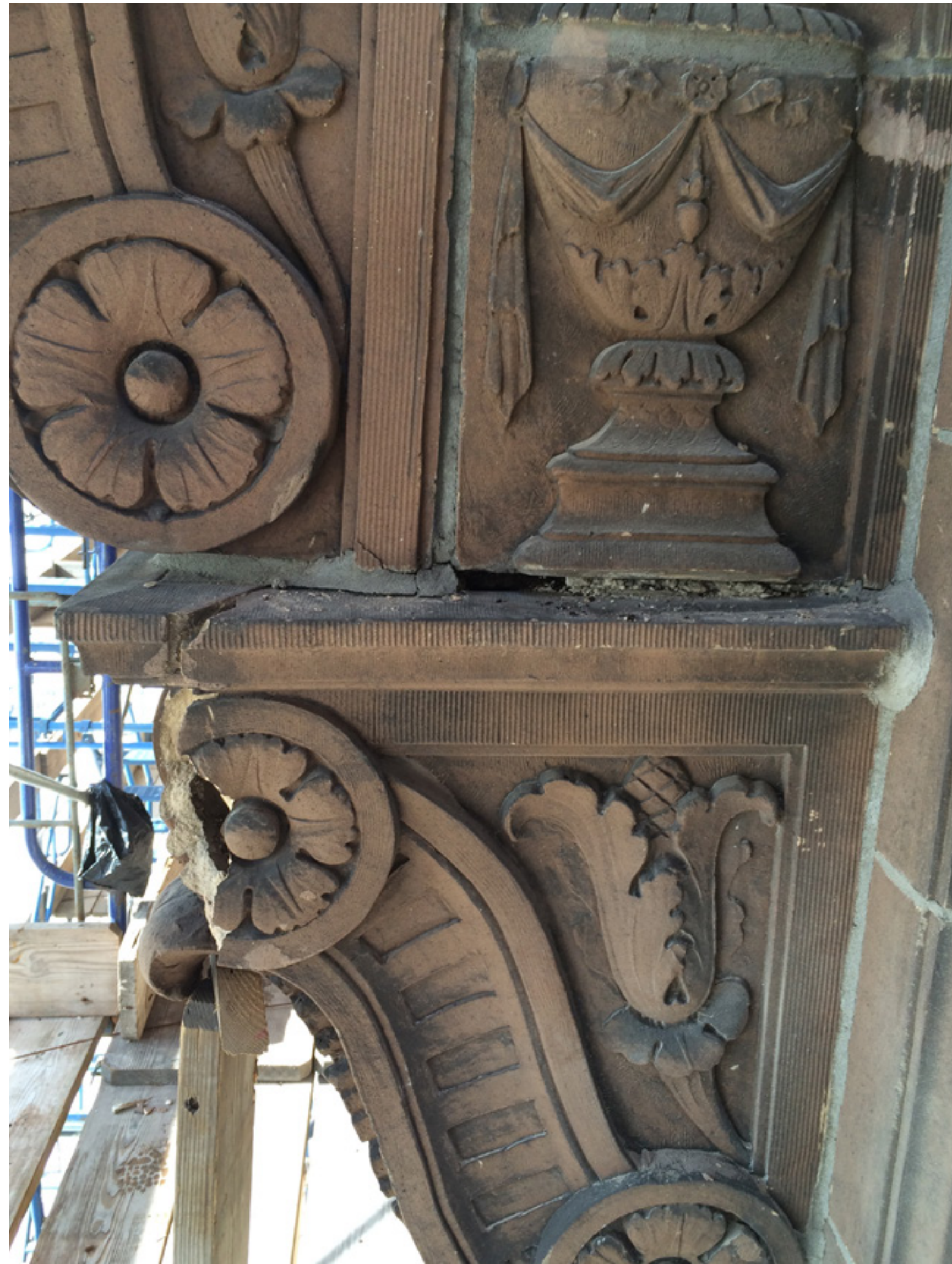
DAMAGED TERRA COTTA BRACKETS AND EXPANDED JOINTS
