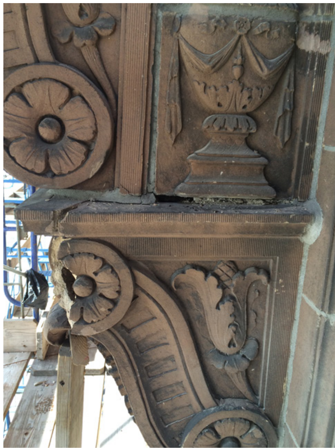
DAMAGED TERRA COTTA BRACKETS AND EXPANDED JOINTS
