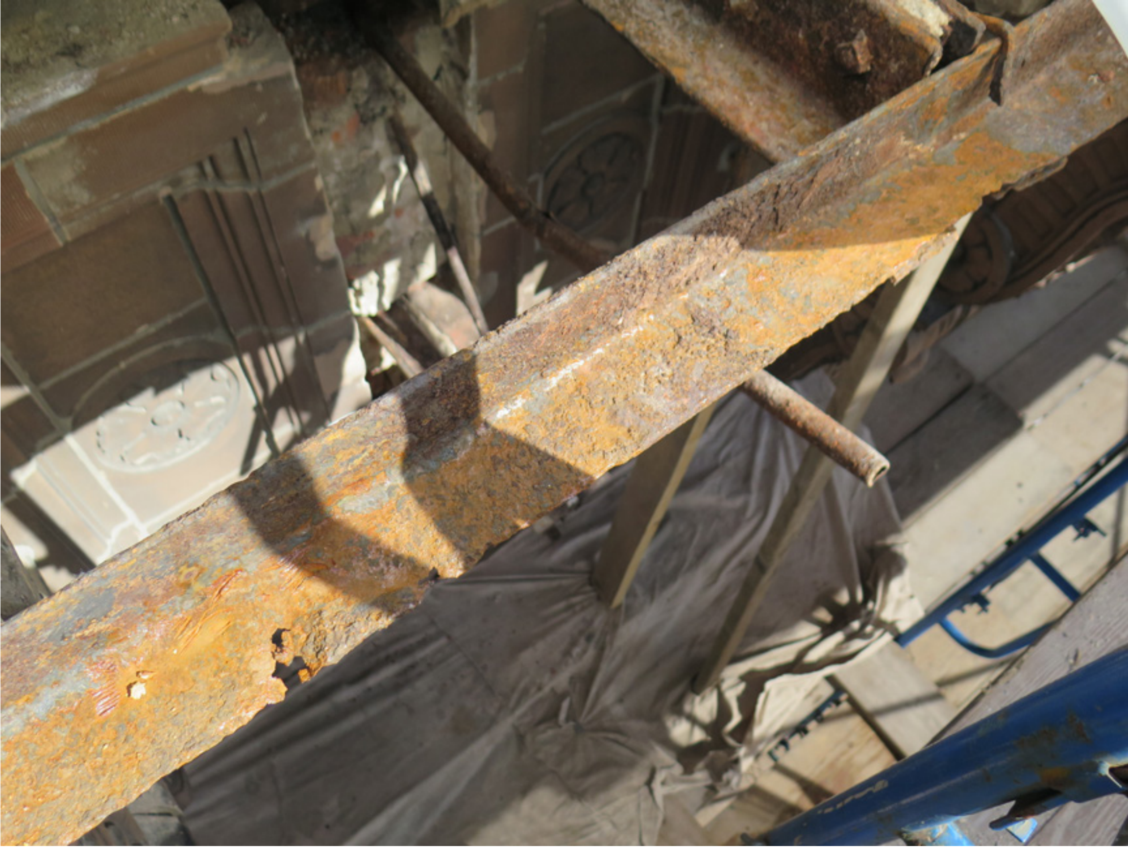
TYPICAL CORROSION AT STEEL ARMATURE
