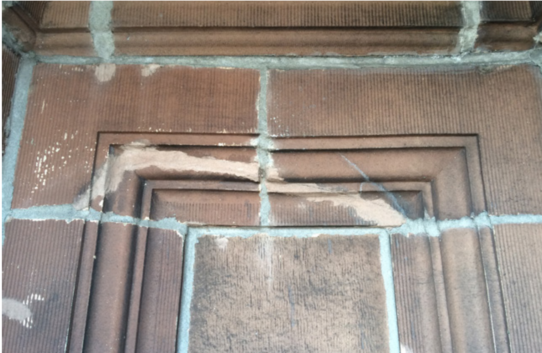
TYPICAL CRACKING NEAR LOCATION OF STEEL STRUCTURE
