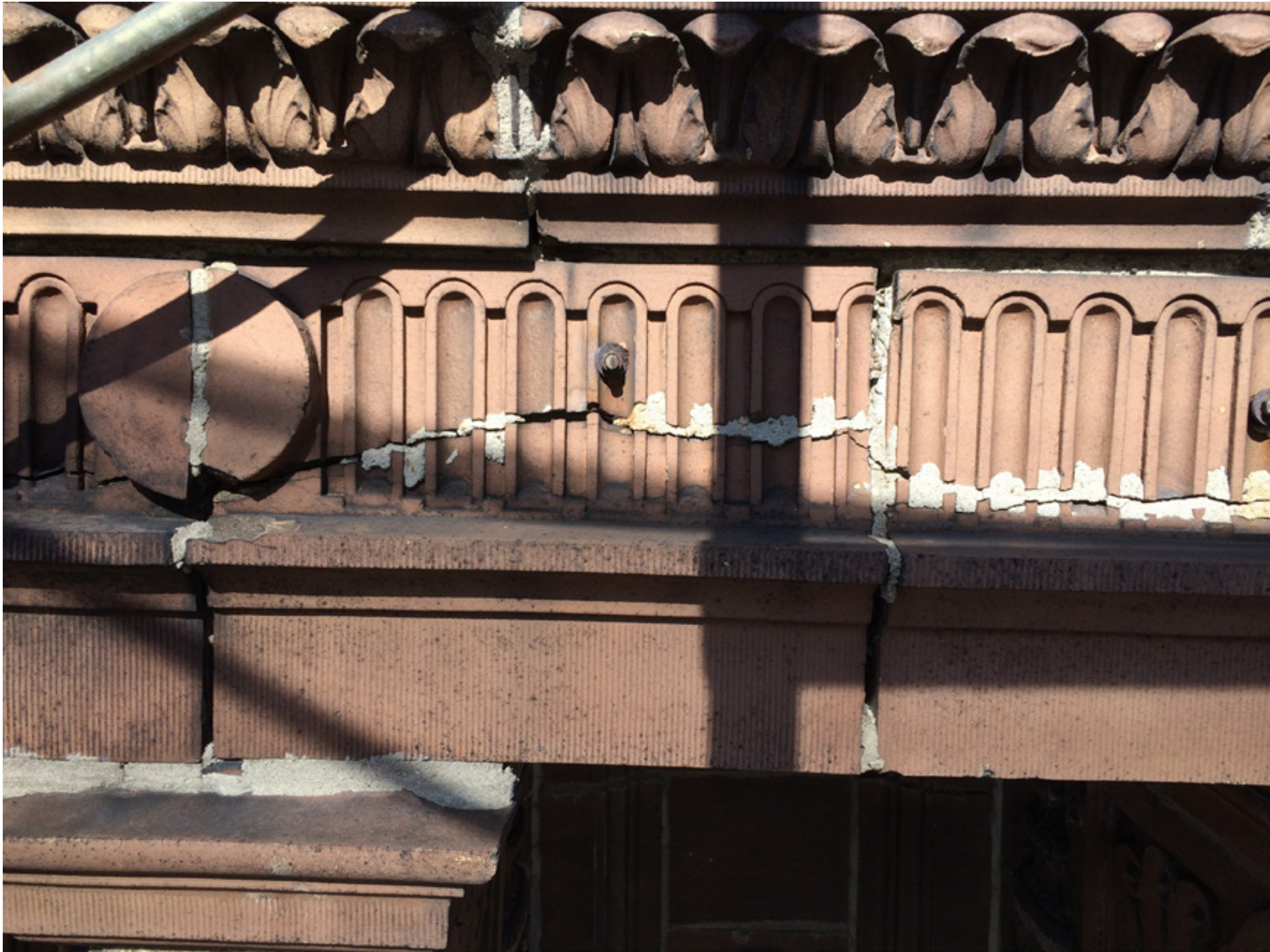
DAMAGED TERRA COTTA AT UPPER BAND COURSE
