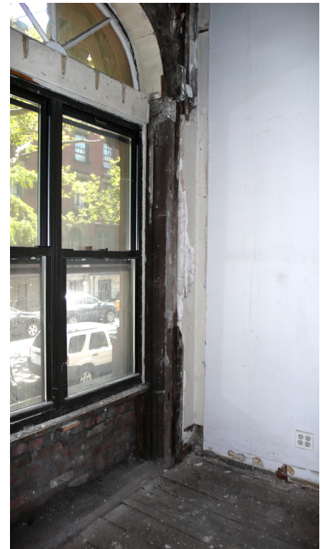
RIGHT SIDE SHOWING DOOR BLOCKING AND STONE SADDLE
