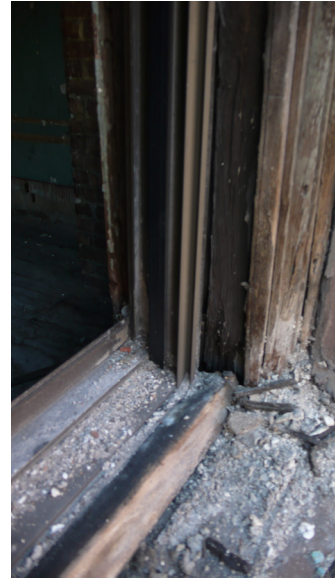
BRICK MOLD UNDERNEATH EXTERIOR CASING OF REPLACEMENT WINDOWS
