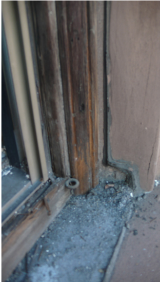
BRICK MOLD UNDERNEATH EXTERIOR CASING OF REPLACEMENT WINDOWS
