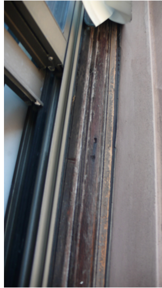
BRICK MOLD UNDERNEATH EXTERIOR CASING OF REPLACEMENT WINDOWS
