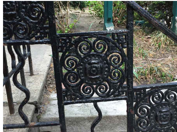
PHOTOS OF EXISTING RAILING - MEDALLIONS AND GENERAL DIMENSION OF NEW GATES TO MATCH EXISTING
