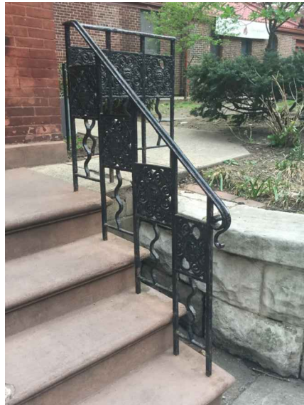
PHOTOS OF EXISTING RAILING - MEDALLIONS AND GENERAL DIMENSION OF NEW GATES TO MATCH EXISTING
