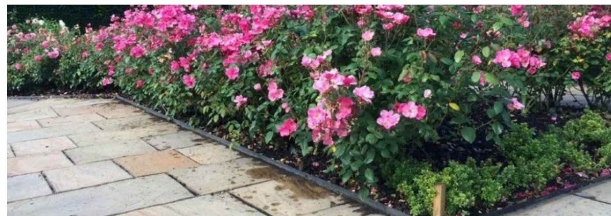
Ⓜ EXAMPLE OF STEEL EDGING TO SEPARATE PAVED AREA FROM PLANTING
