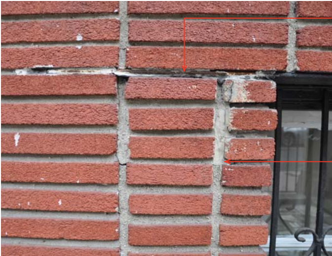
EXPOSED STRUCTURAL LINTEL WITH POTENTIAL WATER DAMAGE
