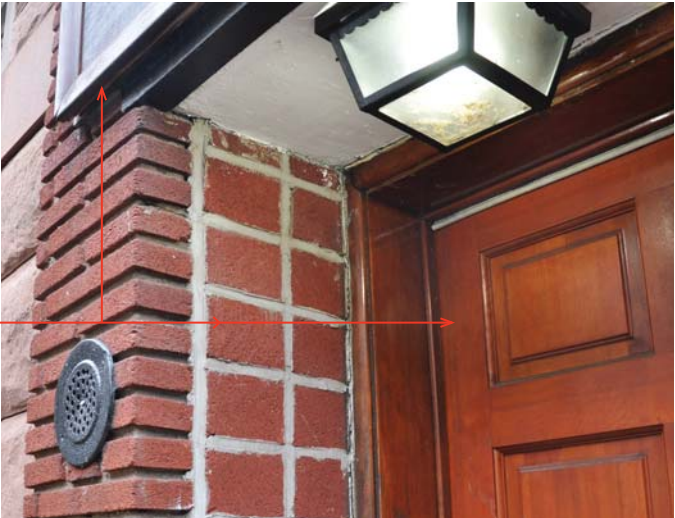
THIN BRICK VENEER AT THRESHOLD, WOOD DOOR AND VALENCE ARE NOT ORIGINAL NOR PART OF THE IFILL & JOHNSON RENOVATION
