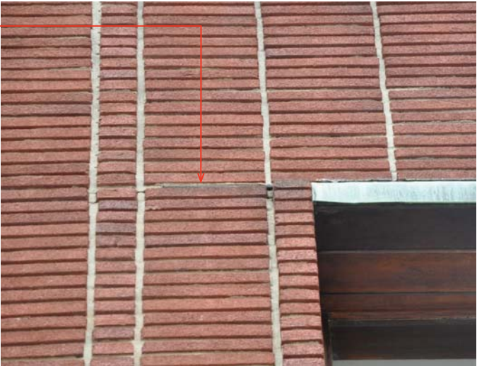
EXPOSED STRUCTURAL LINTEL WITH POTENTIAL WATER DAMAGE
