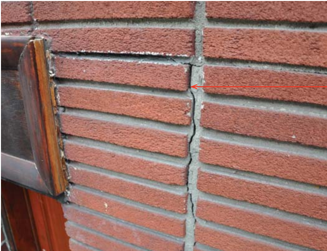
CRACKING AT VENEER BRICK FACADE, TYPICAL NEAR OPENINGS
