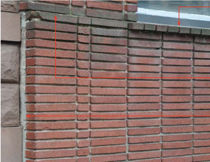
BRICK SILL WITH OVERSIZED RAKED MORTAR JOINTS, VISIBLE WATER DAMAGE
