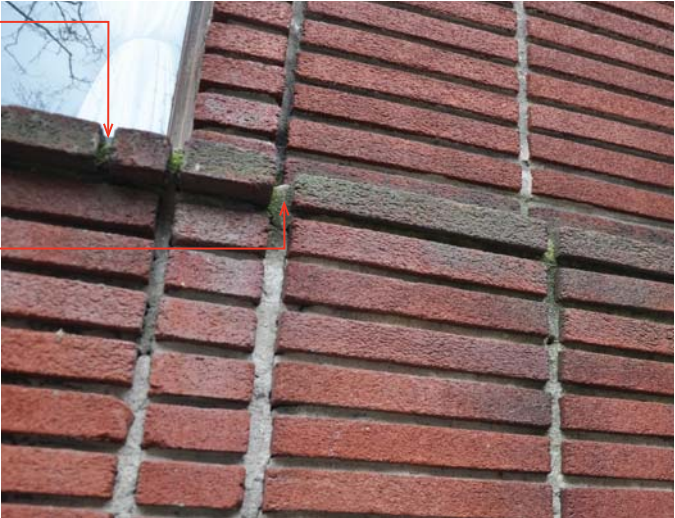
BRICK SILL WITH OVERSIZED RAKED MORTAR JOINTS, VISIBLE WATER DAMAGE
