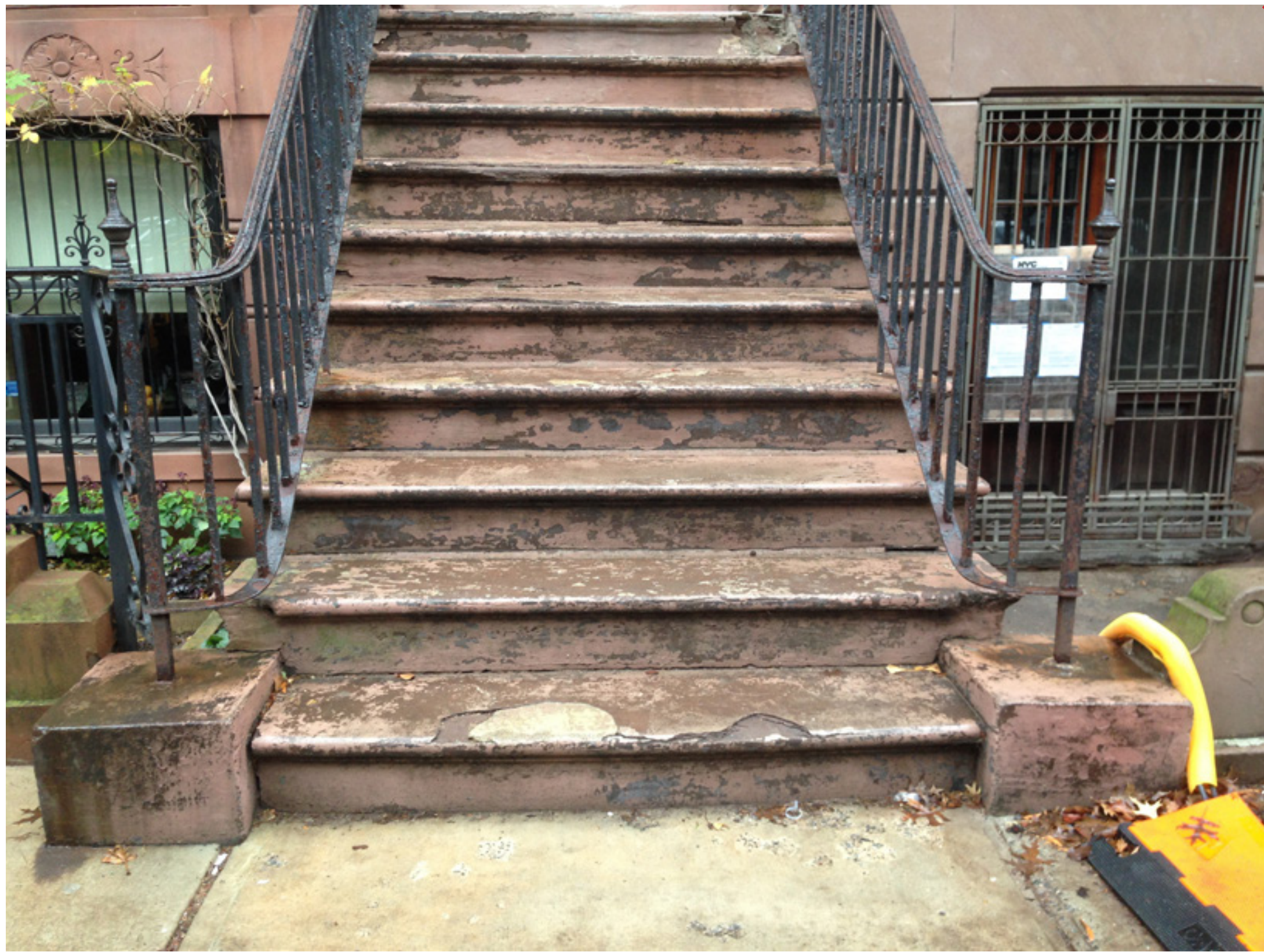
125 West 87th Street - Stoop to be rebuilt to match existing
