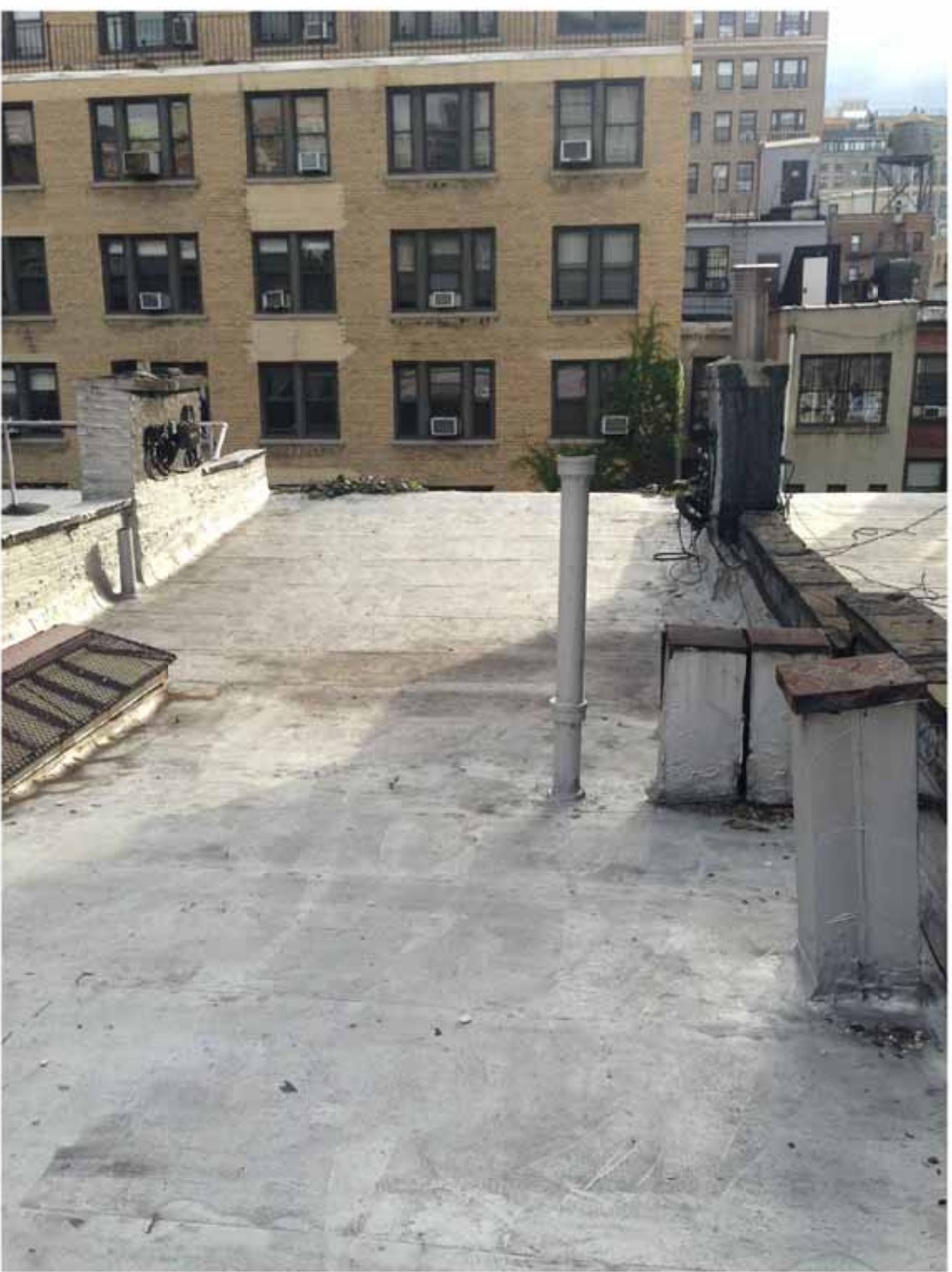
2 | EXISTING ROOF CONDITION LOOKING SOUTHWEST LPC-12 NO SCALE
