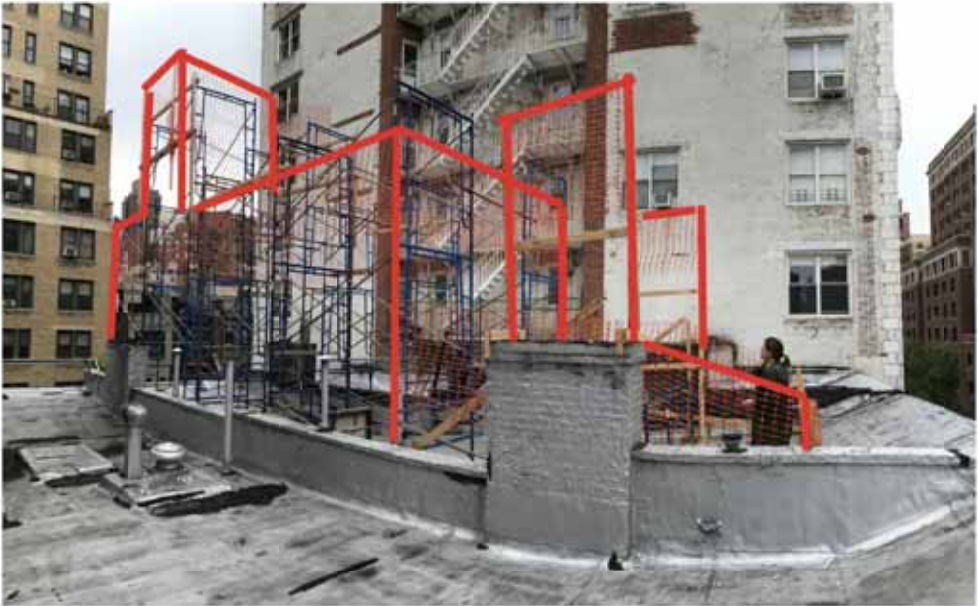
2 122 W. 73RD ST. ROOFTOP ADDITION VIEW FROM ROOF OF 120 W. 73RD ST. LPC-5G NO SCALE
