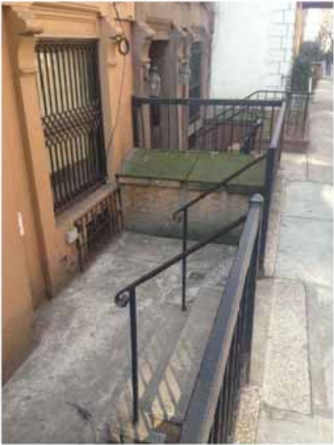
2 | EXISTING AREAWAY LPC-10 | NO SCALE
