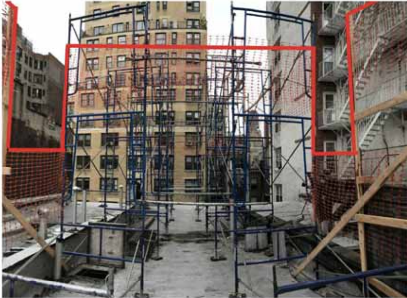
3 122 W. 73RD ST. ROOFTOP ADDITION VIEW FROM ROOF OF 122 W. 73RD ST. LPC-5G NO SCALE
