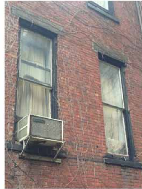
8 EXISTING REAR WINDOW EXTERIOR PHOTO LPC-12 NO SCALE
