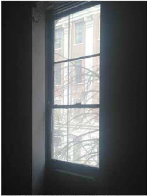
1 EXISTING FRONT WINDOW INTERIOR PHOTO LPC-12 NO SCALE
