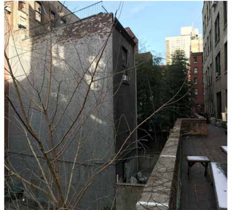
4 VIEW FROM 2ND FL. OF 119 W. 72ND ST. LOOKING NORTHEAST LPC-5E NO SCALE
