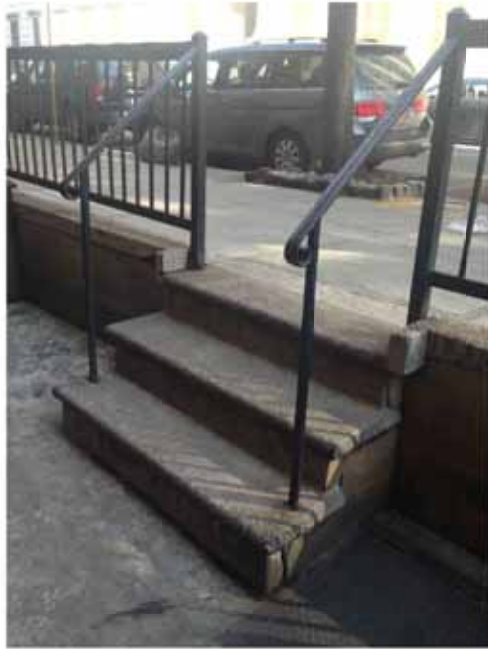
3 | EXISTING AREAWAY LPC-10 | NO SCALE
