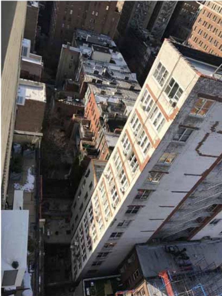
1 VIEW FROM 16TH FL. OF 119 W. 72ND ST. LOOKING NORTHWEST LPC-5D NO SCALE
