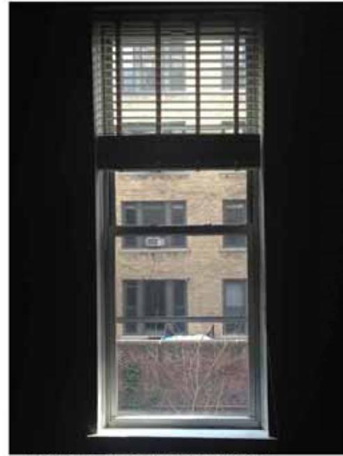
3 EXISTING REAR WINDOW INTERIOR PHOTO LPC-12 NO SCALE
