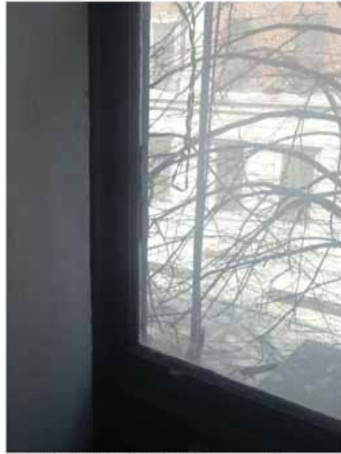
2 EXISTING FRONT WINDOW INTERIOR PHOTO LPC-12 NO SCALE
