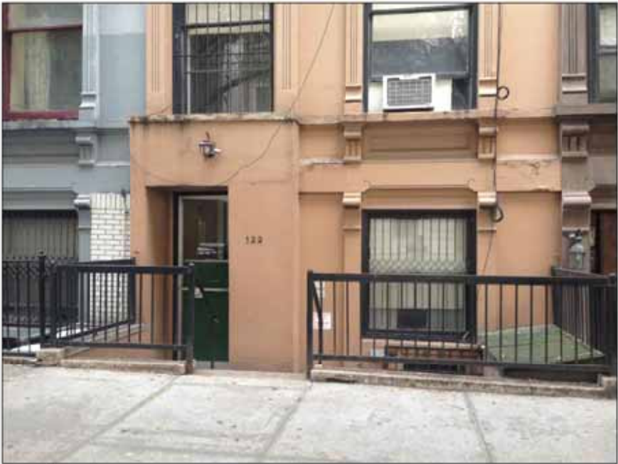
4 | EXISTING AREAWAY LPC-10 | NO SCALE
