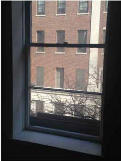
5 EXISTING FRONT WINDOW INTERIOR PHOTO LPC-12 NO SCALE
