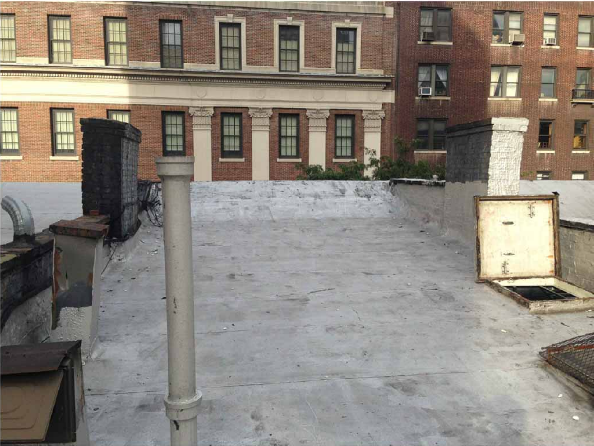
1 | EXISTING ROOF CONDITION LOOKING NORTHEAST LPC-12 NO SCALE
