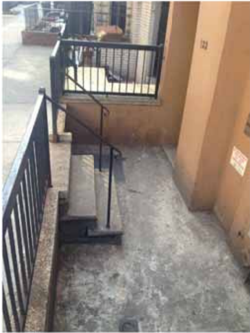
1 | EXISTING AREAWAY LPC-10 | NO SCALE
