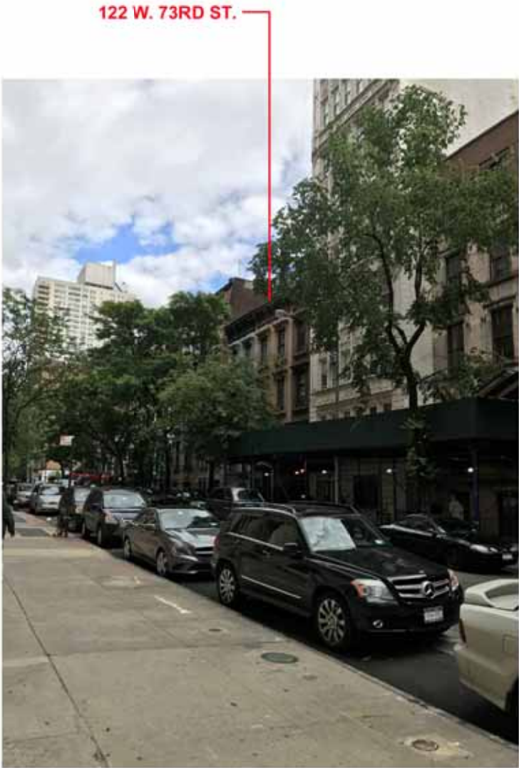
3 VIEW FROM 125 W. 73RD ST. LOOKING SOUTHEAST LPC-5B (ROOFTOP ADDITION NOT VISIBLE)
