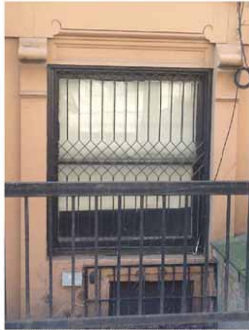
6 EXISTING FRONT BASEMENT WINDOW EXTERIOR PHOTO LPC-12 NO SCALE
