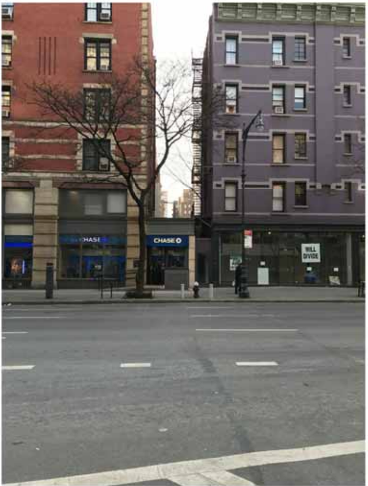
4 122 W. 73RD ST. REAR ADDITION VIEW FROM EAST SIDE OF COLUMBUS AVE. LPC-5F (ADDITION NOT VISIBLE)
