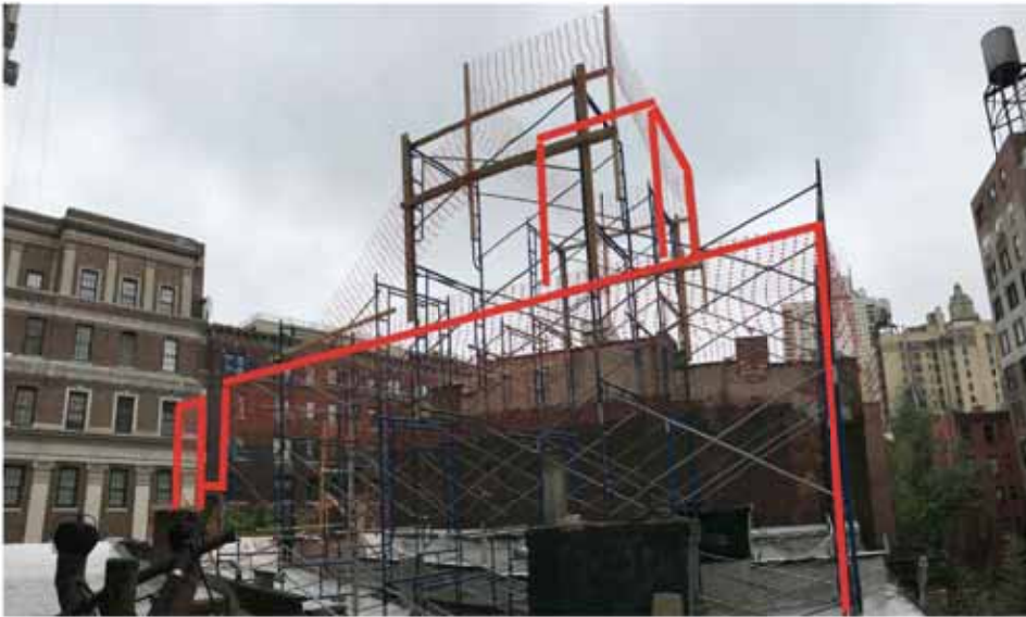
5 122 W. 73RD ST. ROOFTOP ADDITION VIEW FROM ROOF OF 124 W. 73RD ST. LPC-5G NO SCALE
