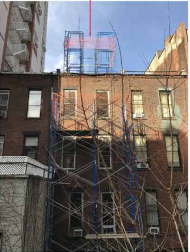
3 VIEW FROM 2ND FL. OF 119 W. 72ND ST. LOOKING NORTH LPC-5E NO SCALE
