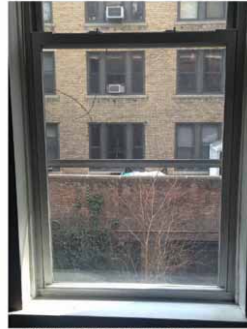
4 EXISTING REAR WINDOW INTERIOR PHOTO LPC-12 NO SCALE
