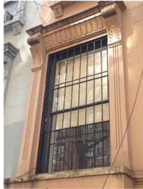
7 EXISTING FRONT FIRST FLOOR WINDOW EXTERIOR PHOTO LPC-12 NO SCALE
