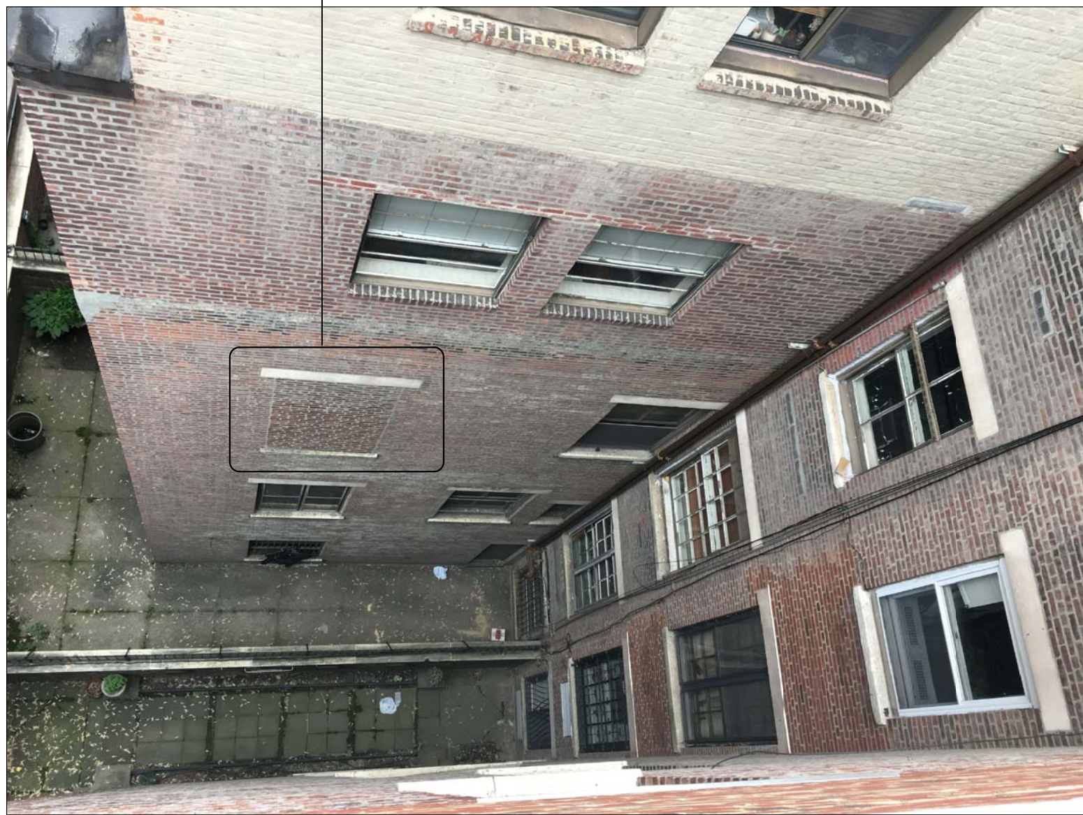
5 PHOTO OF CLOSE-UP VIEW BOTTOM WINDOWS OF THE BLDG.
