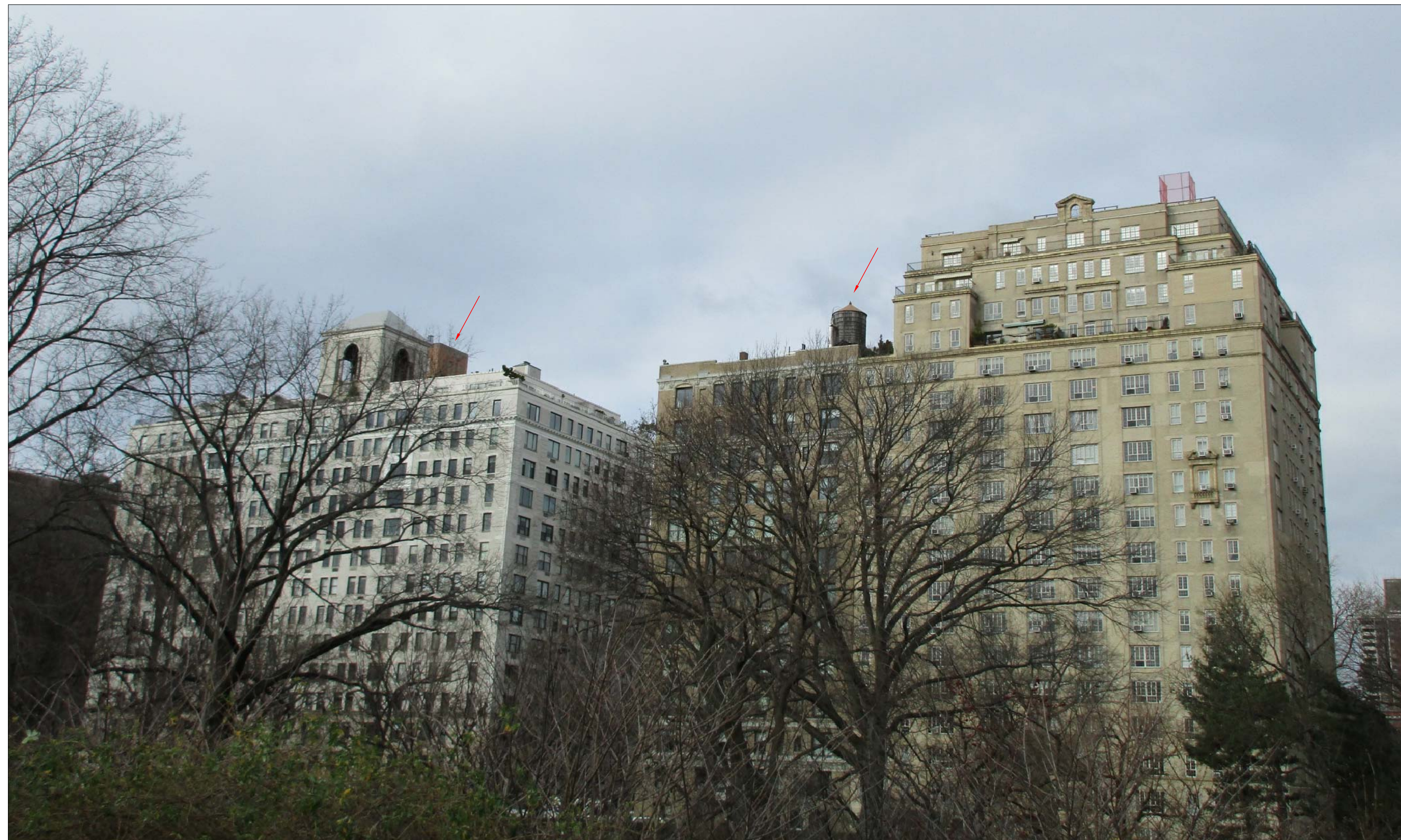
J 262 & 271 CENTRAL PARK WEST - VIEW OF ROOFTOP BULKHEAD AND WATER TOWER FROM CENTRAL PARK
