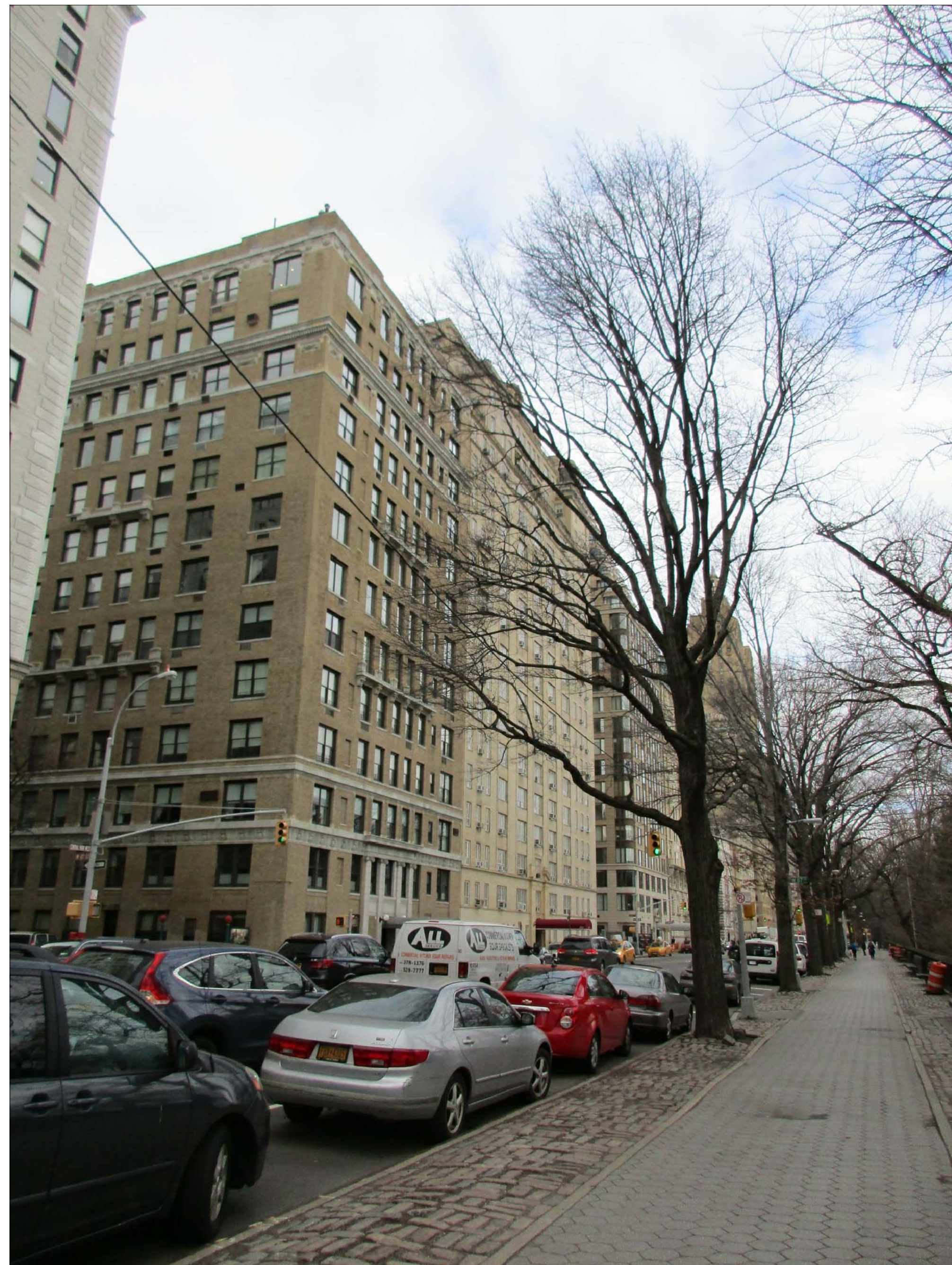
A VIEW FROM THE SOUTH ON CENTRAL PARK WEST (NOTE THAT THE BULKHEAD EXTENSION IS NOT VISIBLE)
