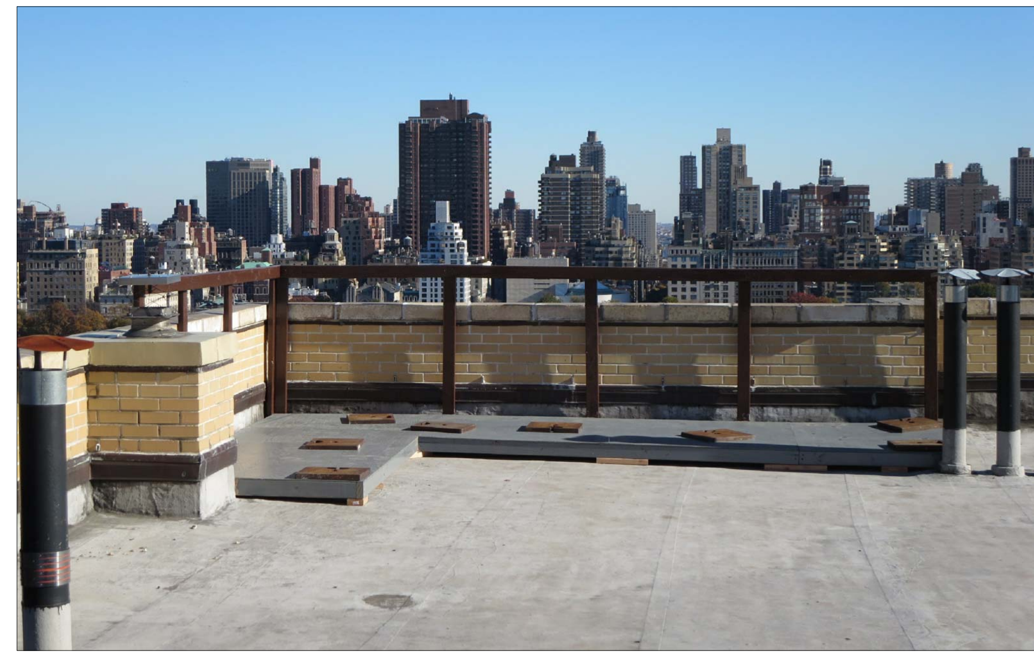
I VIEW OF GUARDRAIL MOCKUP AT THE EAST ELEVATION
