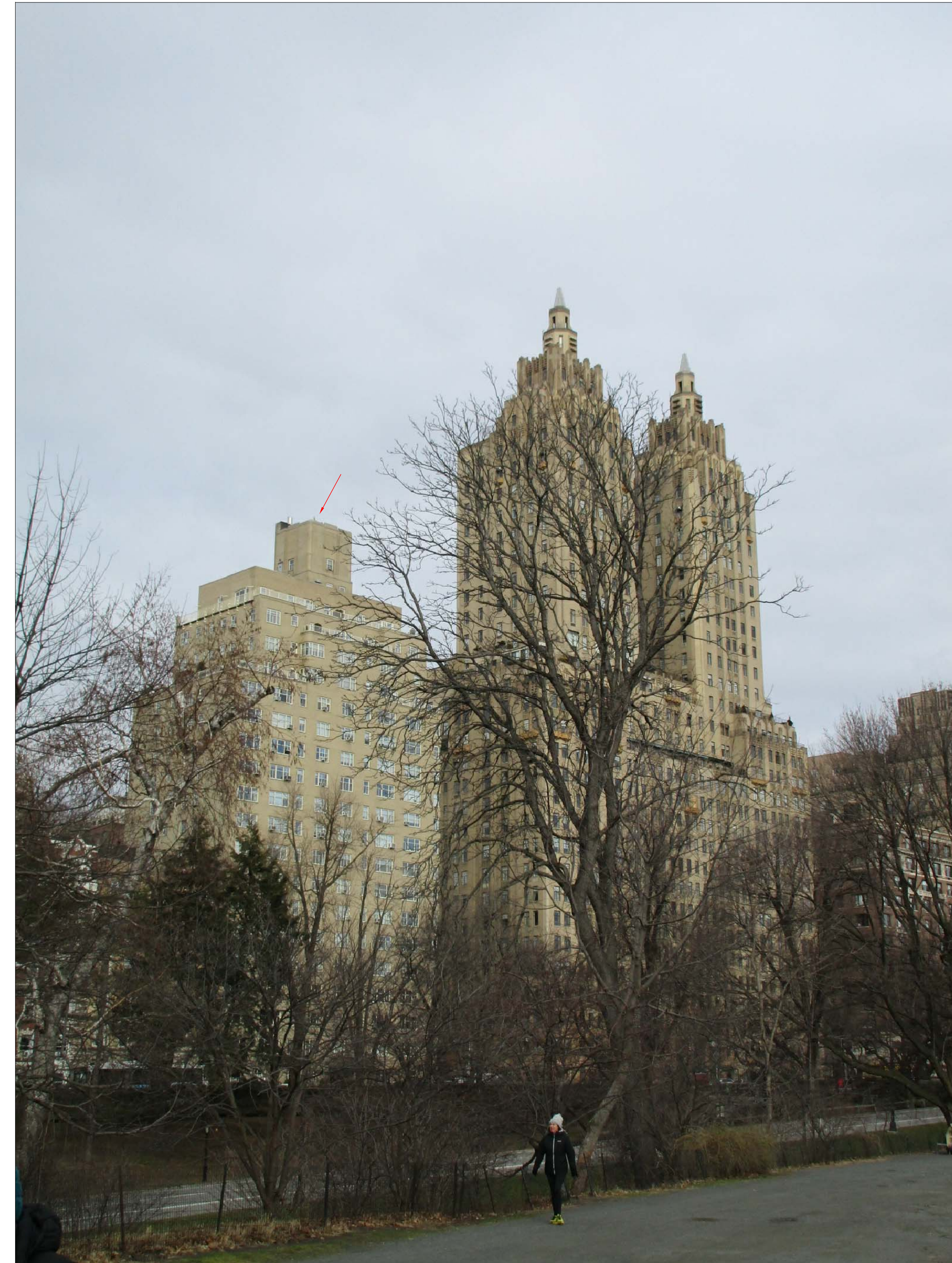
I 295 CENTRAL PARK WEST - VIEW OF ROOFTOP BULKHEAD FROM CENTRAL PARK
