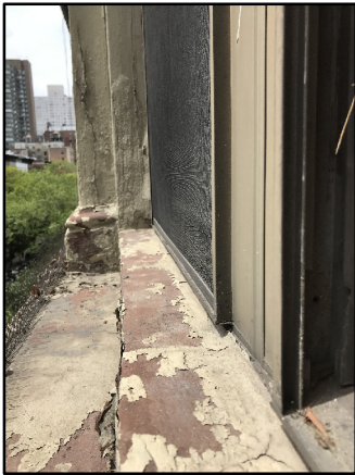
EXISTING 4TH FL SILL SHOWING PANNING
