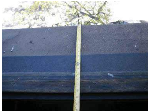
PHOTO OF EXISTING TYPICAL SILL
