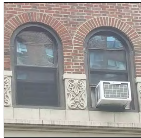
Existing Alum. DH Exterior View
