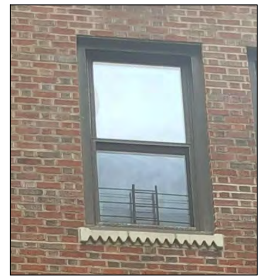
Existing Alum. DH Exterior View
