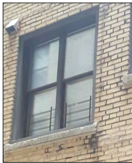
Existing Alum. DH Exterior View
