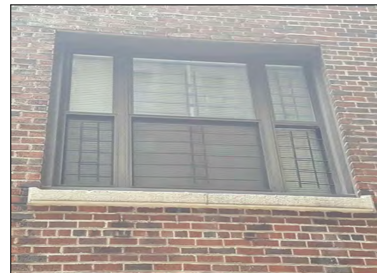
Existing Alum. DH Exterior View
