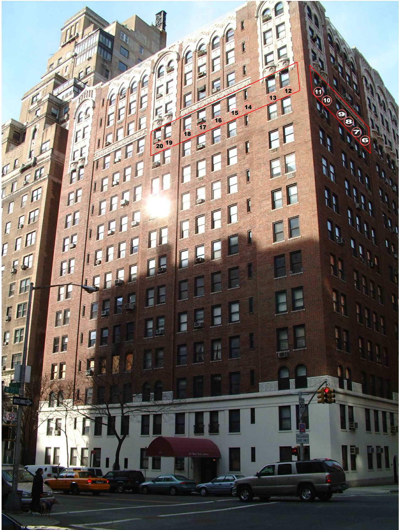
EXISTING WINDOW CONDITION EXTERIOR VIEW
