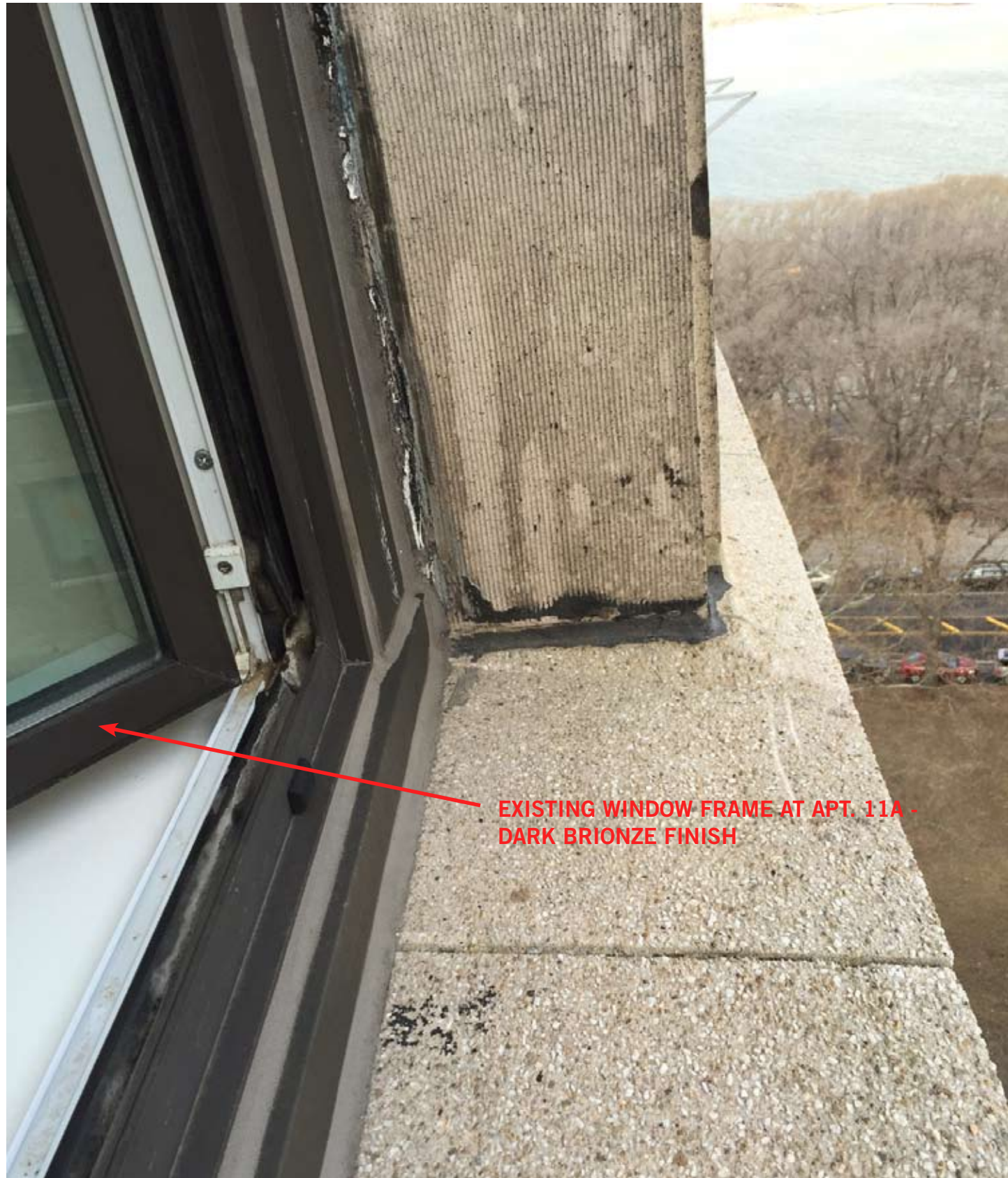
VIEW OF EXISTING WINDOW AND FLASHING - DARK BRONZE
