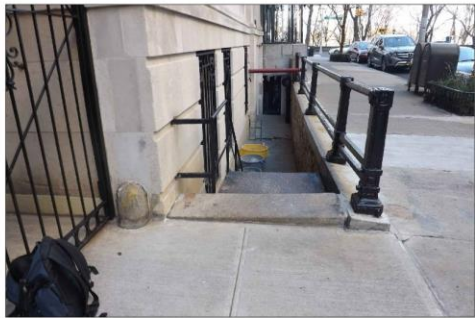
EXISTING LIGHT WELL VIEW FROM STREET
