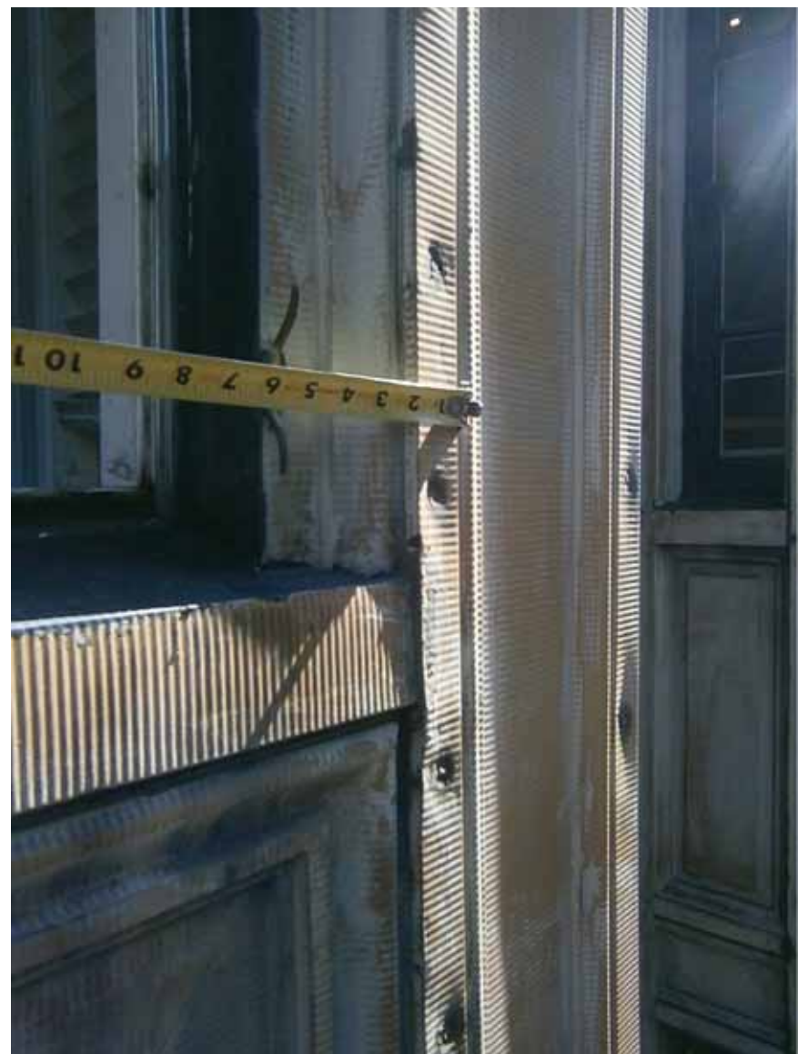
EXTERIOR CONDITION AT COPPER CLADDING W/TAPE MEASURE WINDOW TYPE : C
