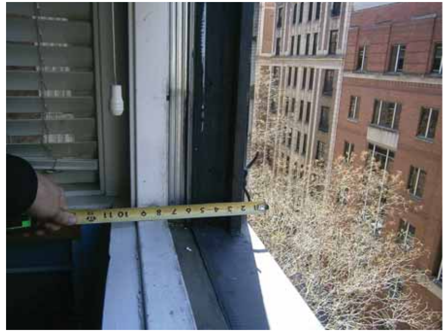
JAMB CONDITION WINDOW TYPE : C
