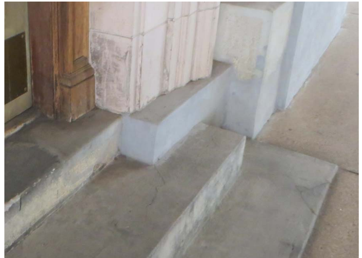
IMAGE 3: EXISTING STEPS WITH CRACKS AND DELAMINATION AND BLUESTONE BASE BEHIND WITH PREVIOUS PATCH REPAIRS
