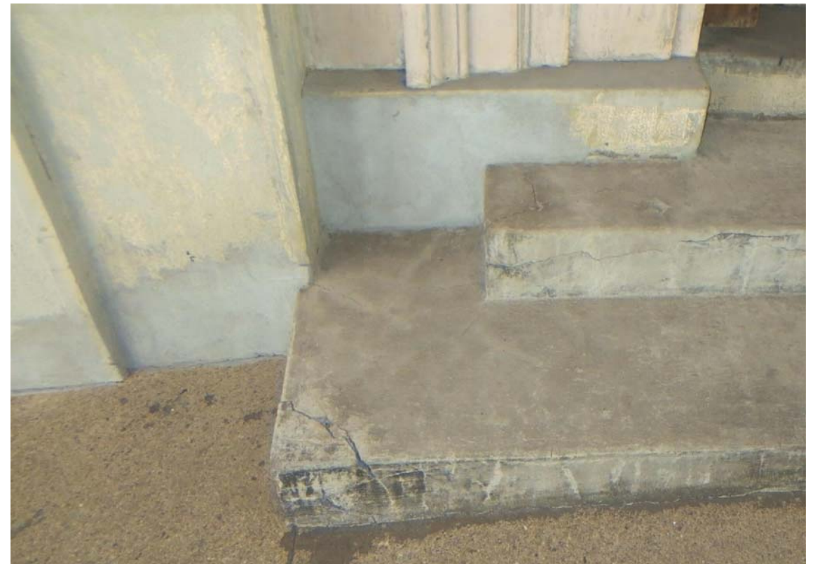
IMAGE 2: EXISTING STEPS WITH CRACKS AND DELAMINATION AND BLUESTONE BASE BEHIND WITH PREVIOUS PATCH REPAIRS
