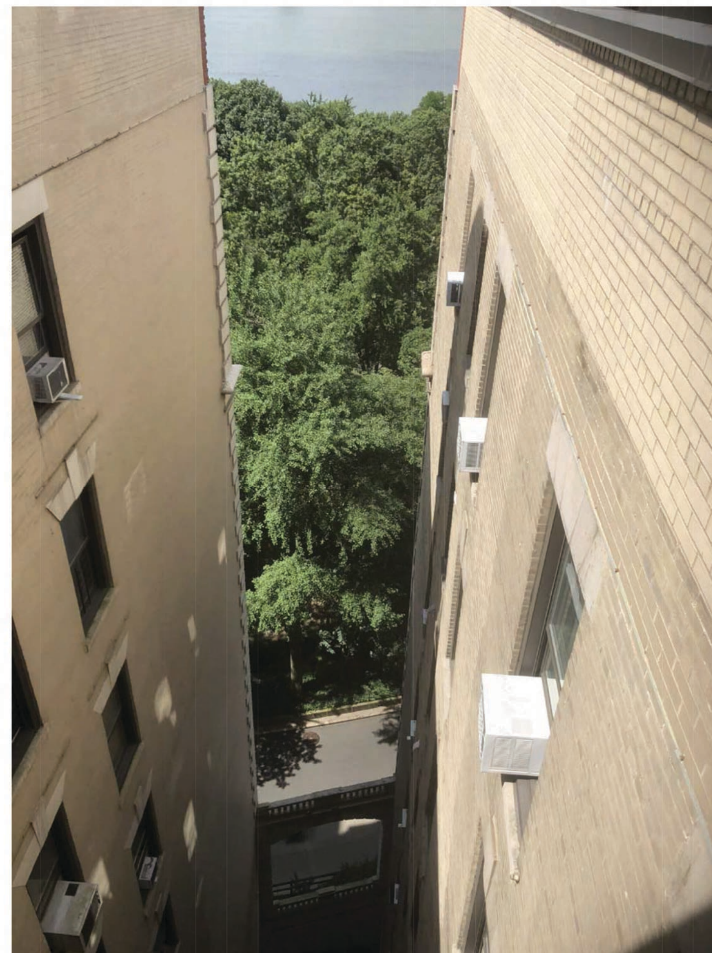
② VIEW FROM ROOF LOOKING THROUGH NORTH COURTYARD AT RSD
