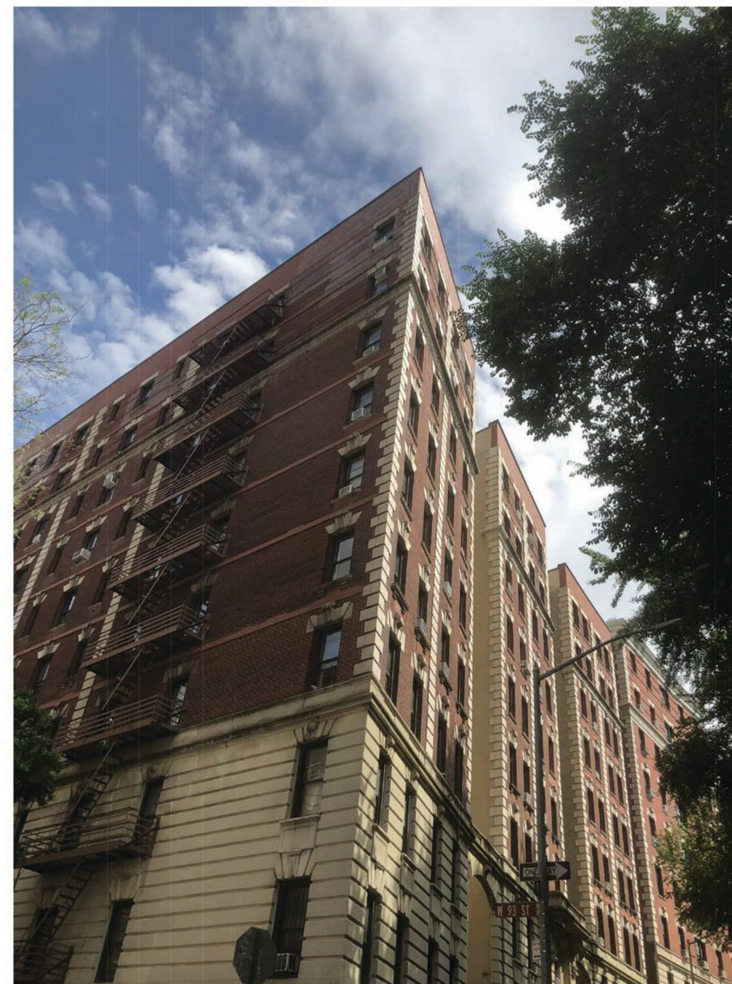
② VIEW OF 202 RSD LOOKING SOUTH FROM WEST 93RD ST NOT VISIBLE
