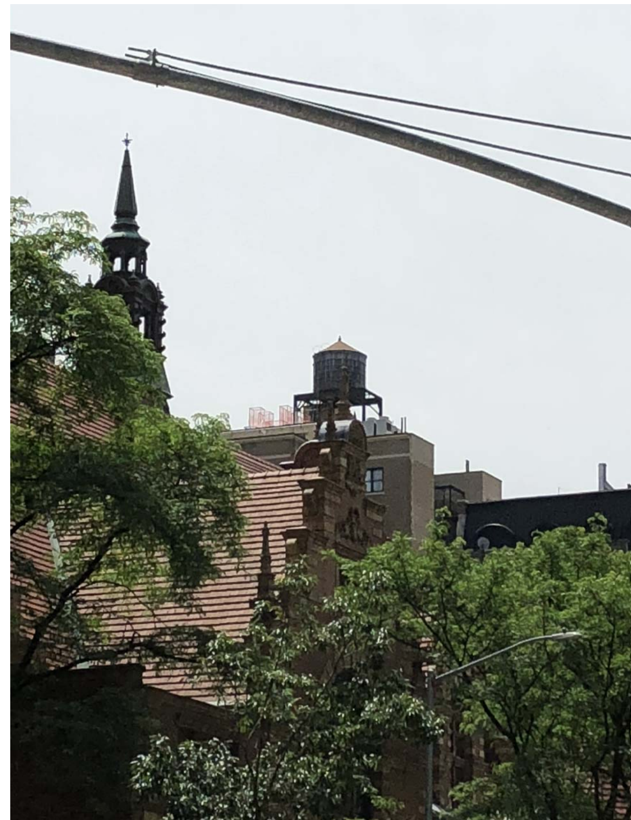
SOUTHWEST CORNER AT WESTEND AND 77TH STREET LOOKING SOUTH
