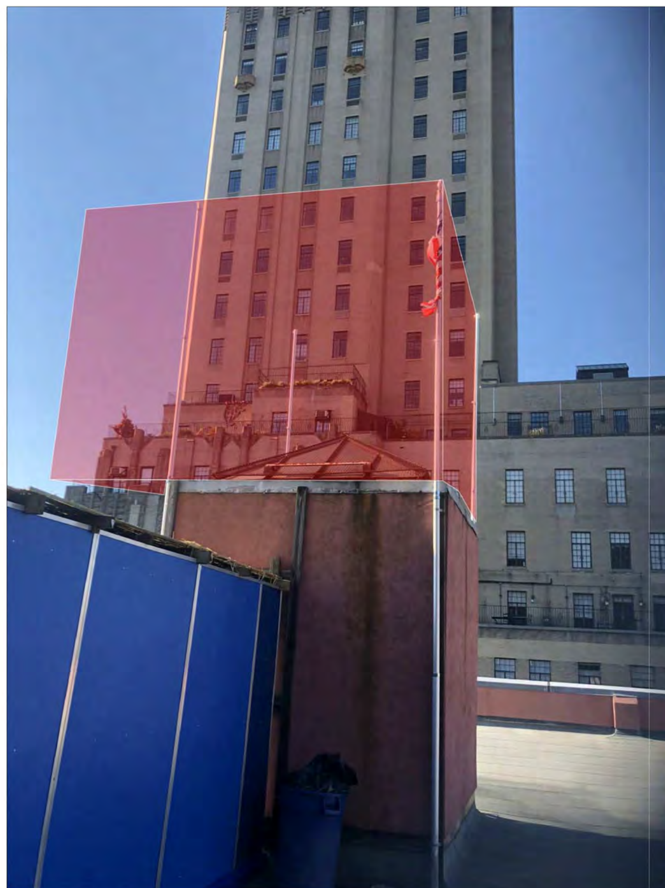
② AT ROOF SW PASSENGER ELEVATOR BULKHEAD & PROPOSED EXTENSION
