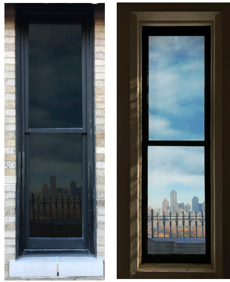
WINDOW 6 (Exterior & Interior)
