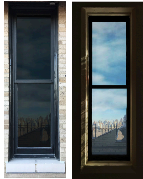
WINDOW 5 (Exterior & Interior)
