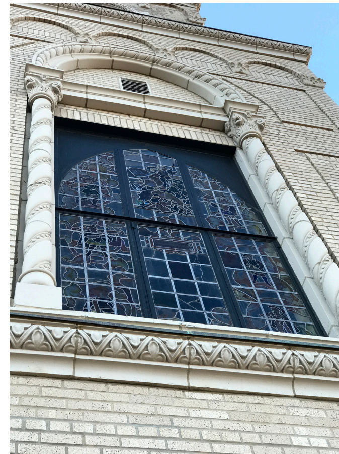
LPC PERMIT APPROVED (Exterior)
