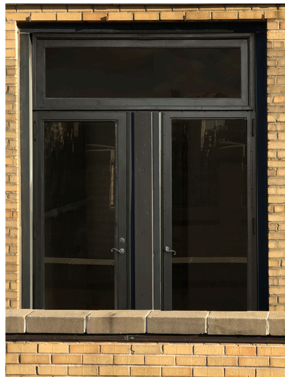
LPC PERMIT APPROVED (Exterior)
