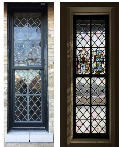
WINDOW 6 (Exterior & Interior)
