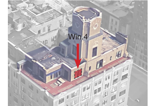
Window 4 on East Facade
