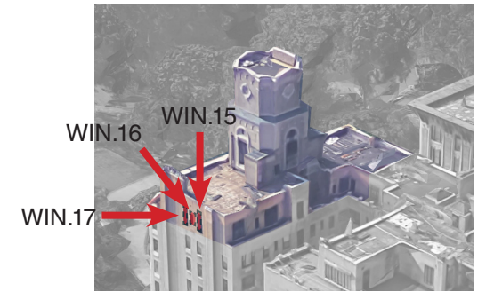
North & West Facade
