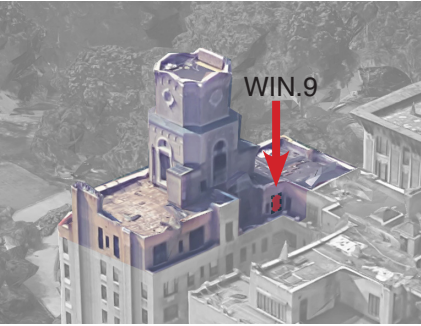
North & West Facade
