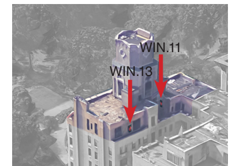
North & West Facade
