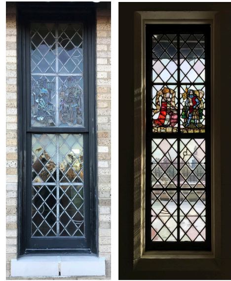
WINDOW 5 (Exterior & Interior)
