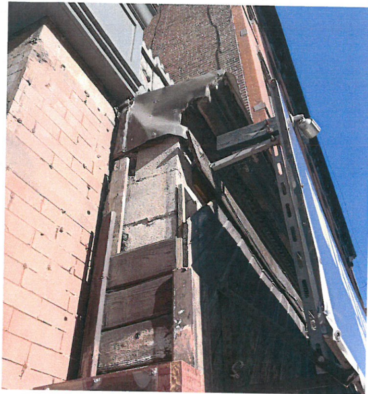
1 CMU WALL, WOOD CLADDING, AND CORNICE
