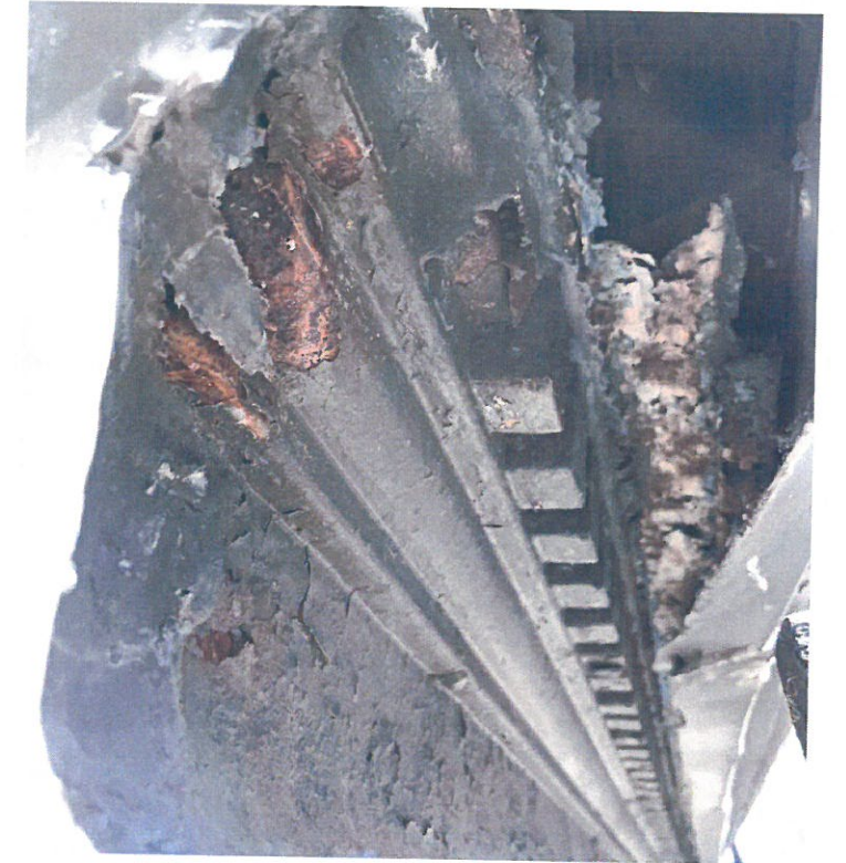
4 DETERIORATED CORNICE
