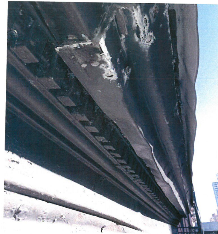
3 DENTIL BAND AND FLASHING
