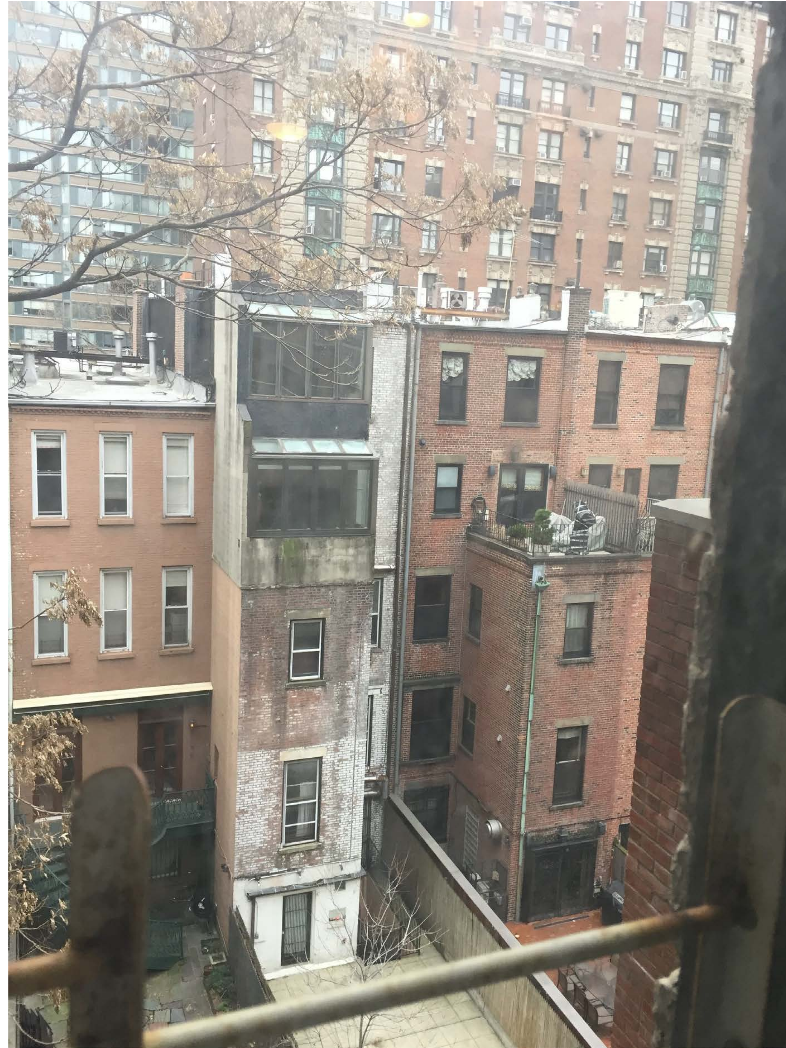
2 PHOTO FROM REAR ROOFTOP TO BUILDING BEHIND SCALE: NTS
