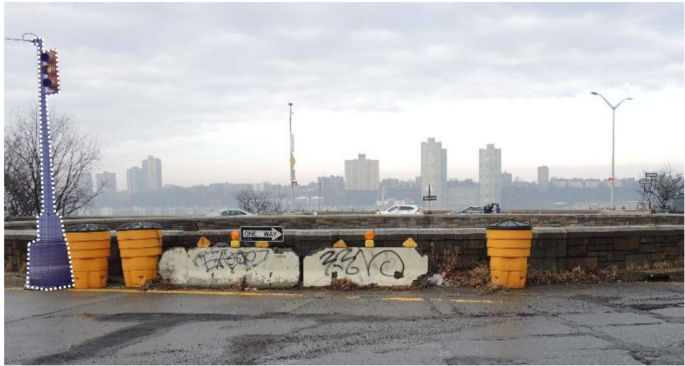
Existing Traffic Circle Light Post to be replaced with NYCDOT Historic Type F Luminaire
