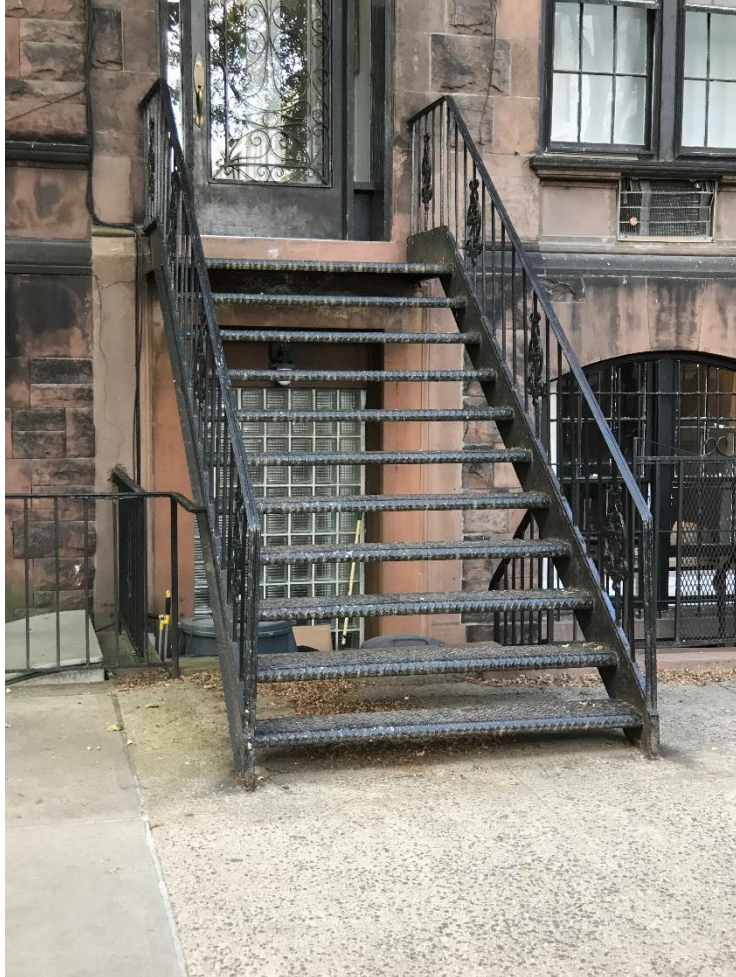
Metal staircase will be replicated in kind
