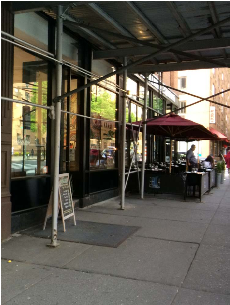
4 STOREFRONTS, LOOKING NORTH
