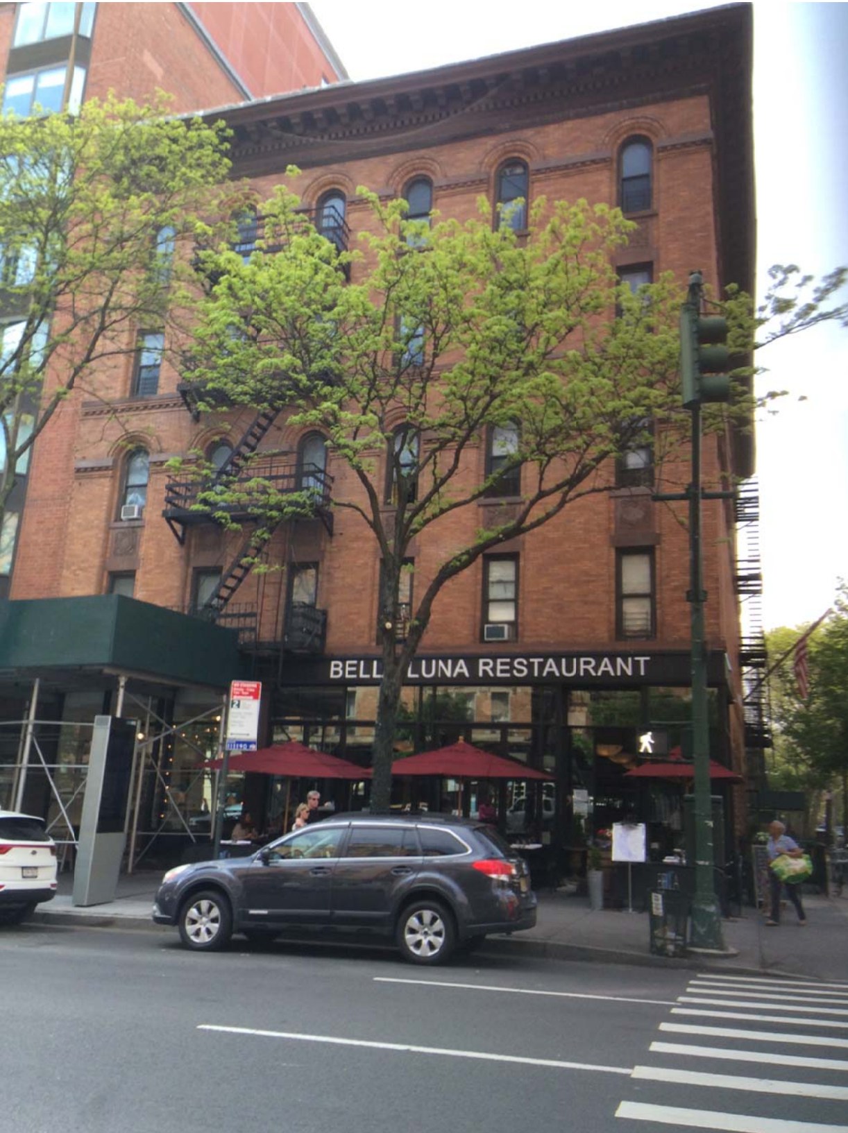
1 BUILDING PHOTO, FROM COLUMBUS AVENUE
