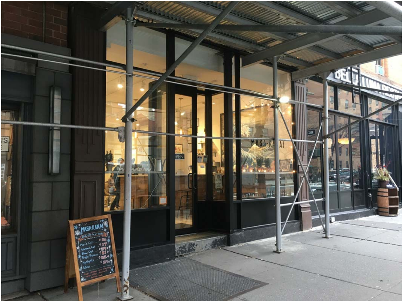
EXISTING MASA-KANAI STOREFRONT
