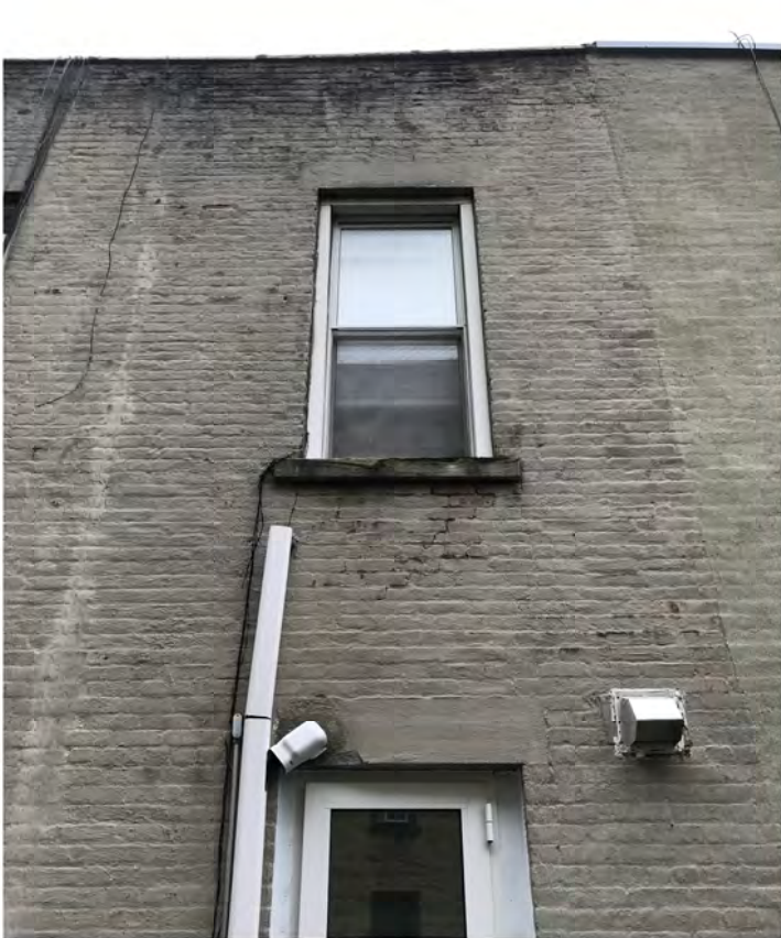
Existing 4th floor window to be replaced with door
