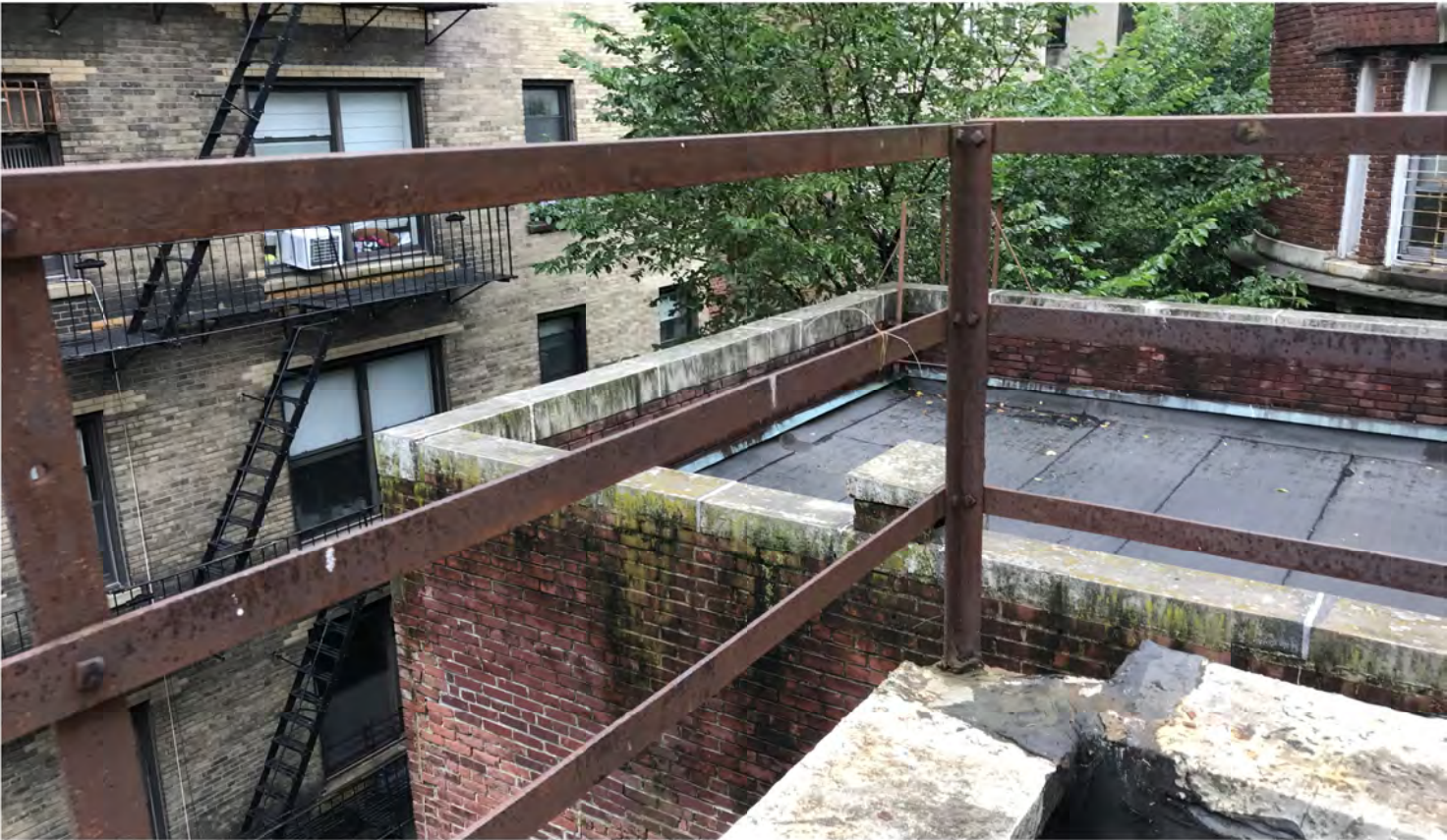
Existing roof guard rail to be replaced with steel guard rail (painted black)
