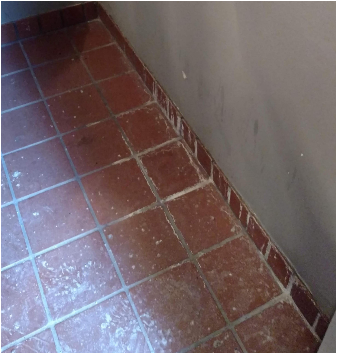
LACK OF VENTILATION AT THE GARDEN LEVEL VESTIBULE WITH NO ABILITY FOR WATER TO DRAIN CAUSES WALL, UNDER STAIR STRUCTURE AND PLASTER DAMAGE WITH VISIBLE EFFLORESCENCE DEPOSITS
