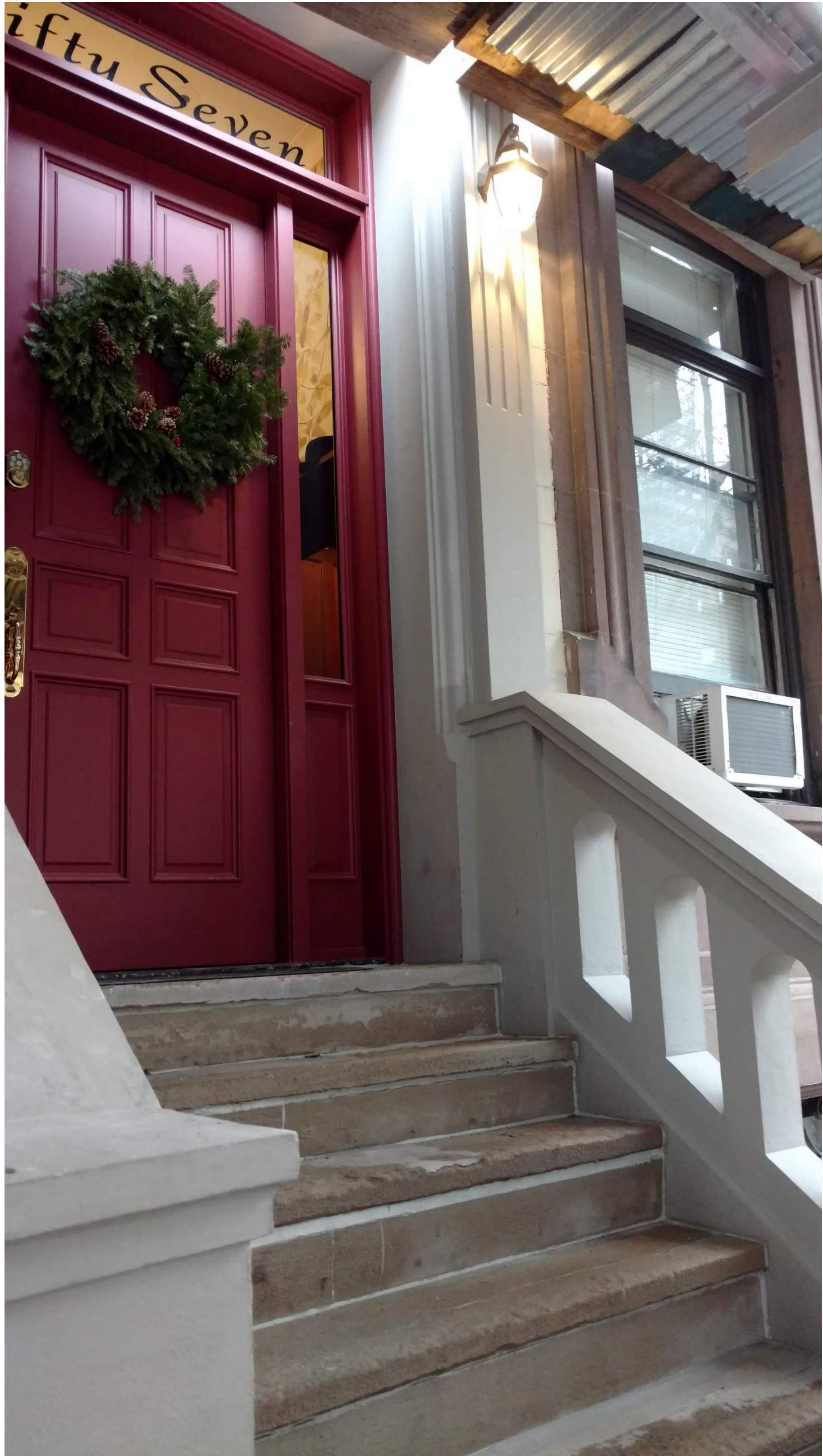
NO LANDING AT THE PARLOR MAIN ENTRANCE DOOR IS POSING SAFETY, TRIPPING HAZARDS
