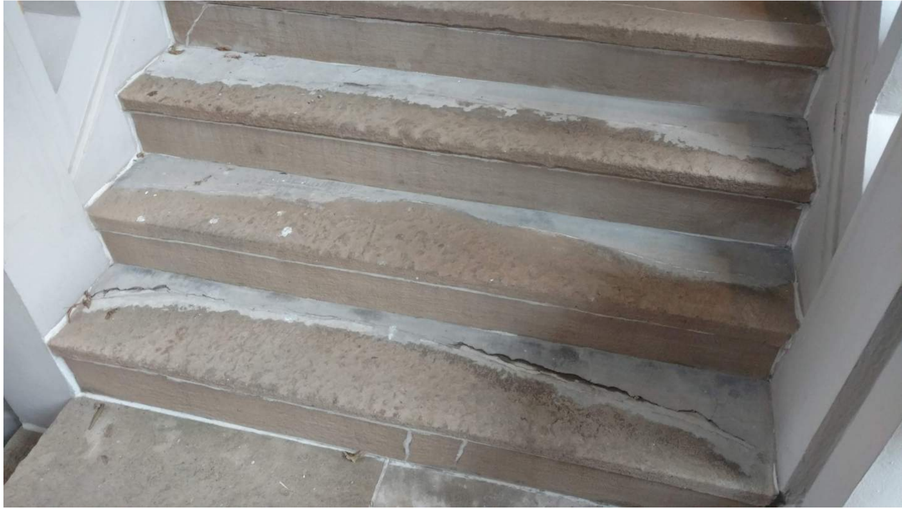
WATER PENETRATING INTO THE STAIRS IS UNDERMINING THE STRUCTURE OF THE STOOP THROUGH THE FREEZE/THAW CYCLE
