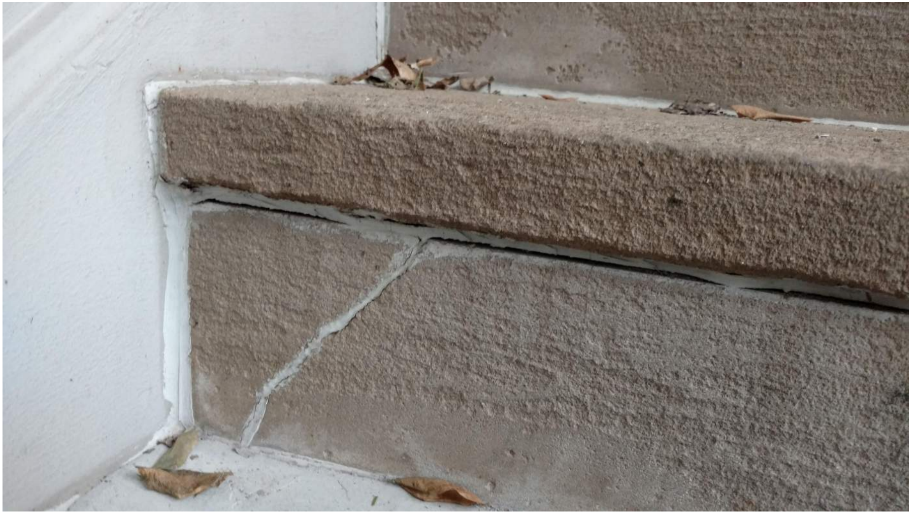
WATER PENETRATING INTO THE STONE THREADS AND RISERS IS SPALLING THE STONE SURFACE
