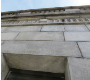
EXISTING CONDITIONS OF EXTERIOR GRANITE (SOILING AND CRACKING)
