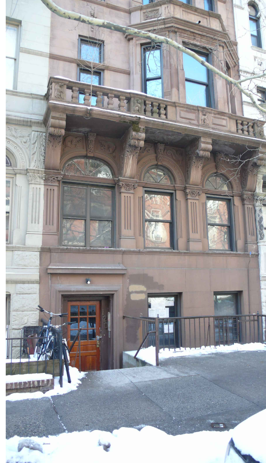
PHOTO @ 120 W 74TH STREET
