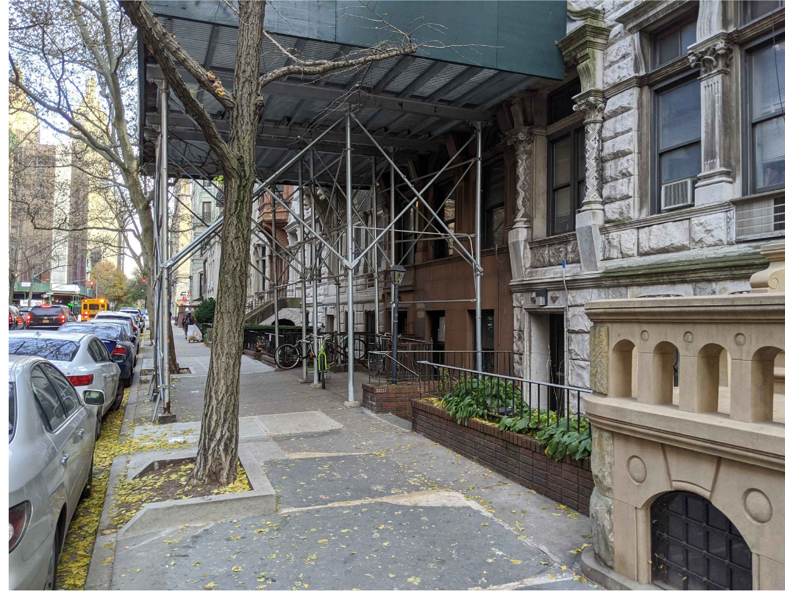
PHOTO @ 122 W 74TH STREET
