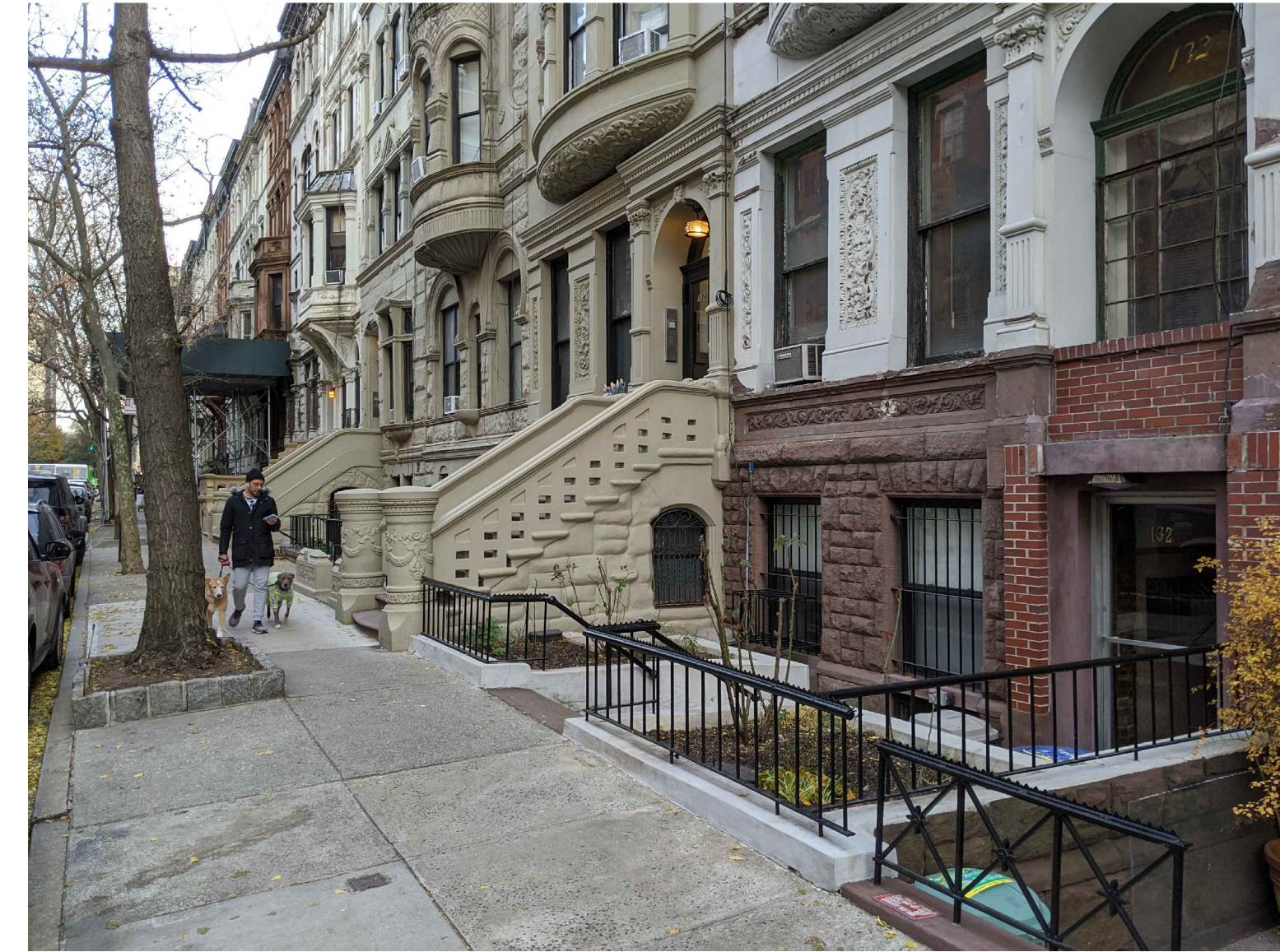
PHOTO @ 132 W 74TH STREET
