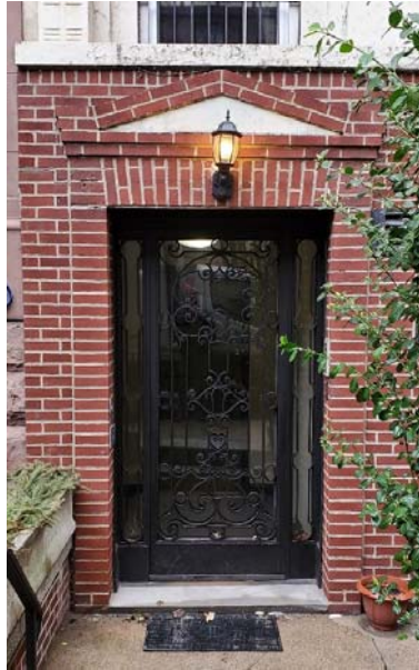
Re-purposed original metal and glass single leaf entry door from 309 West 90 th Street. Currently installed on basement level
