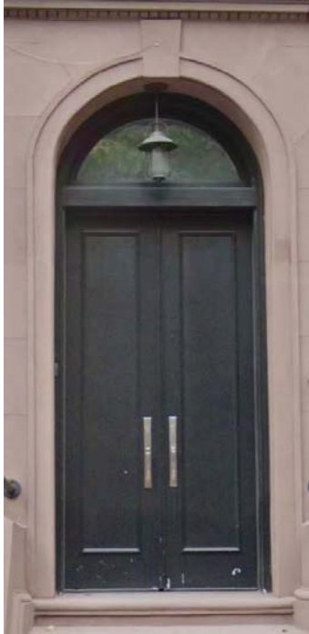
Existing Main Entry Door, Installed around 2008
