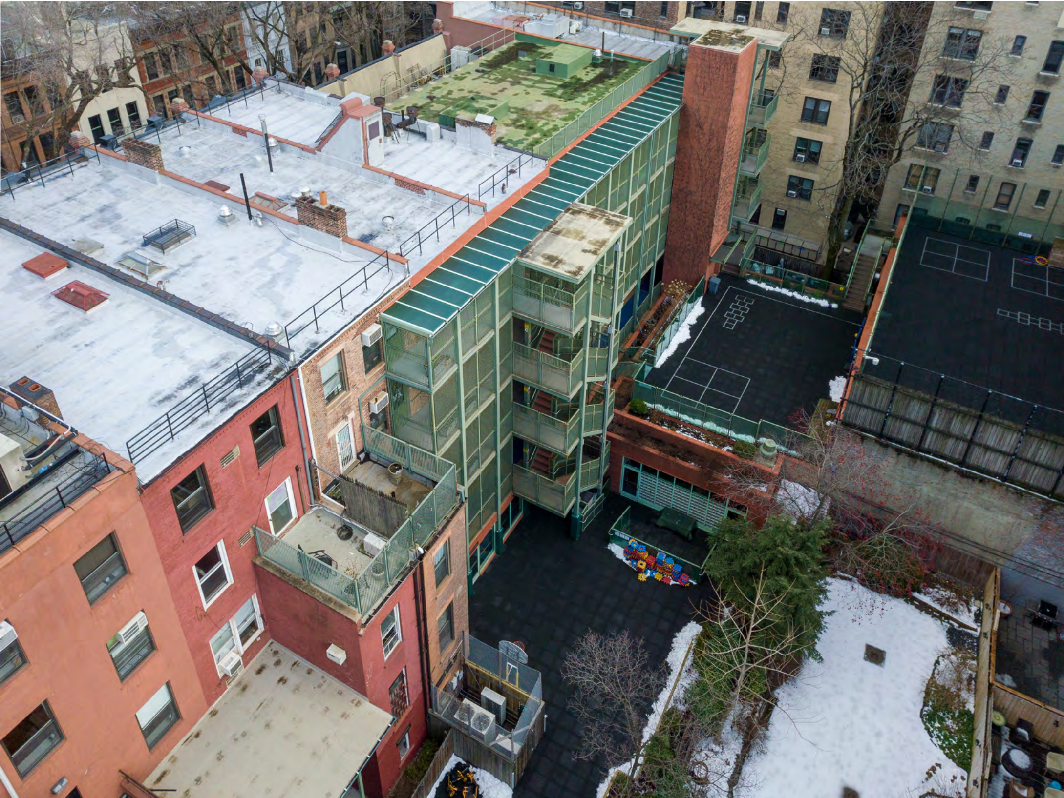
VIEW 04 - NEIGHBORING REAR FACADES
