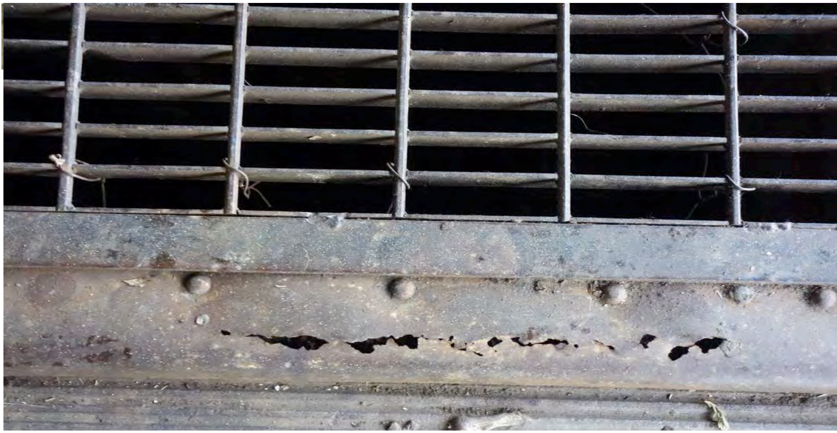
16 DETAIL VIEW OF VAULT DECKING IN POOR CONDITION
