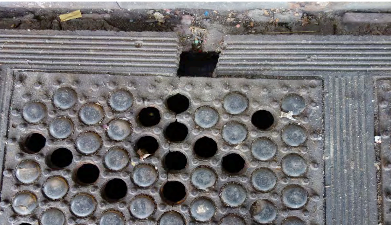
15 DETAIL VIEW OF VAULT DECKING IN POOR CONDITION
