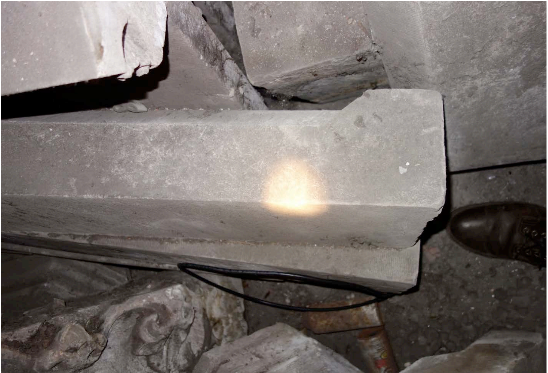
10 COMPONENTS OF FORMER STONE GUARDRAIL at INTERIOR HISTORIC FABRIC
