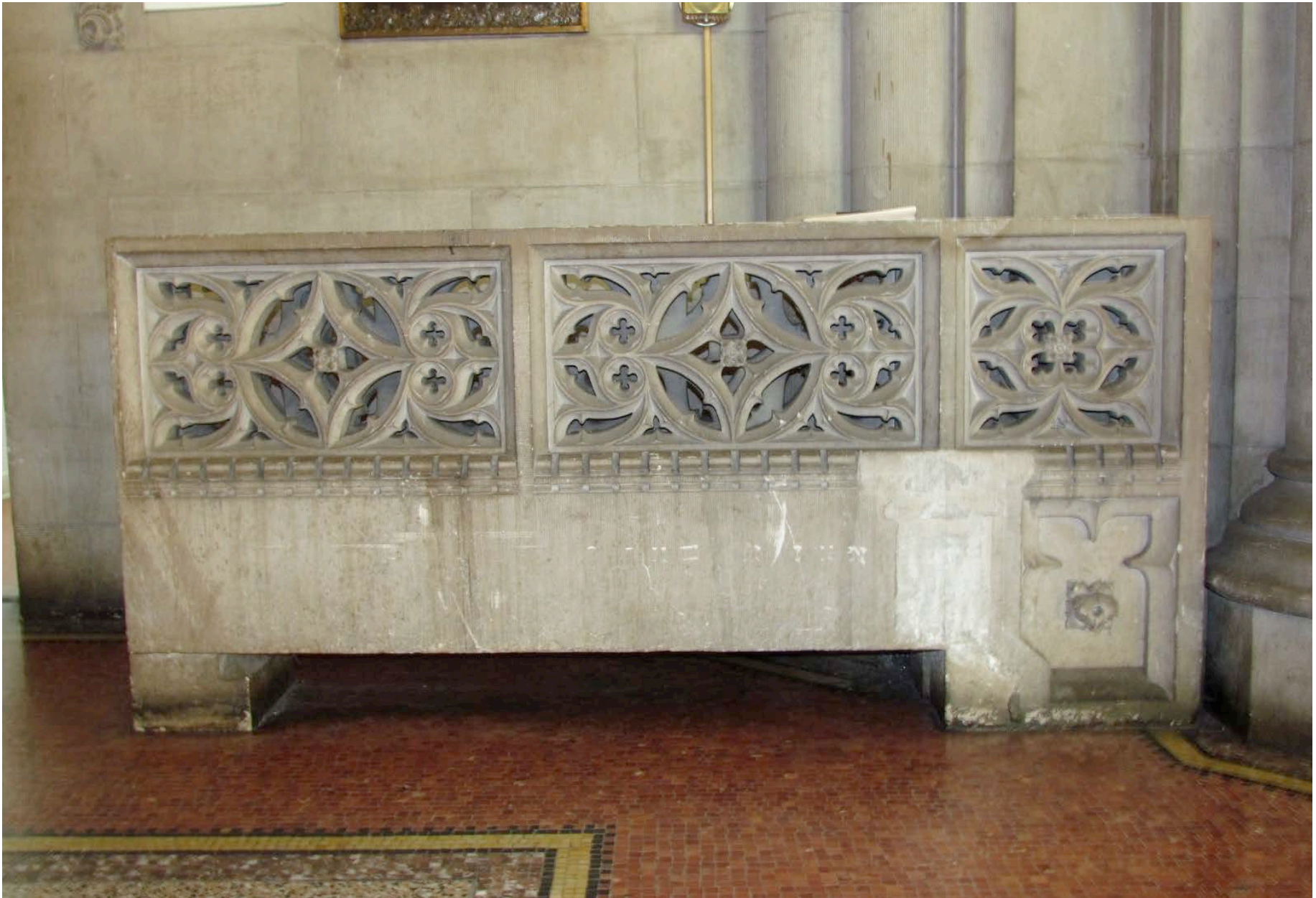
12 SALVAGE STONE GUARDRAIL (Two Units) FOR REUSE INTERIOR
