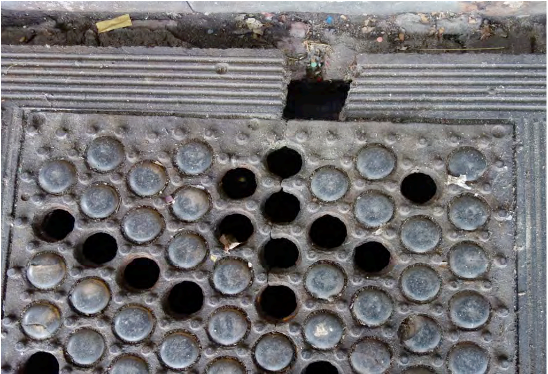
15 DETAIL VIEW OF VAULT DECKING IN POOR CONDITION CENTRAL PARK WEST FACADE
