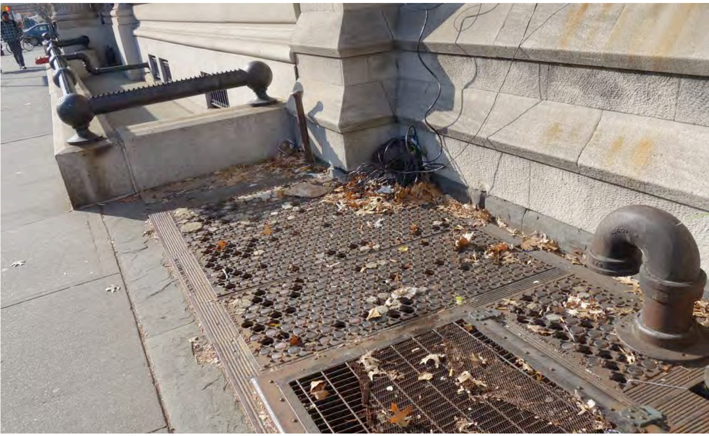
13 EXISTING MECHANICAL VAULT IN POOR CONDITION SOUTH SIDE OF CENTRAL PARK WEST
