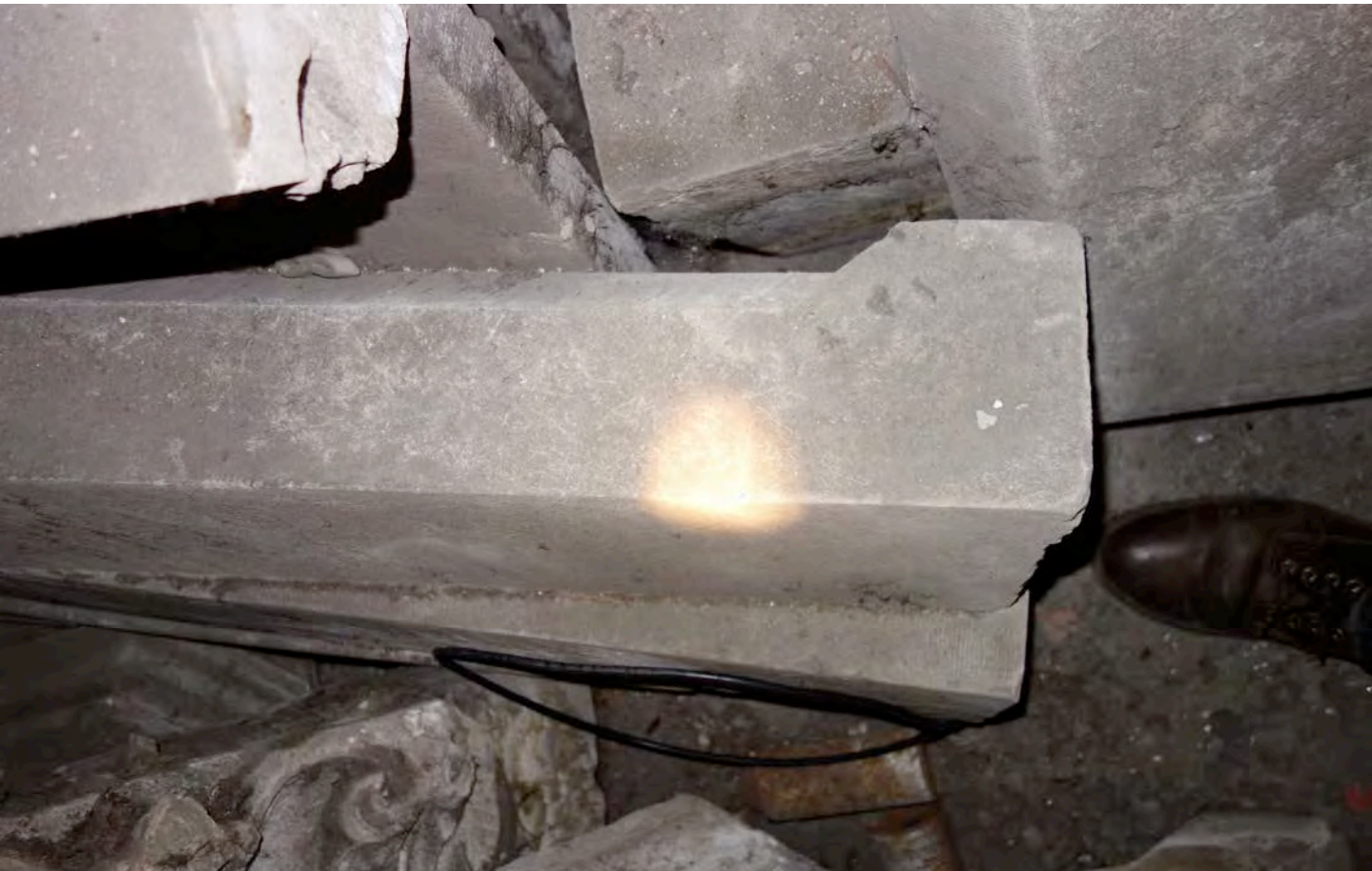
10 COMPONENTS OF FORMER STONE GUARDRAIL AT INTERIOR HISTORIC FABRIC
