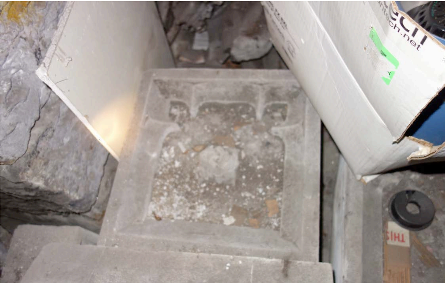
9 COMPONENTS OF FORMER STONE GUARDRAIL AT INTERIOR HISTORIC FABRIC
