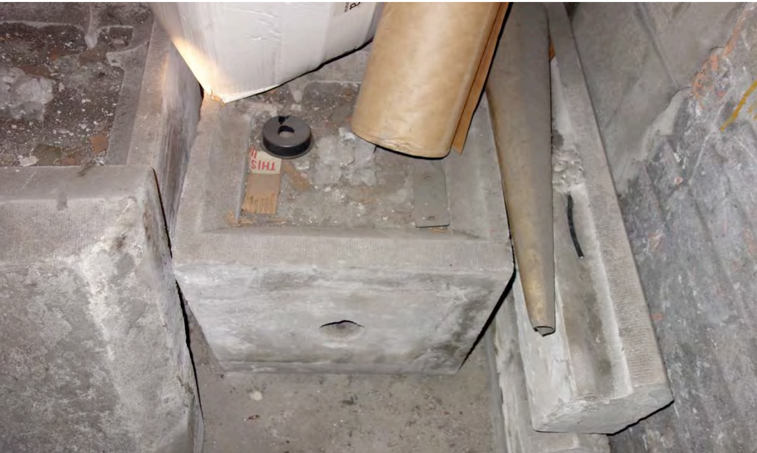
11 COMPONENTS OF FORMER STONE GUARDRAIL AT INTERIOR HISTORIC FABRIC
