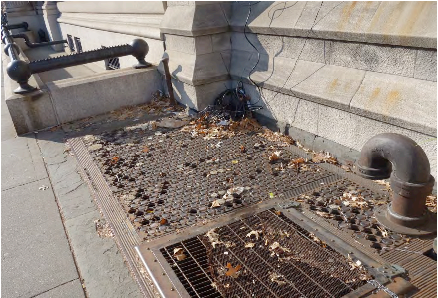
13 EXISTING MECHANICAL VAULT IN POOR CONDITION CENTRAL PARK WEST FACADE LOOKING SOUTH
