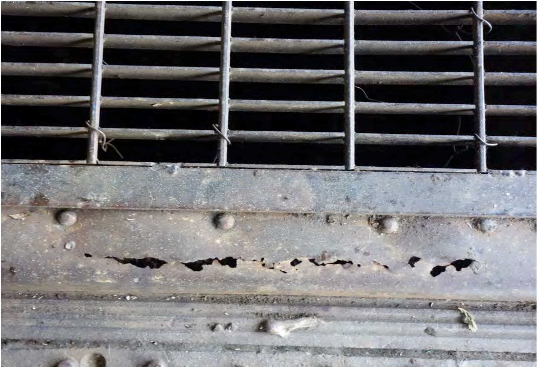
16 DETAIL VIEW OF VAULT DECKING IN POOR CONDITION CENTRAL PARK WEST FACADE
