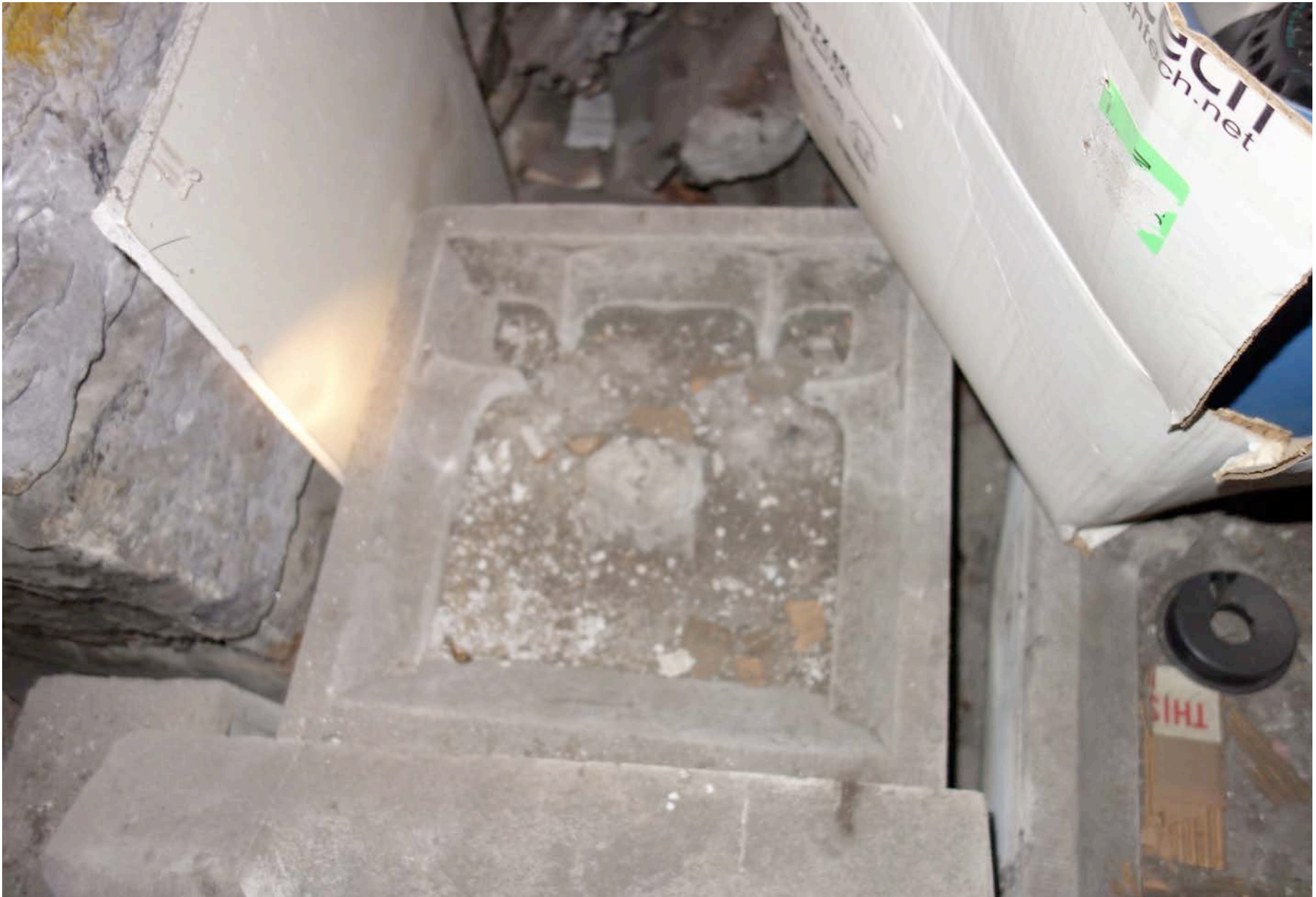
9 COMPONENTS OF FORMER STONE GUARDRAIL at INTERIOR HISTORIC FABRIC
