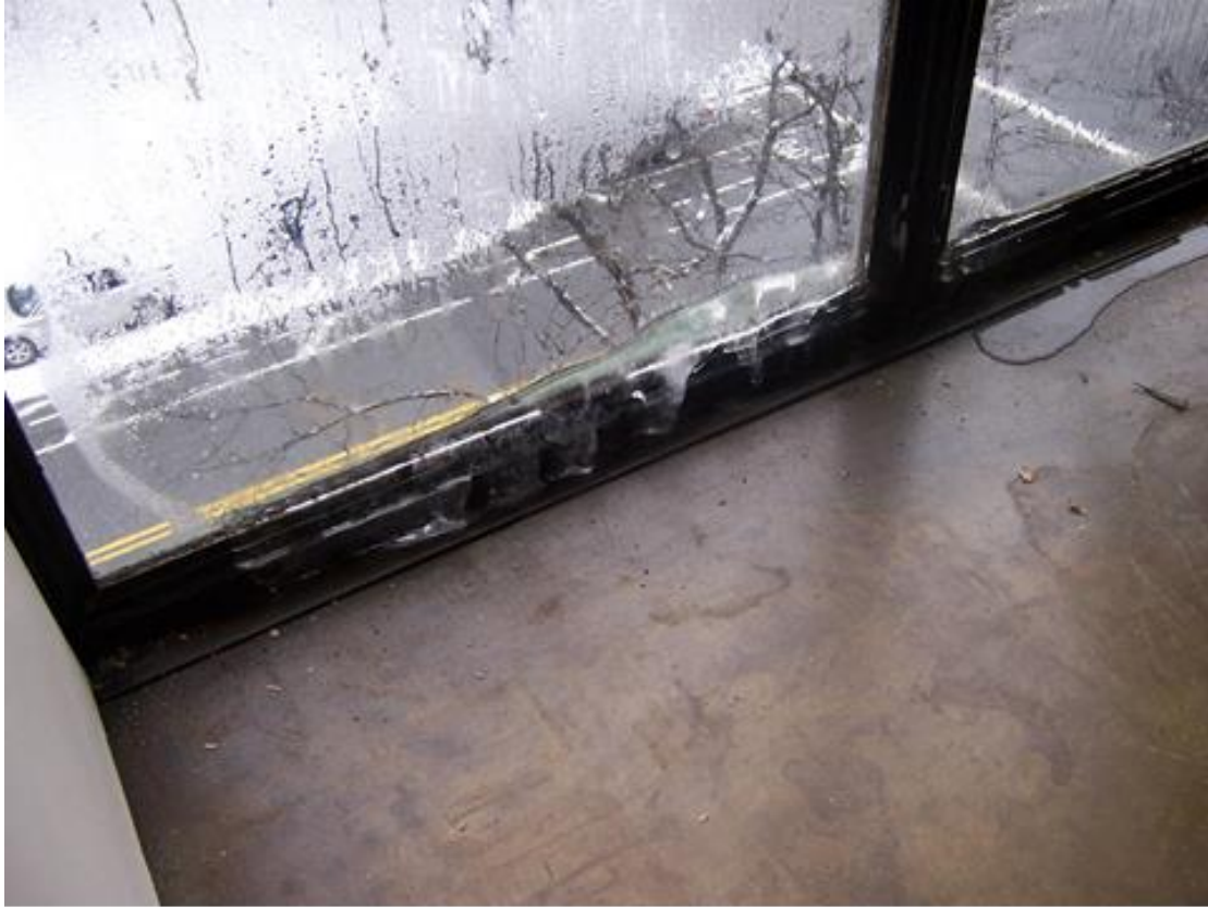
Condensation, ice and water pooling.
