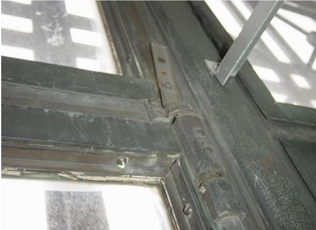
Damaged hardware, signs of water run-off, deteriorated putty and pitting.
