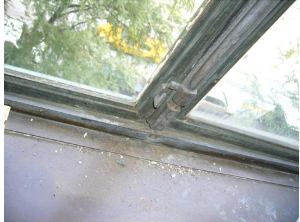
Deteriorated putty. Oxidation not allowing proper closing and locking.
