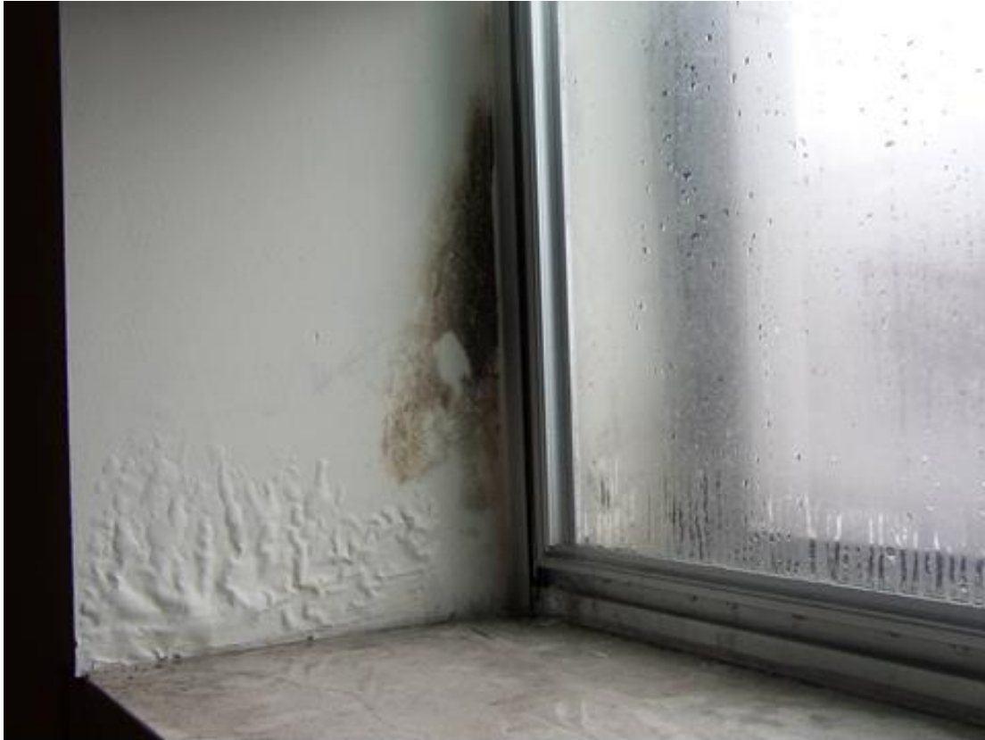
Finish damage and mold at interior storm window.
