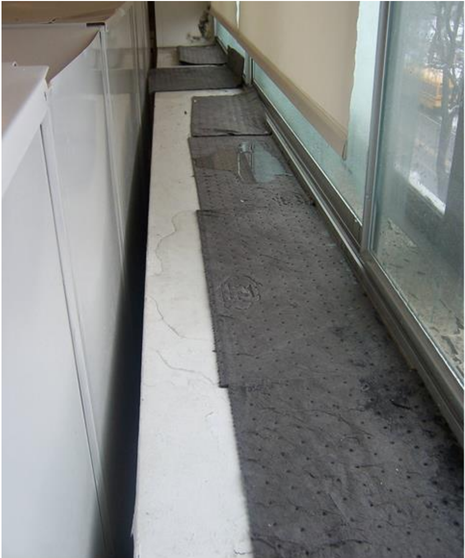
Water pooling and mold at existing interior storm window.
