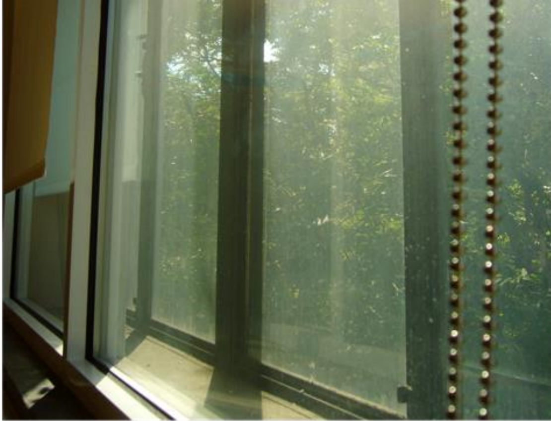
One type of existing interior storm window.
