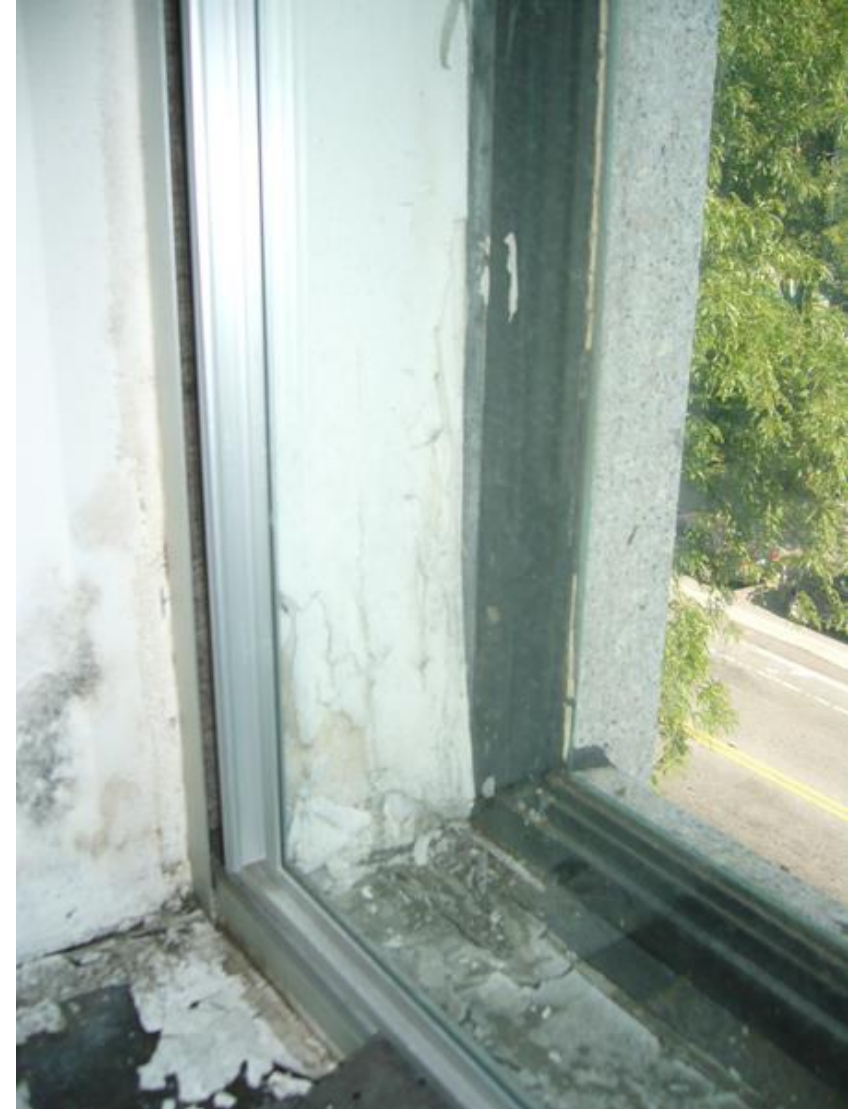
Finish damage and mold at interior storm window.
