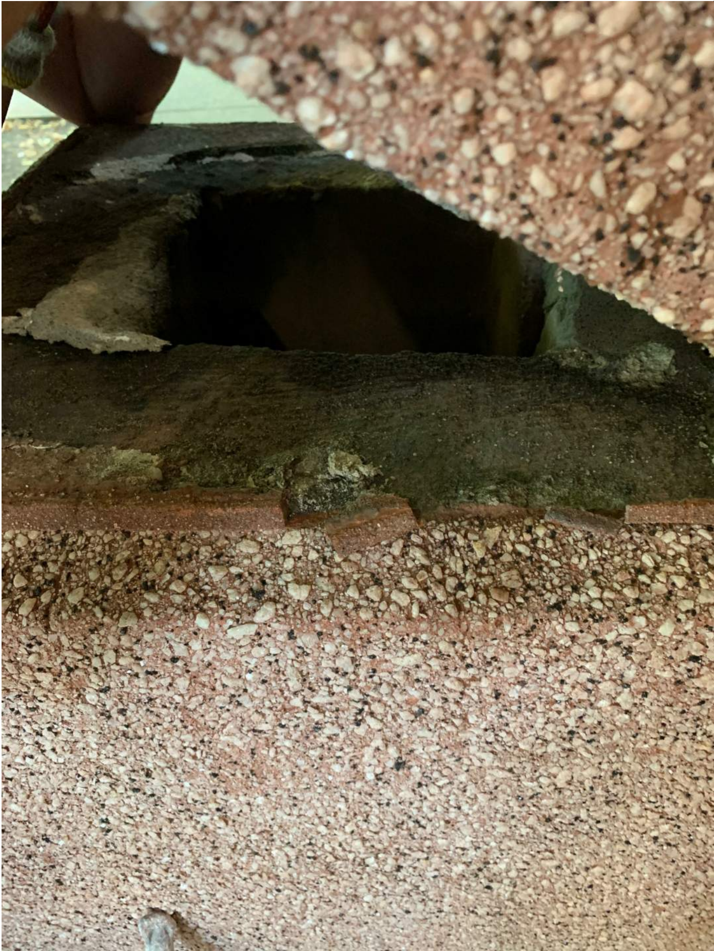
E1 PIER PROBE - LIFTED TOP OF PIER
