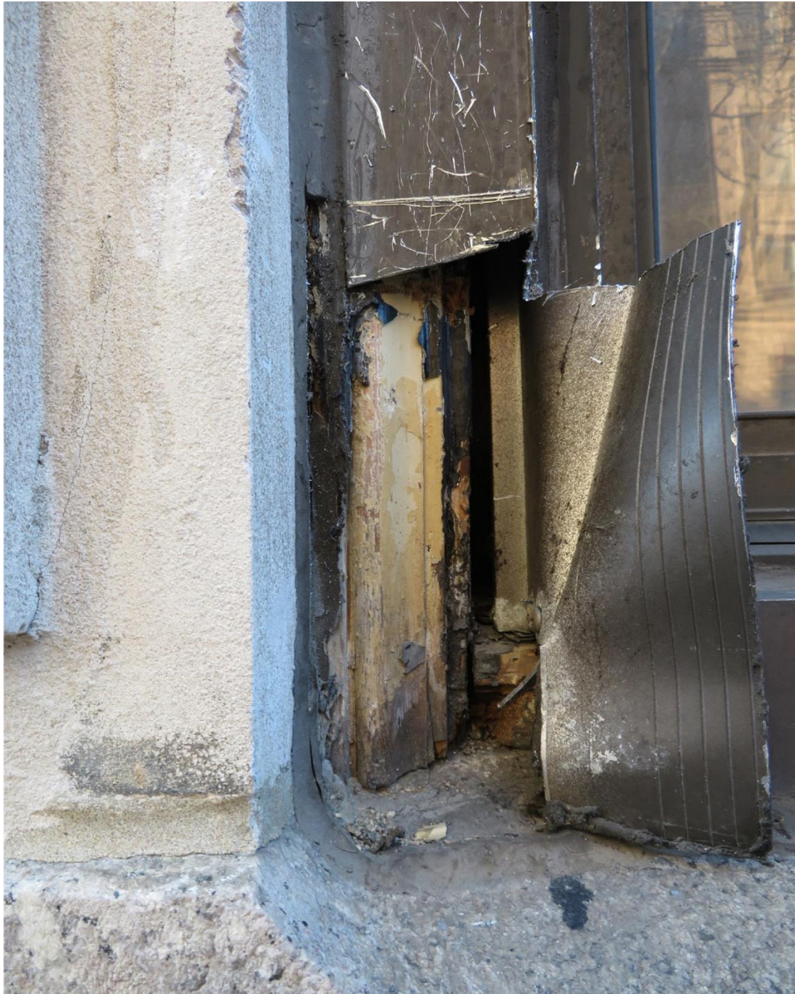
Probe at West 87th Street showing original brick mold
