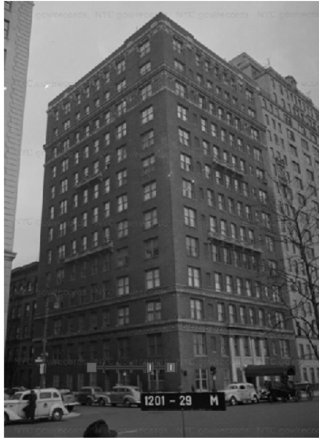
271 Central Park West (at West 87th Street) Schwartz & Gross, 1912-13 NYC Municipal Archives ca. 1940s Tax Photo
