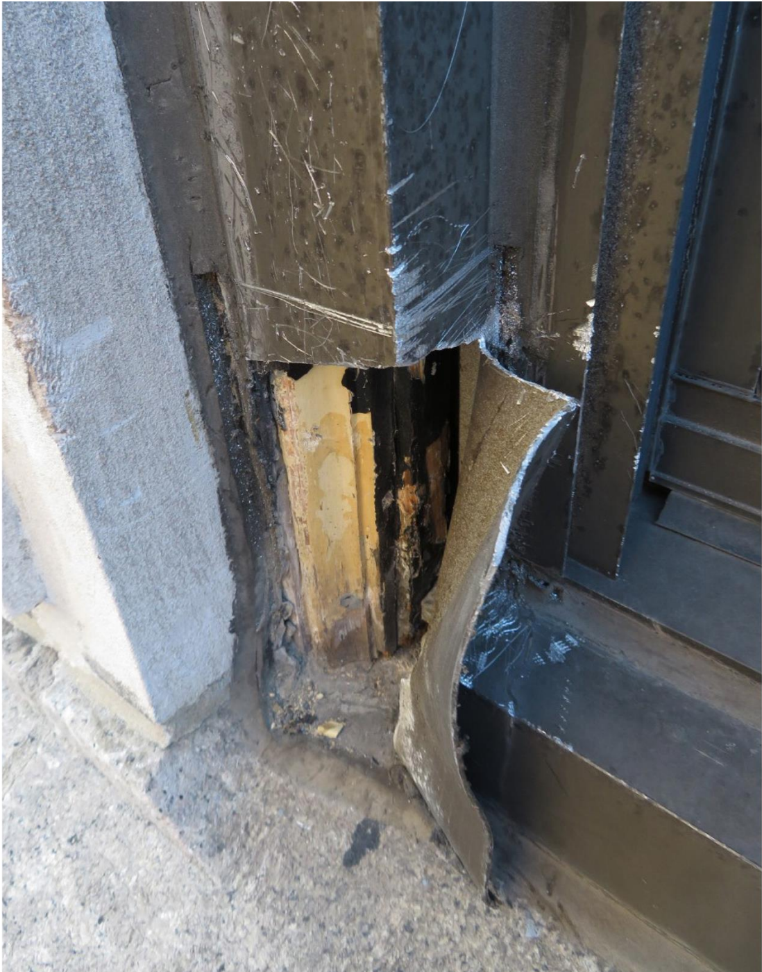
Probe at West 87th Street showing original brick mold
