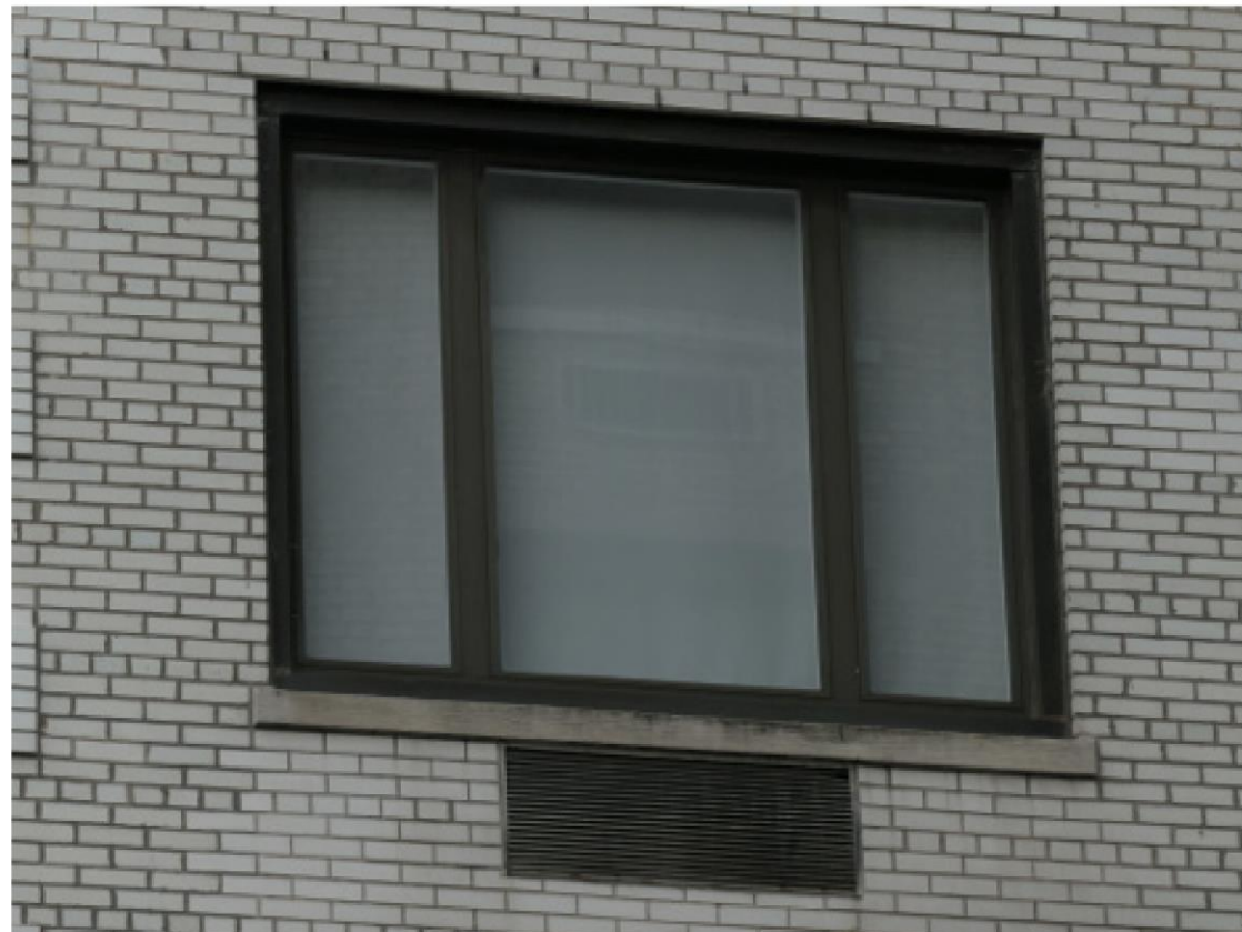
Photos showing the variation in triple-gang windows across the facades. The mullion thicknesses, spacing and projections vary significantly. The result is a loss of articulation in these large window openings.
