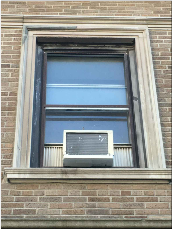
2 TYPICAL DOUBLE HUNG WINDOW (PRIMARY FACADE) SCALE: 1" = 1'-0" • One-over-one double hung windows with black frame typical throughout visible facades. • Aluminum window frame with perimeter aluminum panning
