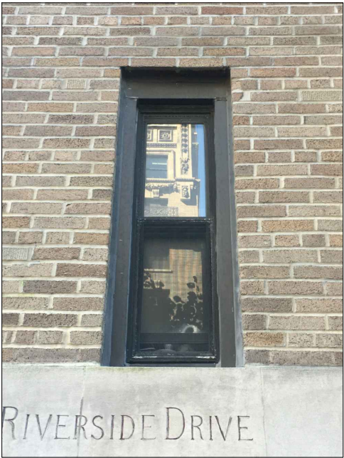
3 TYPICAL DOUBLE HUNG WINDOW (PRIMARY FACADE) SCALE: 1" = 1'-0" • One-over-one double hung windows with black frame typical throughout visible facades. • Aluminum window frame with perimeter aluminum panning
