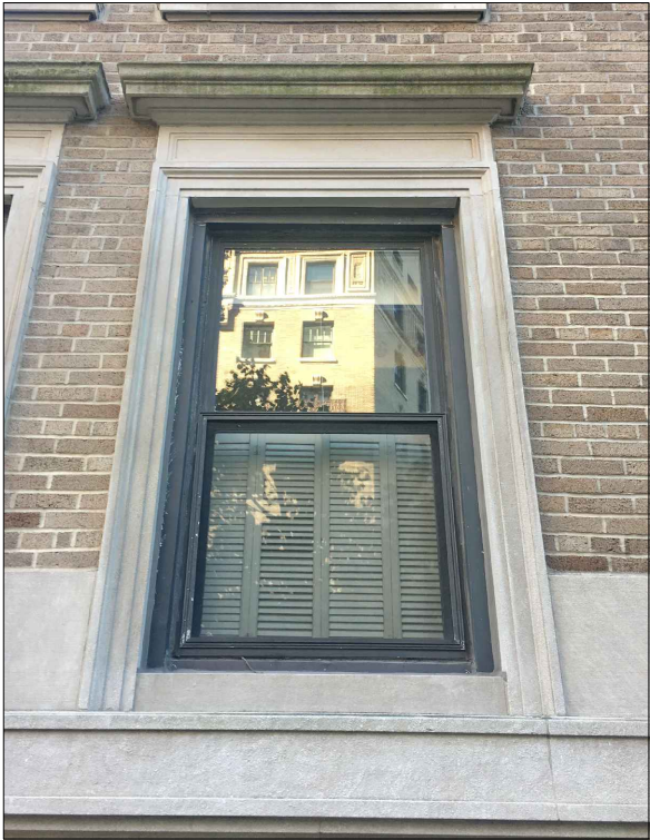
1 TYPICAL DOUBLE HUNG WINDOW (PRIMARY FACADE) SCALE: 1" = 1'-0" • One-over-one double hung windows with black frame typical throughout visible facades. • Aluminum window frame with perimeter aluminum panning
