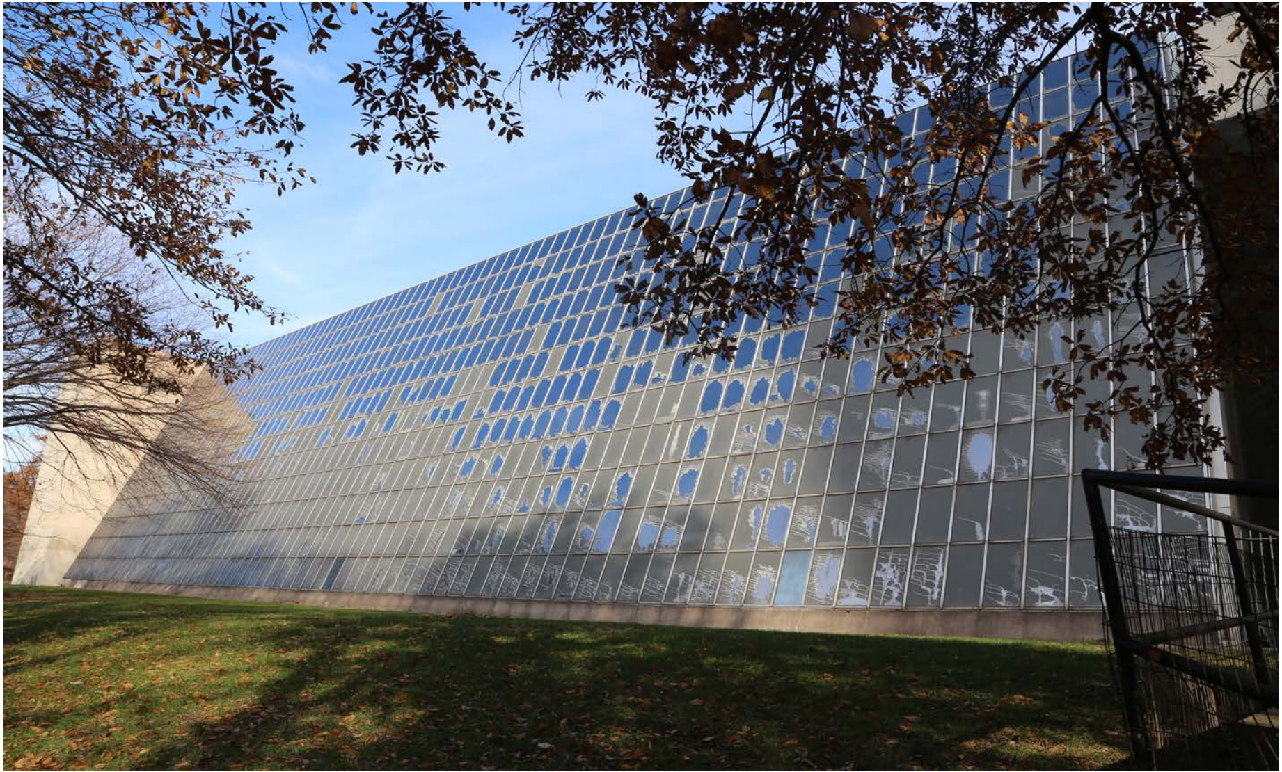
Existing Condition View from South of Rockefeller Sloped Glazing Sloped glazing is 200 feet long, 60 feet high and at a 70 degree slope with a surface area of approximately 12,000 square feet.
