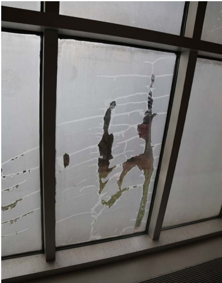
Interior detail of with deteriorating plastic film
