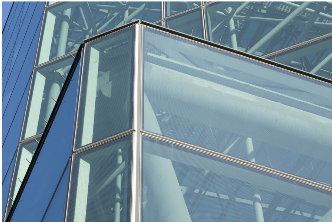
PRECEDENT: EXAMPLE OF FRITTED BIRD FRIENDLY GLASS AND ITS VISIBILITY FROM A DISTANCE: RENOVATION OF JACOB JAVITS CONVENTION CENTER
