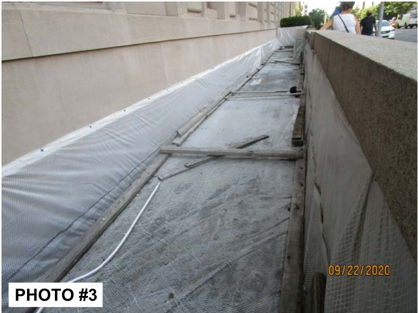
3 | VIEW OF THE TEMPORARY PROTECTION INSTALLED OVER AREAWAY WATERPROOFING VIDARIS PHOTO, SEPTEMBER 2020
