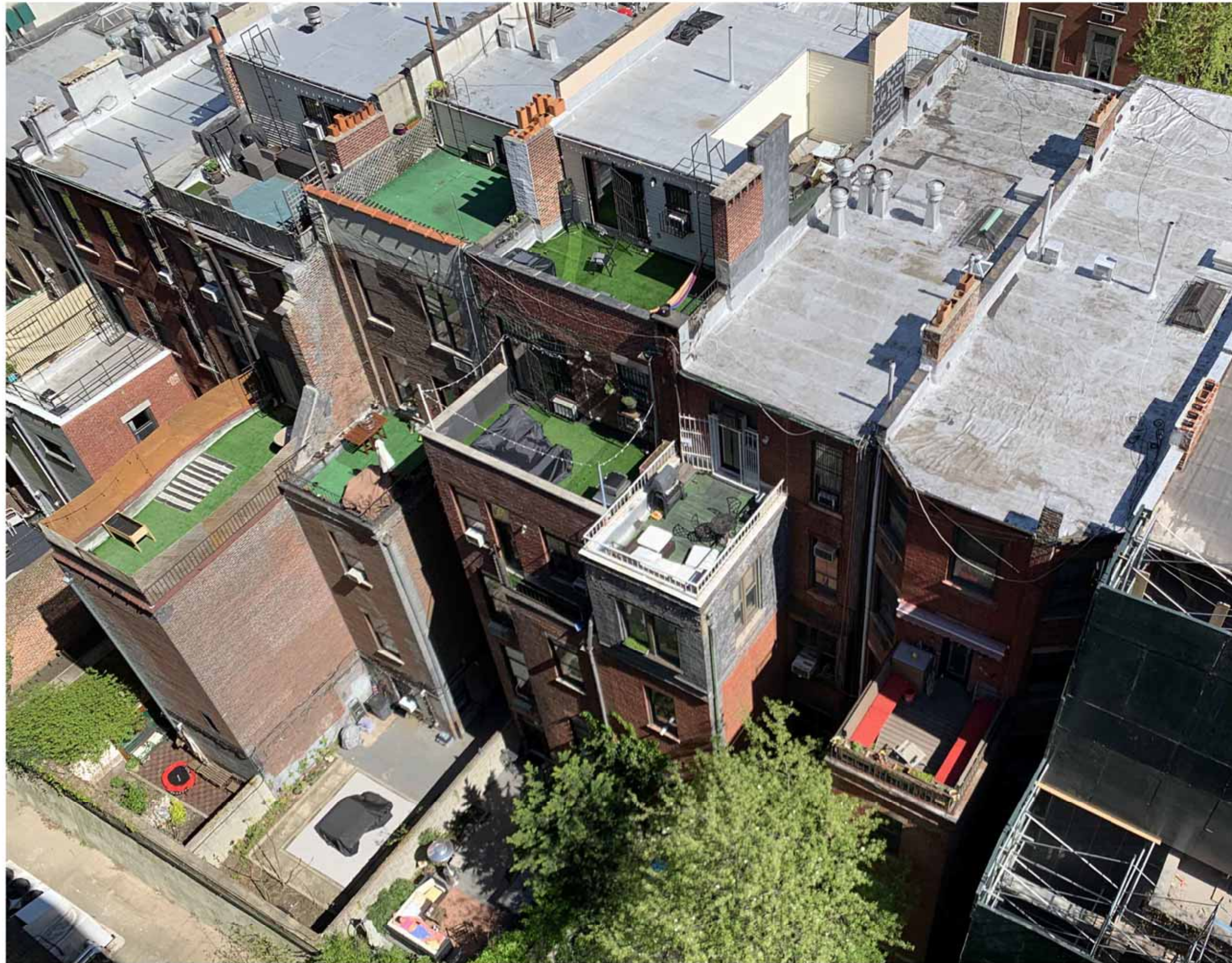
132-120 W 74TH ST REAR PARAPETS
