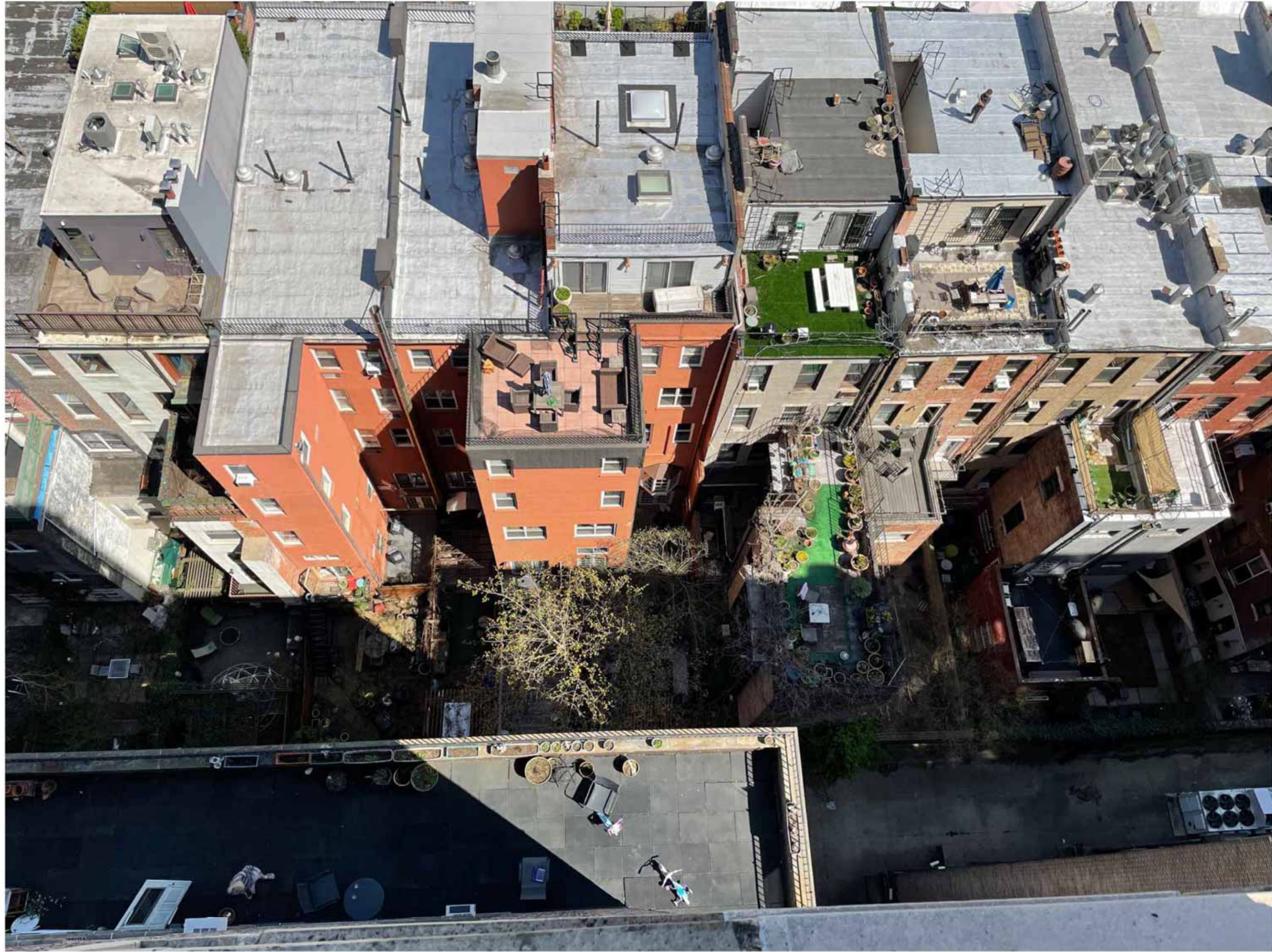
140-144 W 74TH ST REAR FACADE
