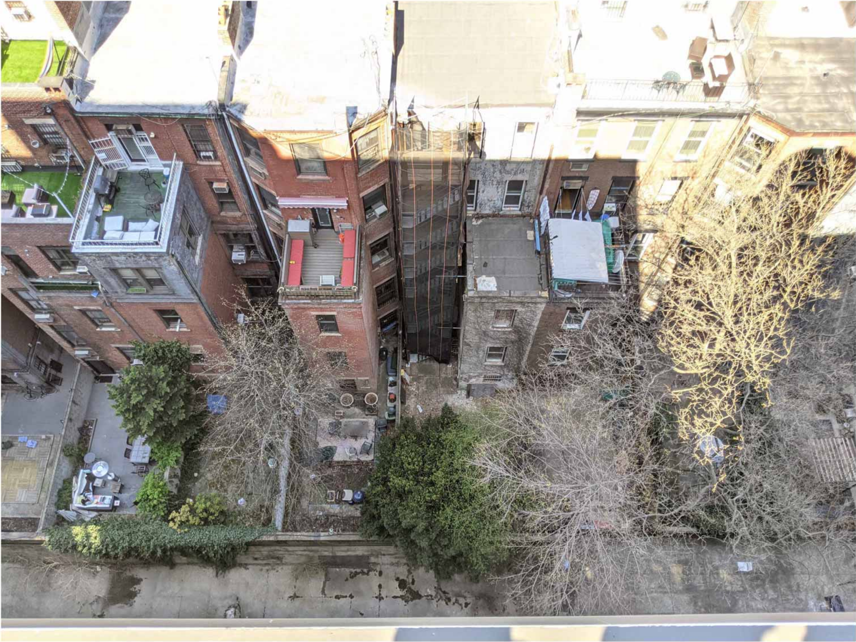
120 W 74TH ST REAR FACADE
