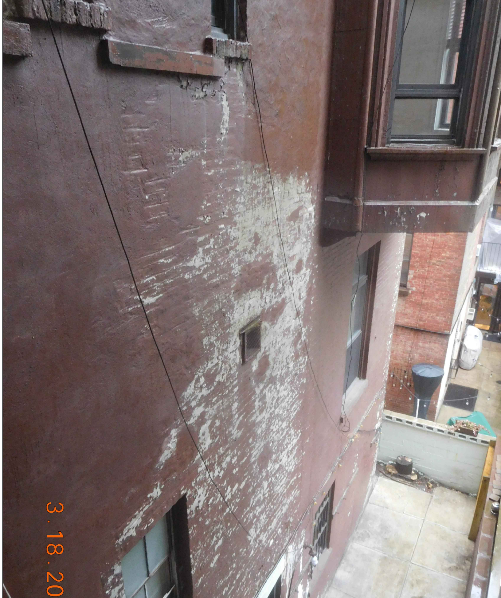
PHOTOS OF REAR EXTENSION TO BE REMOVED SHOWING POOR CONDITION OF EXISTING MASONRY
