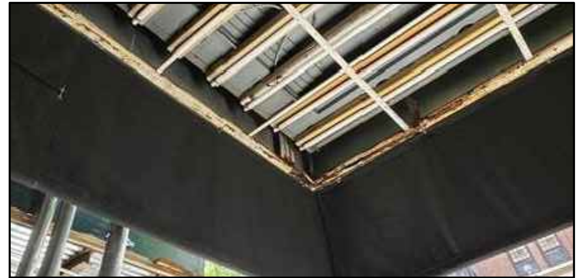
EXISTING FABRIC BELOW MARQUEE AT CORNER
