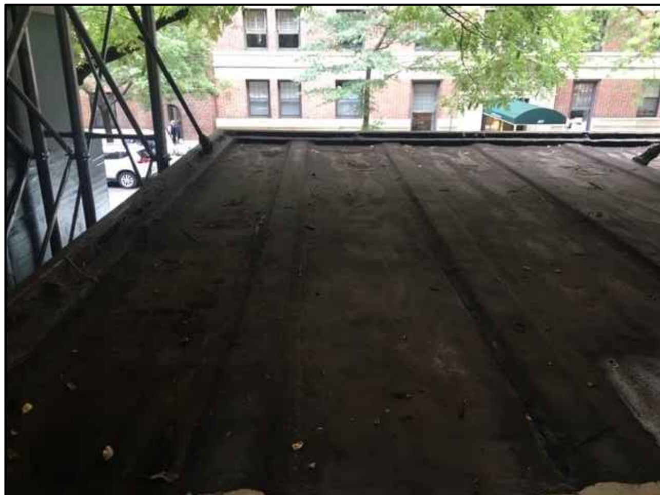
EXISTING AWNING FROM ABOVE
