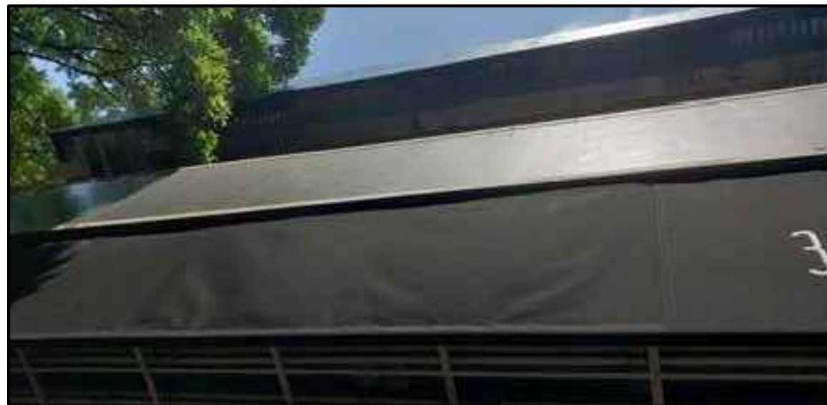
EXISTING FABRIC BELOW MARQUEE FROM STREET
