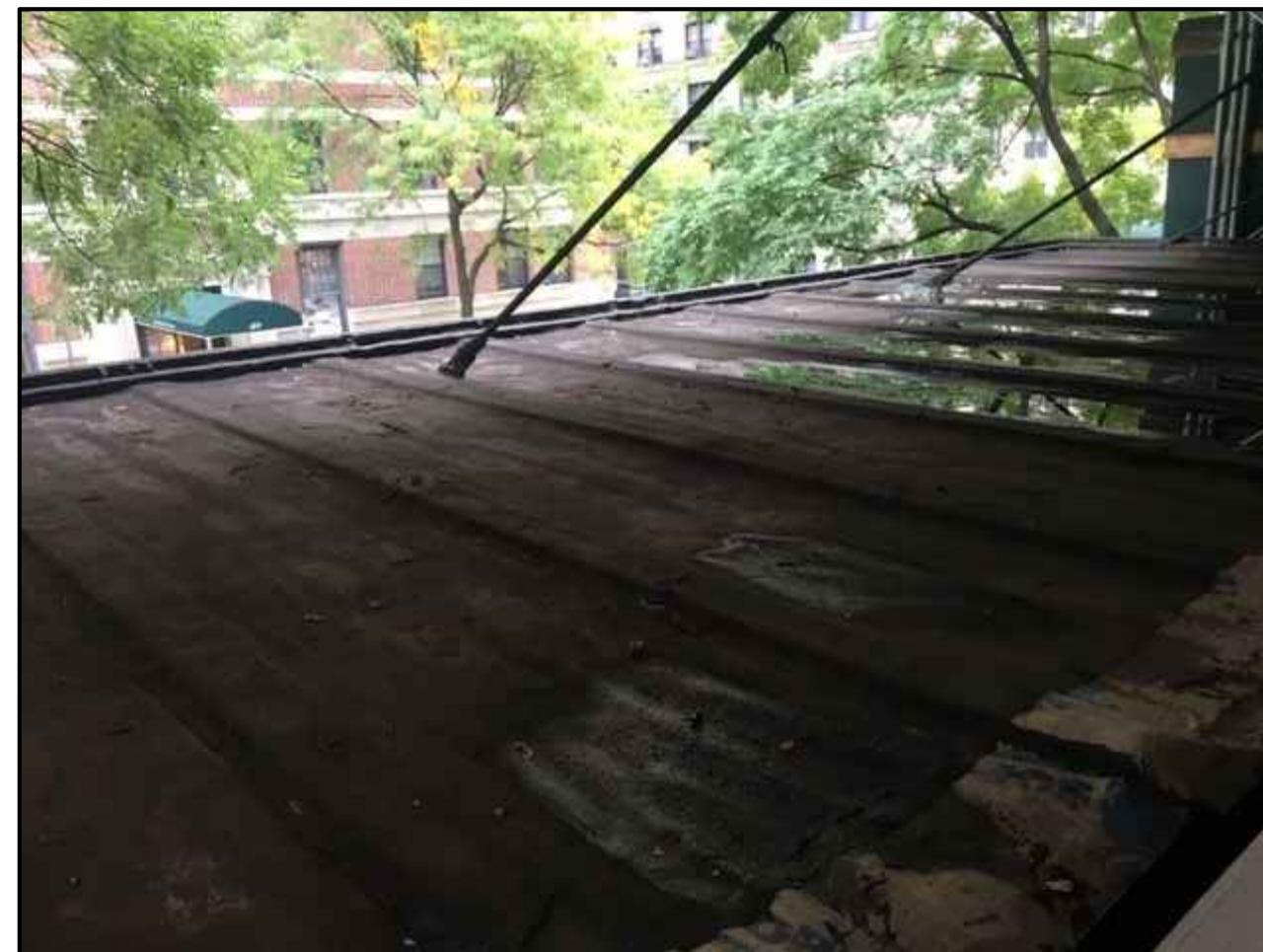
EXISTING AWNING FROM ABOVE
