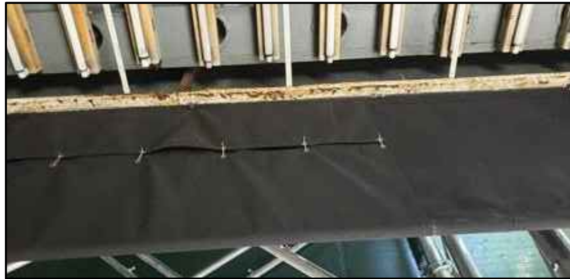
EXISTING FABRIC BELOW MARQUEE
