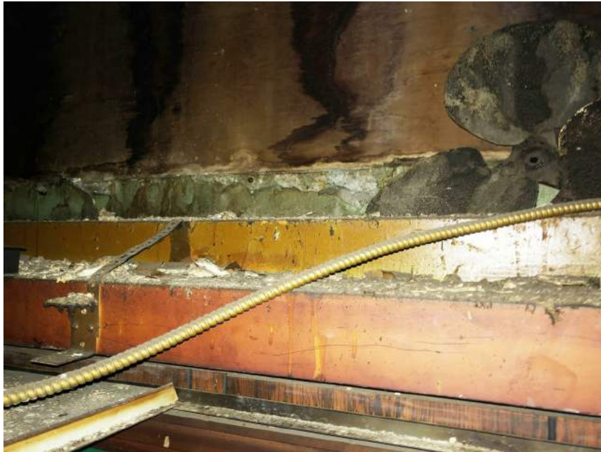
PROBE AT PLYWOOD INFILLED HISTORIC STOREFRONT
