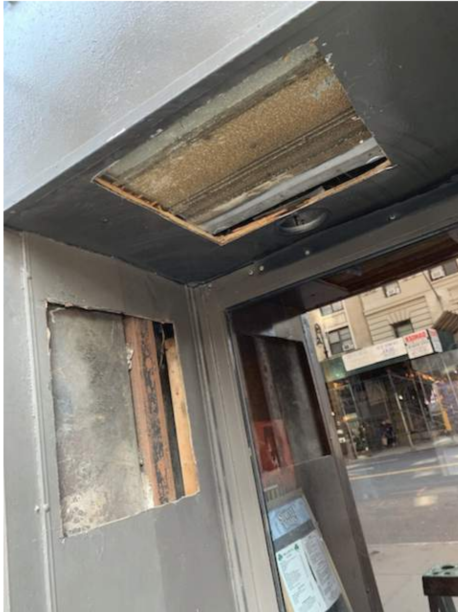
PROBE AT BAR ENTRY SOFFIT
