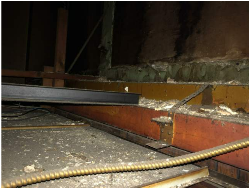
PROBE AT PLYWOOD INFILLED HISTORIC STOREFRONT
