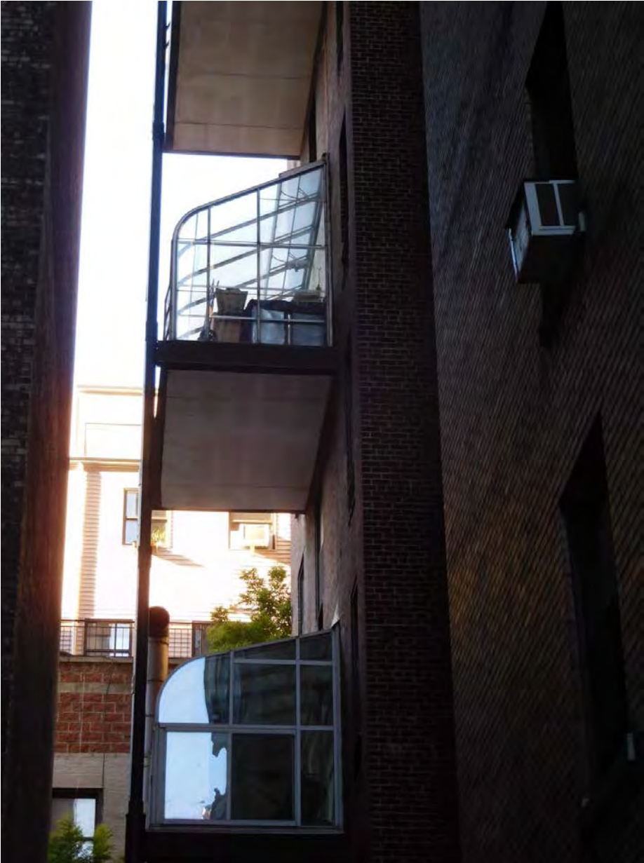
Existing Conditions 3B
