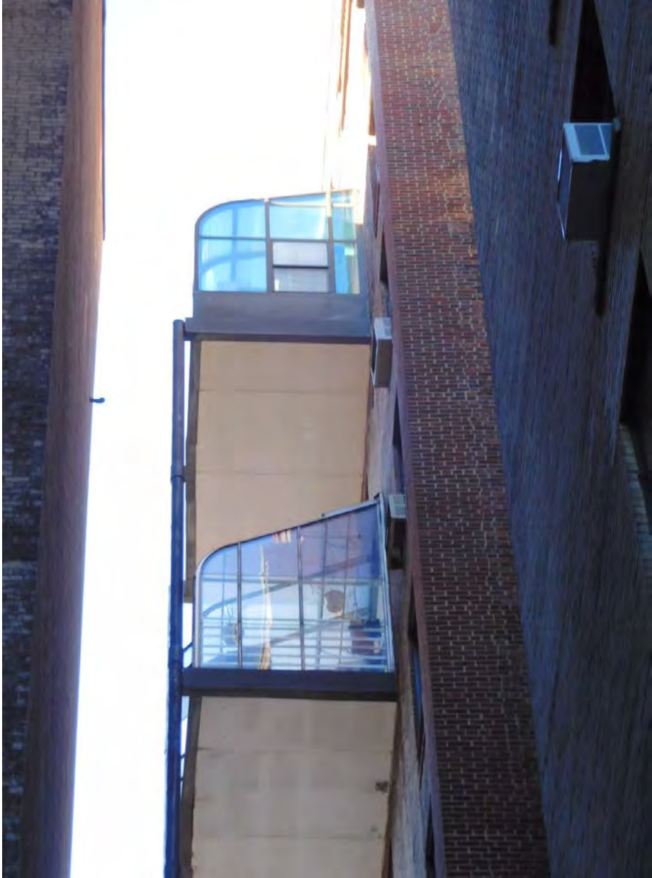
Existing Conditions 11B
