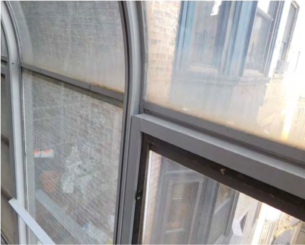
Glazing Conditions Photo #2 4970
