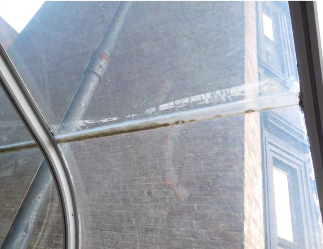
Glazing Conditions Photo #1 4969
